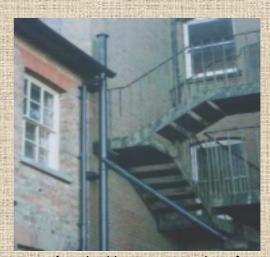
**vent pipe:** in this case vent pipes from each chamber meet to vent any smells above the gutter line.
