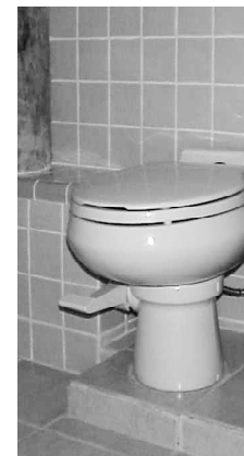
A Typical guest house (Left) at Lalatl, a eco-resort in Fiji. Each guest house features a roll-away composter (top right), a micro-flush toilet (above) and a Washwater Garden for graywater (top left). (Photos: Linda Kwasny)
