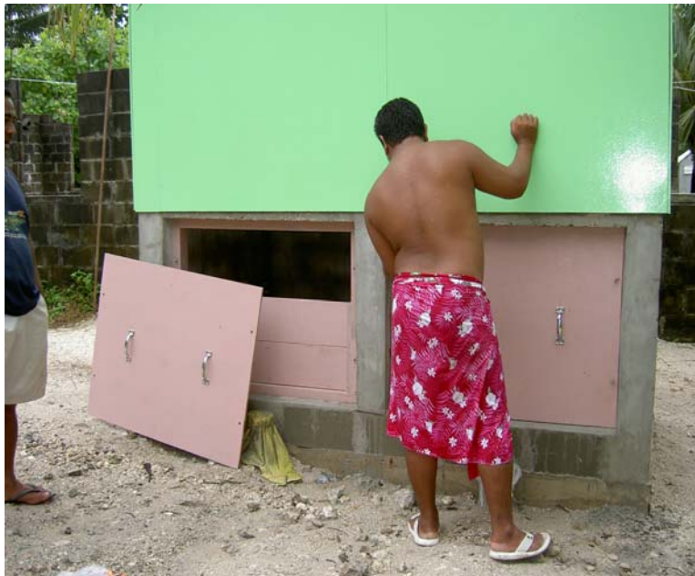
Composting chambers underneath toilet house.
