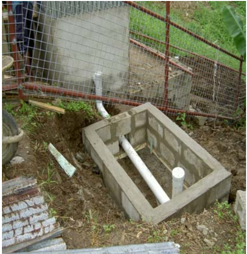
The evapo-transpiration trench, before it is covered with stones and soil.
