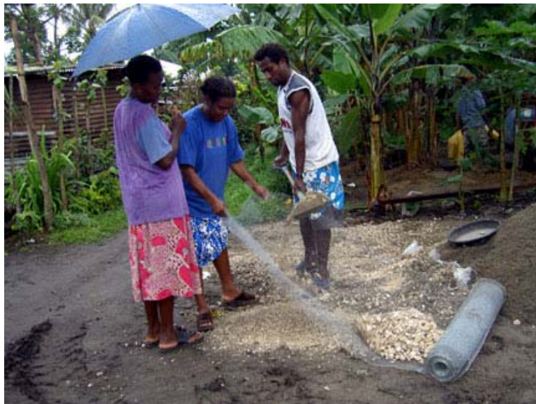
Builders in Vanuatu -making sure the stones/coral are the right size
