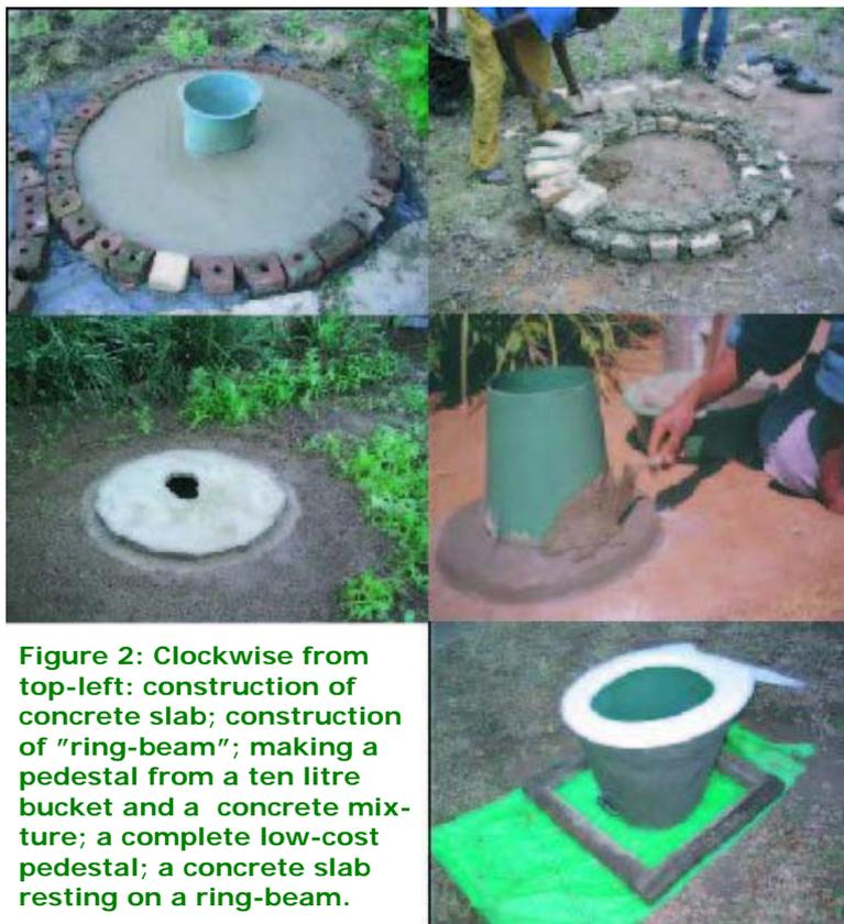
**Figure 2: Clockwise from top-left: construction of concrete slab; construction of "ring-beam"; making a pedestal from a ten litre bucket and a concrete mixture; a complete low-cost pedestal; a concrete slab resting on a ring-beam.**
