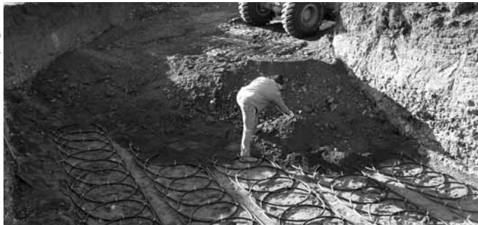
The coil for a ground-source heat pump being laid in a domestic garden
