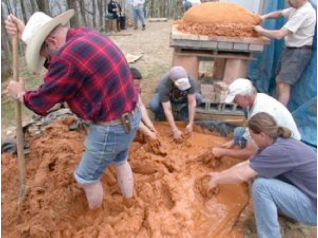
Preparing cob lumps ready for placing on the sand form.
