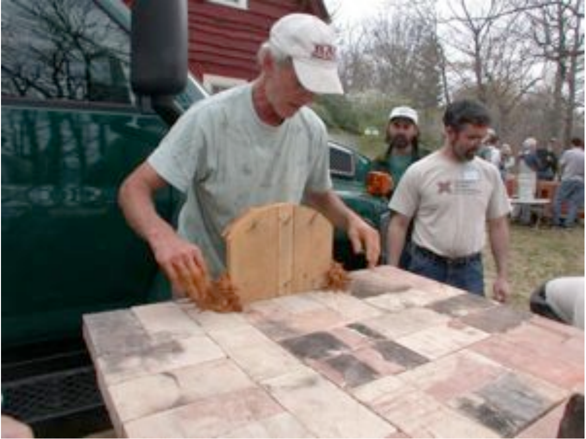
The hearth is recycled firebrick laid dry. Tom spots the door plug in place with cob.
