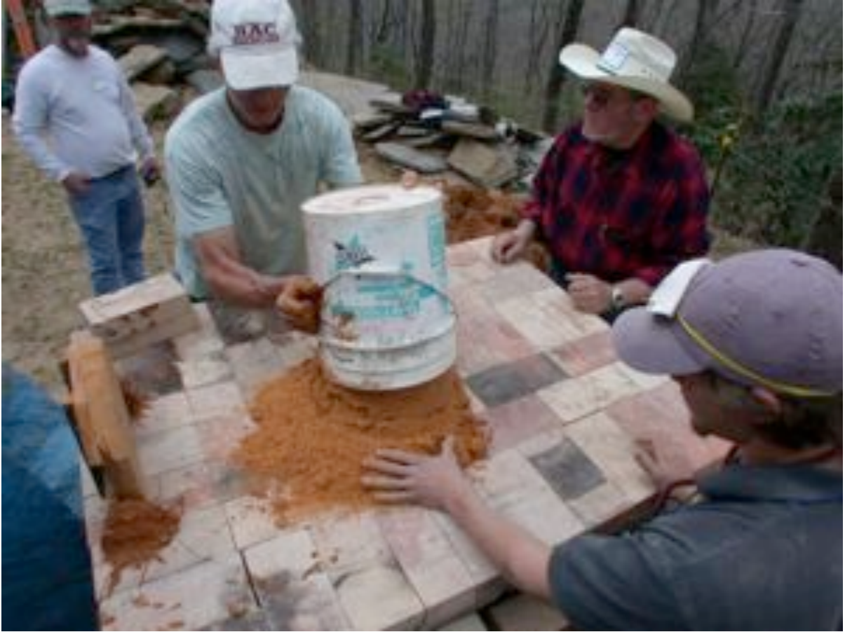
Damp sand is used to form a mold for the clay oven shape.
