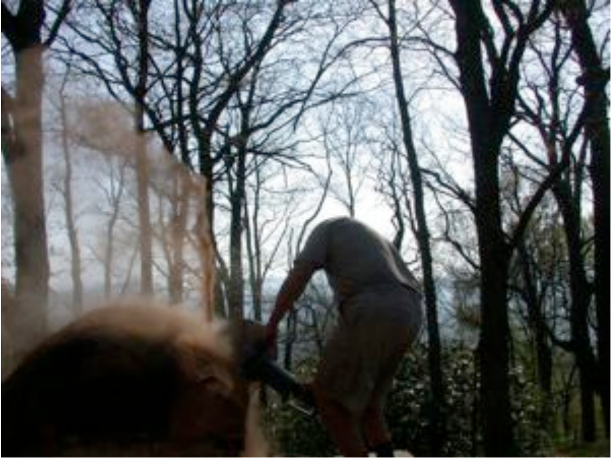
Norbert Senf slices the oven with a diamond blade.
