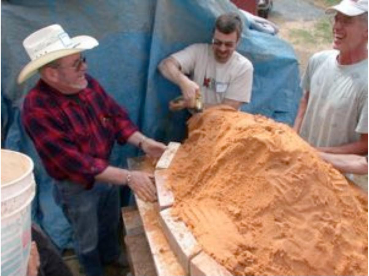
Firebricks are used to shape the edge of the sand. John Rousseau wets the sand.
