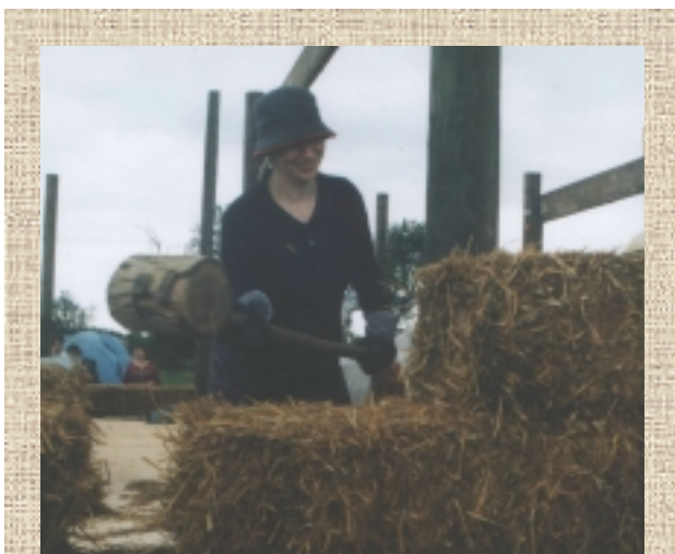
the 'persuader': another home-made tool, this time for gently persuading bales into the position you want.
