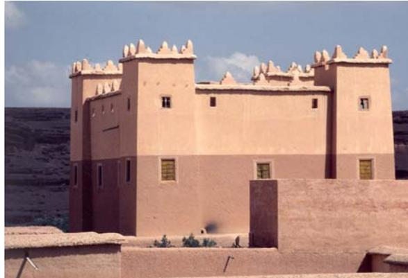
Figure 1: House with stabilised soil render in Atlas Mountains, Morocco.
