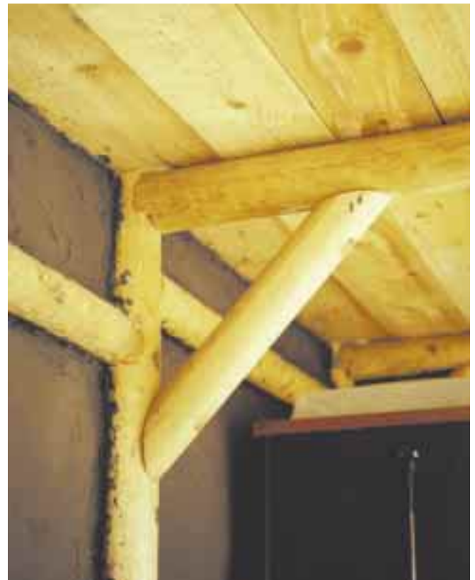
Above: Posts and beams still spotted with stucco.
