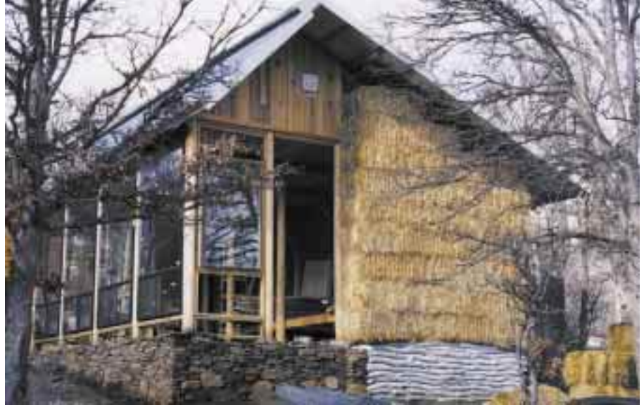
Above: The east end shows dirt bag, stone, and straw bale techniques.
