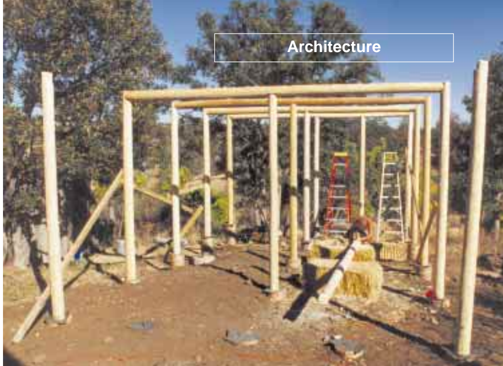
Above: Working our way up, post and beam on concrete piers.
