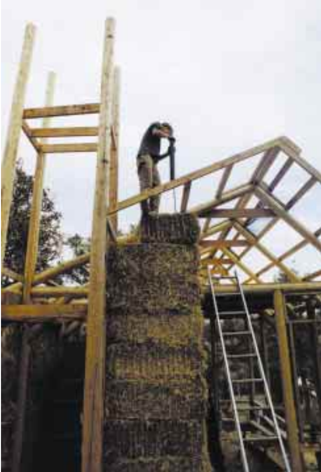
Above: Driving the rebar which pins bales together.
