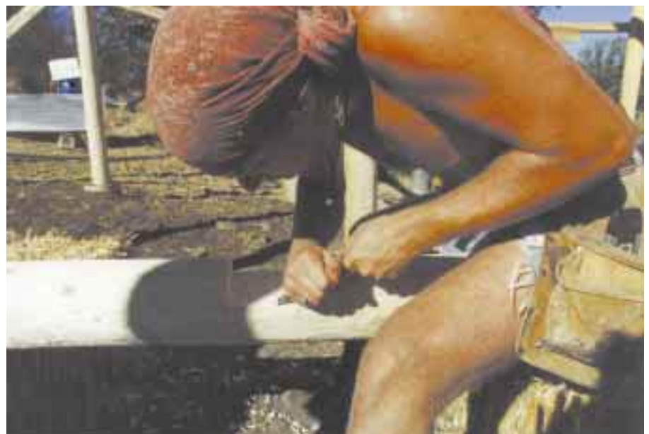
Below: Ben cleans up a notch in a beam.
