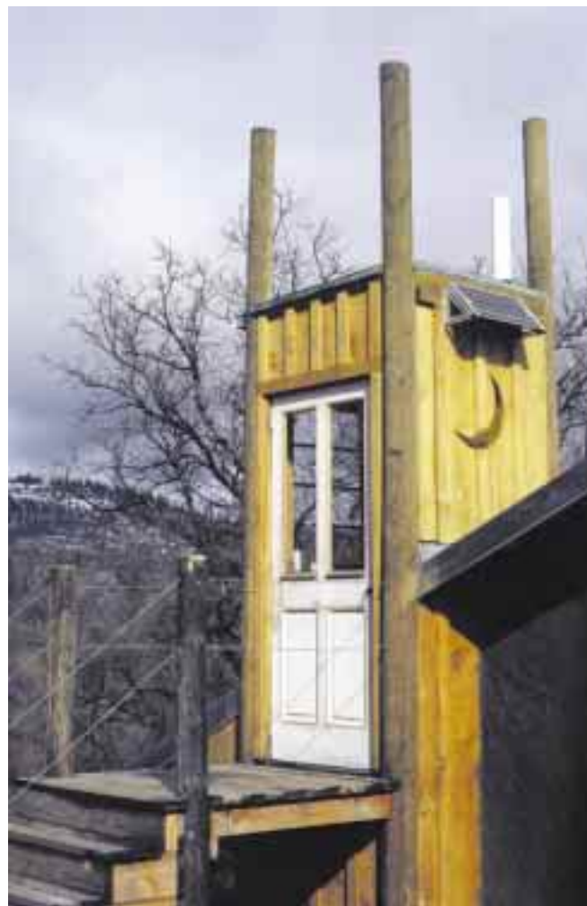
Above: The Turd Tower with obligatory moon window. The small PV powers the toilet's vent fan.
