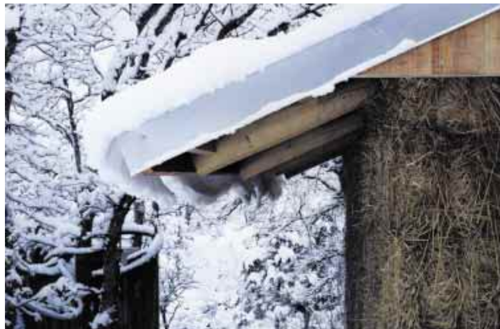
Below: large roof overhangs kept bare bales dry over the winter.
