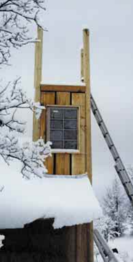
Above: The tower from the North. No access yet.
