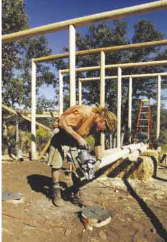
Above: Joe notches beams.
