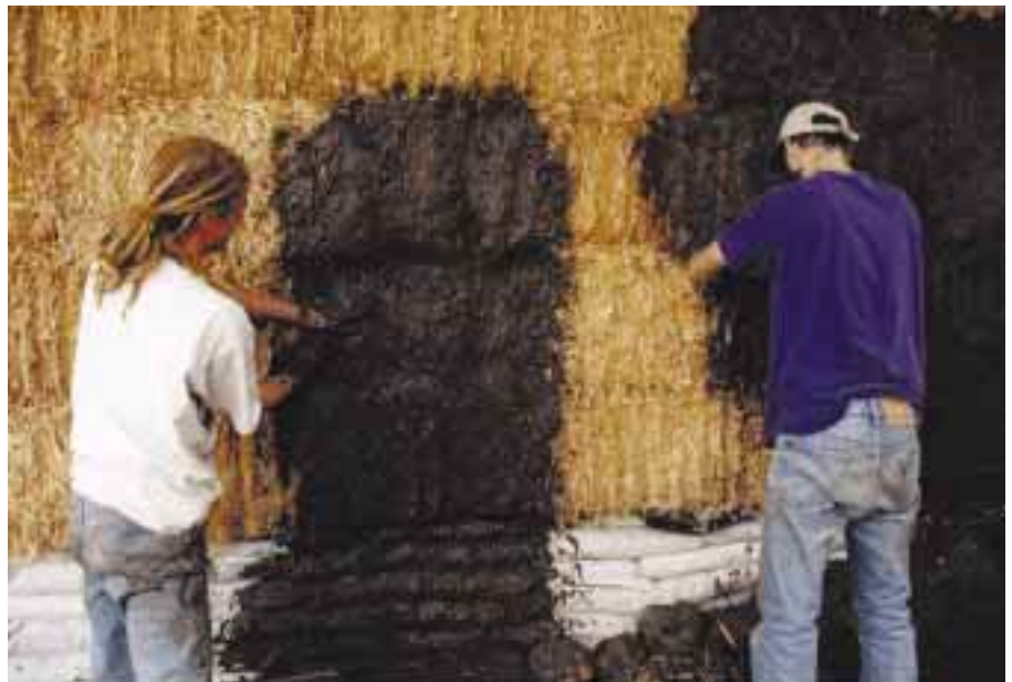
Below: Joe and Doug spread the first thin layer of stucco.
