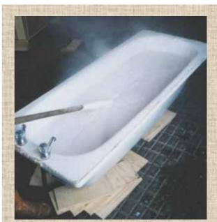
quicklime being slaked in an old bath: the lime must be added to the water and not the other way round, as it could cause an explosion. The ratio of water:lime is 3:1. To ensure that all the lime is slaked, the mixture is raked continuously for 10 minutes. There is a violent reaction, and heat and steam is given off. When it is cool, the 'lime putty' can be stored in plastic buckets indefinitely as long as there is a layer of water on top.
