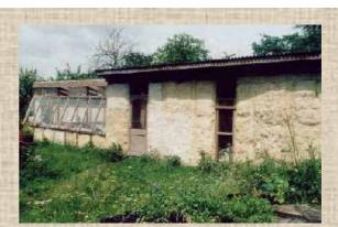
straw-bale building with lime render: 1 part lime putty is mixed with 3 parts sharp sand. The walls are sprayed with water first; apply two coats, and allow each to dry slowly by covering with wet sacking.
