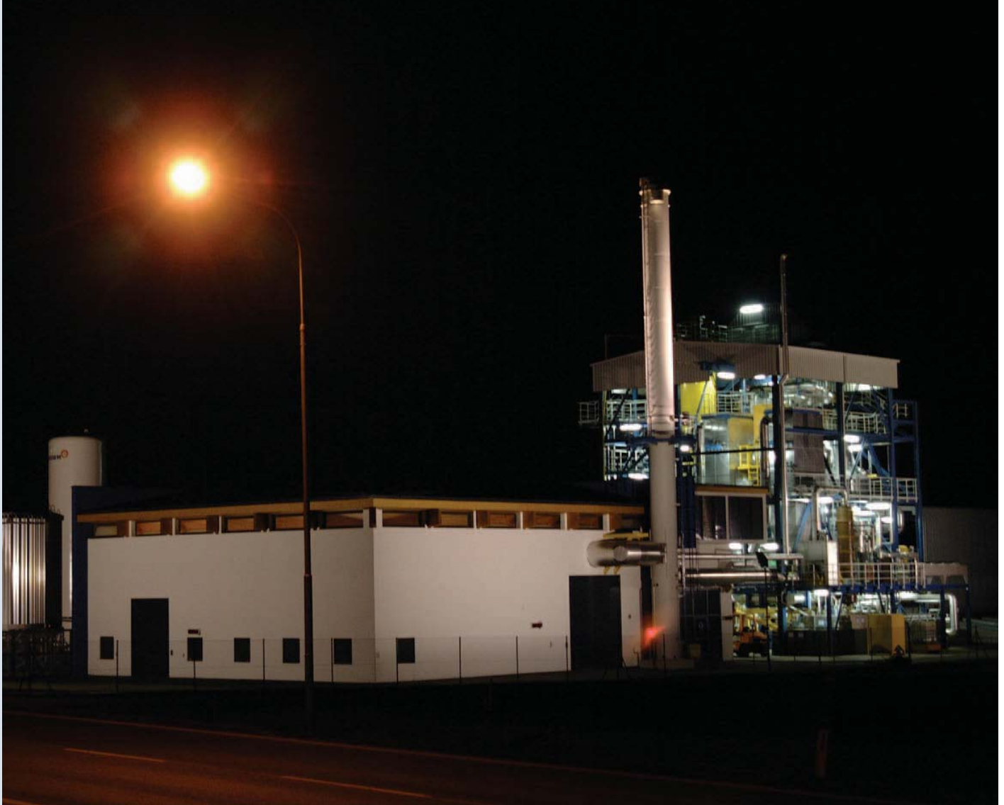
The Güssing gasification plant (above) has two connected fluidised bed chambers, one for the gasification itself, the other for combustion. Because steam rather than air is used in the gasification chamber, which operates at around 850°, the biomass is turned into a gas with very little tar, with a high heat value because it is not diluted with nitrogen as it would have been if air had been used. The main components of the gas are hydrogen, carbon monoxide and methane
