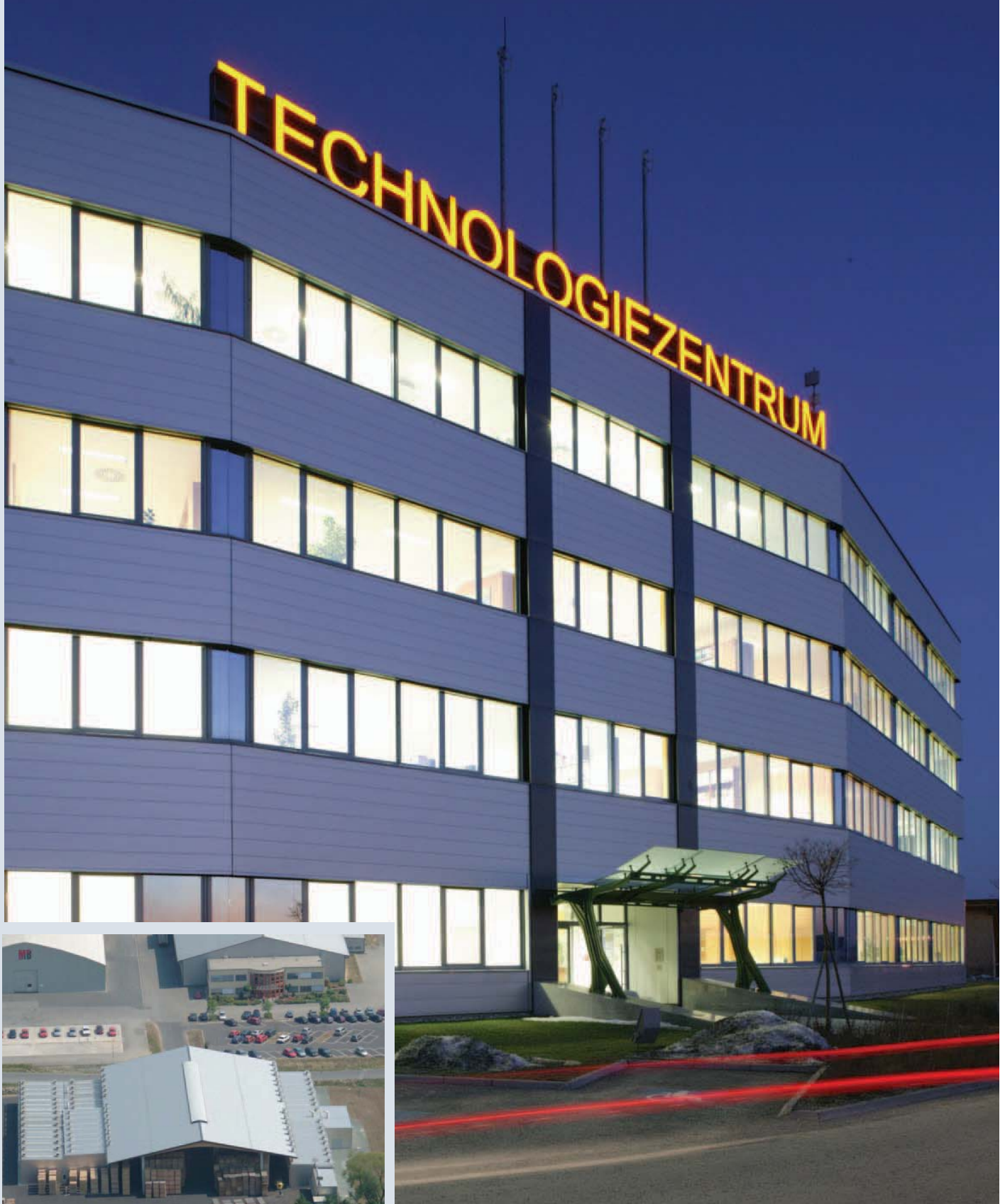
Because of the availability of cheap heat, over 1,000 jobs have been created in and around Güssing, including 100 in a new office building on an industrial estate which houses EEE, the European Centre for Renewable Energy (above); just outside the EEE office block are the yards occupied by two manufacturers of parquet flooring (inset), who use the heat to kiln-dry their timber, which mostly comes from the local woods, before processing it
