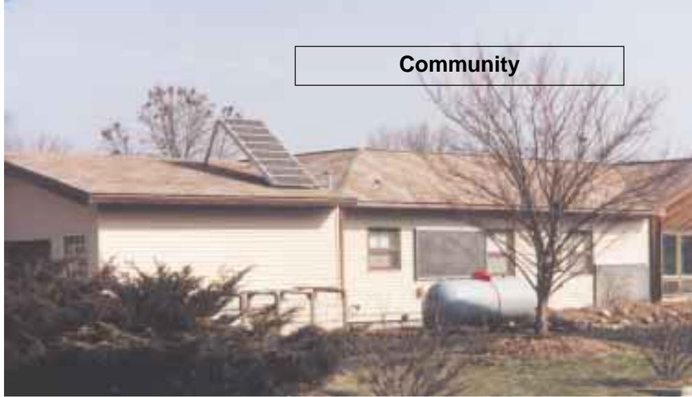
**Russ Hardtke has eight Arco Solar 16-2000 PVs and solar hot air collectors.**
