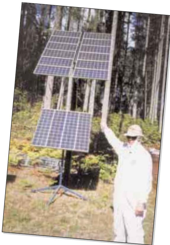
This system consists of approximately 800 peak watts of PV on a fixed pole mount. Eight Trojan L-16 batteries connected in series/parallel yield a storage capacity of 700 AH at 24 VDC. Battery charge is regulated by a Heliotrope CC-120 charge controller in the event of utility failure. A Trace SW4024 inverter is used to supply dedicated circuits in both the house and garage. AC inputs to the SW4024 consist of both a 30 amp utility source and a small 3 KW diesel generator.
