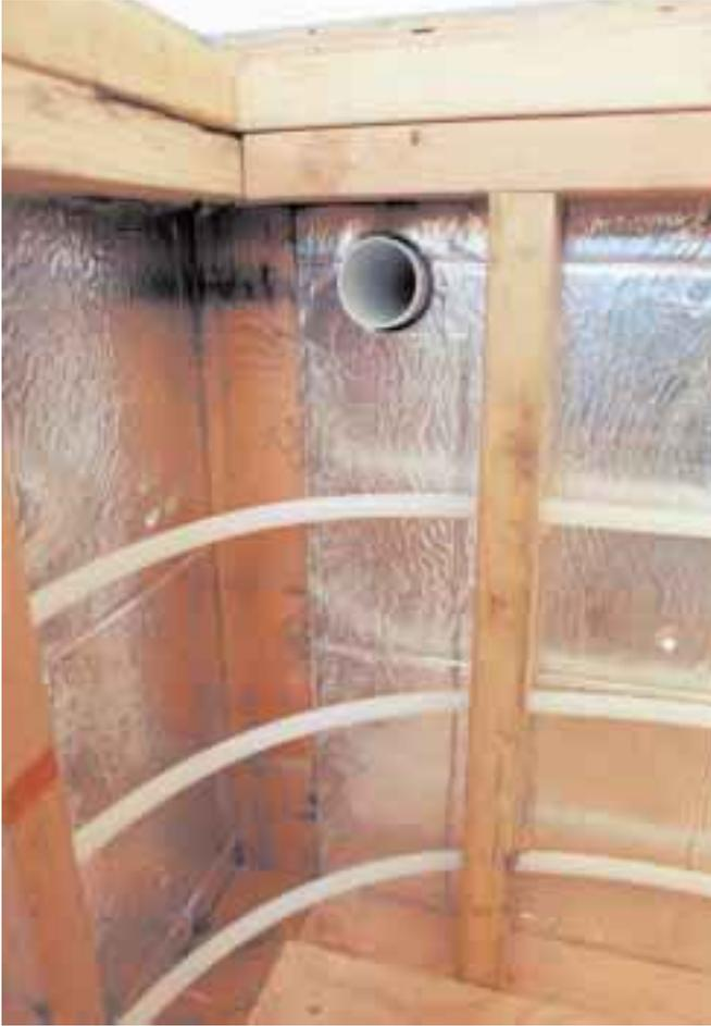
**1/2 inch PEX tubing carries the hot water through the battery space. Intake for the Power Vent is visible above.**
