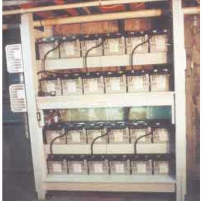
**Twenty-four Concorde SunXtender sealed absorbed glass mat batteries provide 1,800 amp-hours at 48 VDC.**
