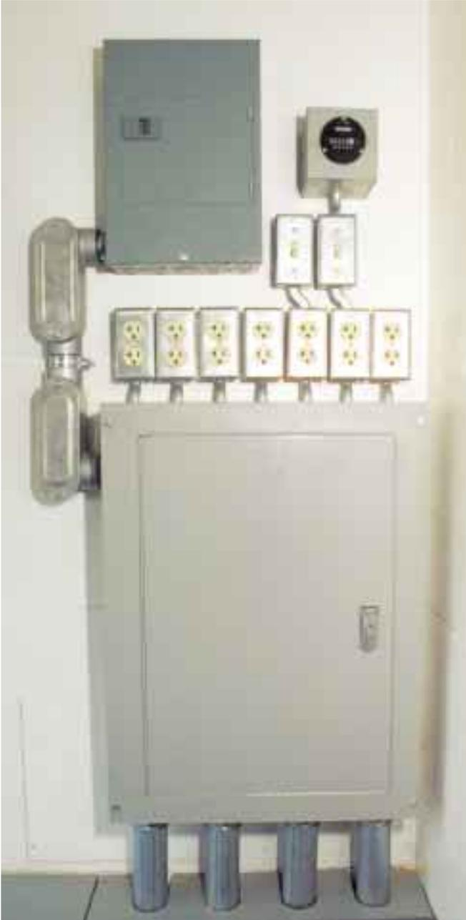
**The AC distribution center provides test plugs for seven possible 120 VAC power sources.**
