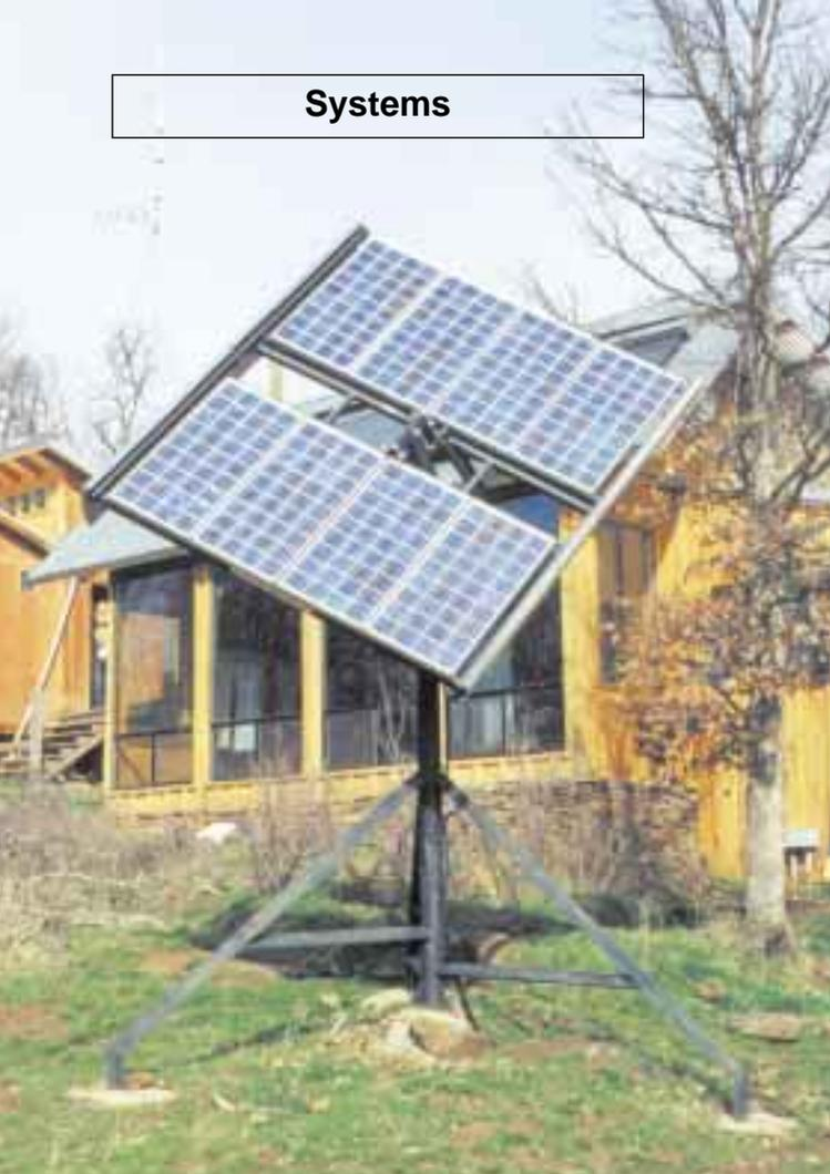
**Sub-array #2: Eight Kyocera J51 PV panels on a Zomeworks tracker provide 408 watts rated.**
