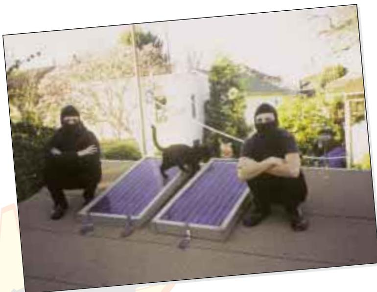
Closer to the inspector's headquarters than most, this guerrilla solar-electric system is located in the heart of one of the largest metropolitan areas in the U.S. It consists of two 60 watt Solarex panels wired in series to a 100 watt Trace Microsine intertie inverter, converting the DC electricity to AC.
