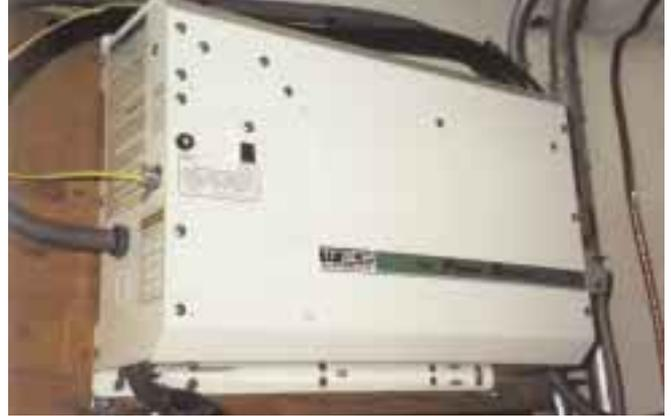
**The Trace inverter draws 5 watts when in search mode, and about 12 watts when operating.**
