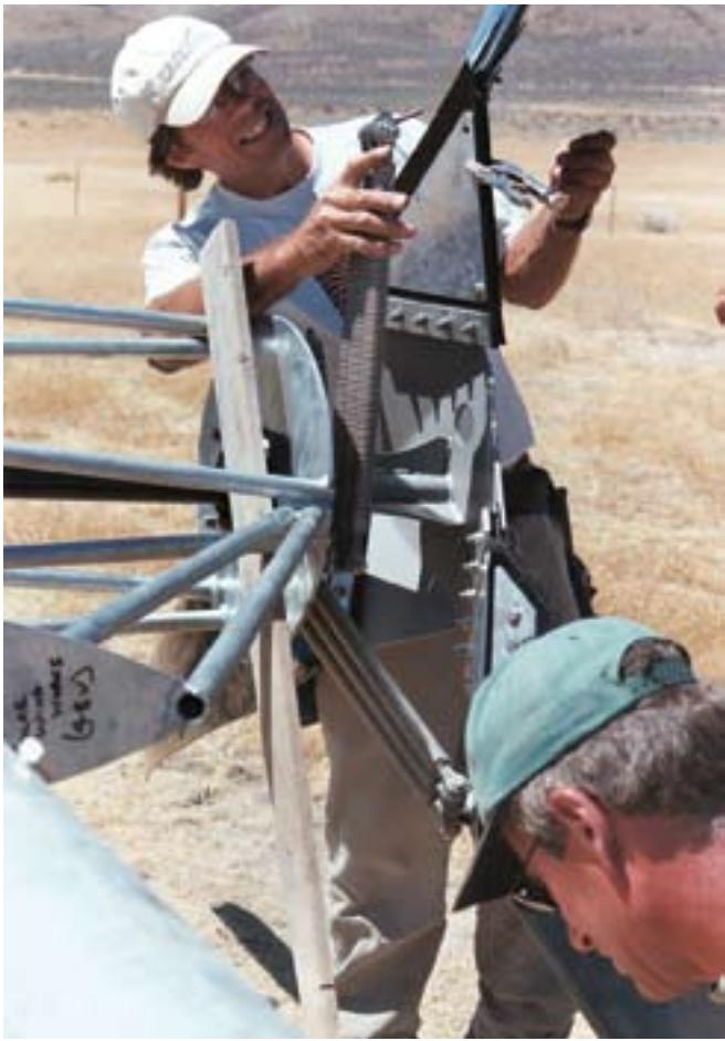
**Chris attaches a spring pack, which tensions the blade, allowing it to bend back for high-wind governing.**
