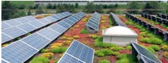
SOURCE: http://www.igra-world.com/images/Solar-Green-roof-2.jpg Greenroof Integrated with Solar Panels
