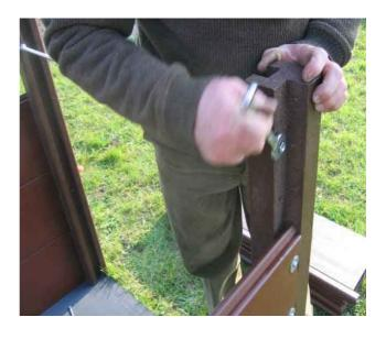
The back panel planks can now be screwed in – remember the washers, to the predrilled holes.
