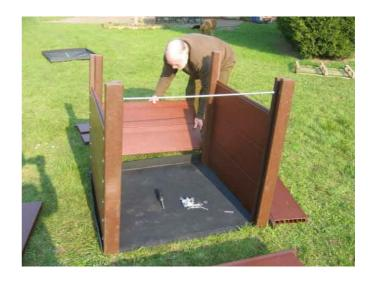
The rubber mallet is used to snap the tongue and grooved planks together as you attach them.
