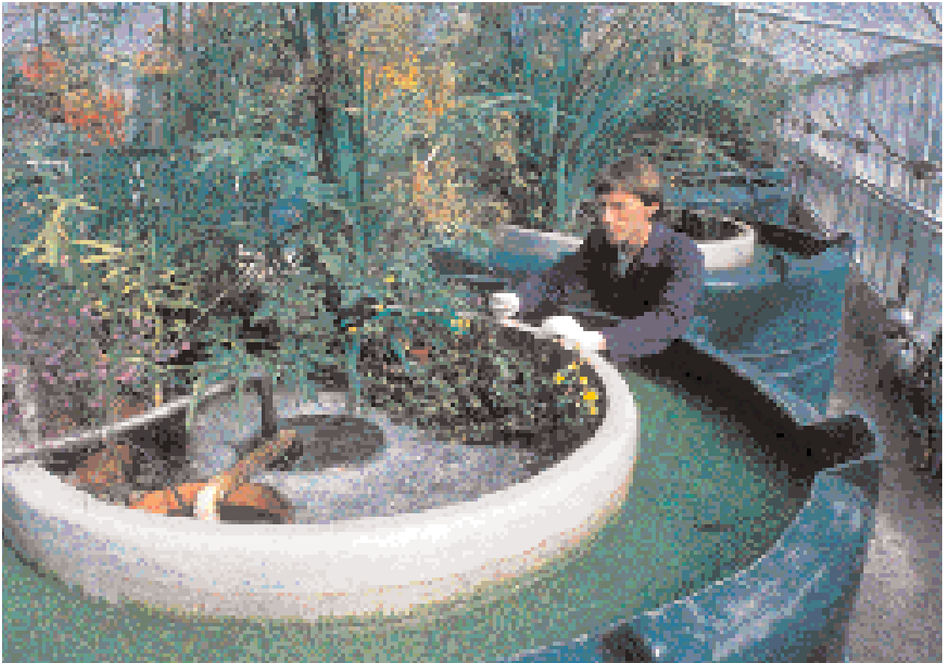
A Living Machine at Findhorn ecovillage, which cleans the community's waste water
