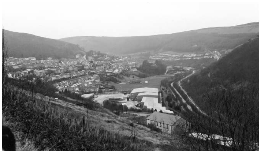
Photo 3.1: A view up the Rhondda Fach valley from Ferndale showing typical strip housing and demonstrating the constraints on industrial expansion at ground level
