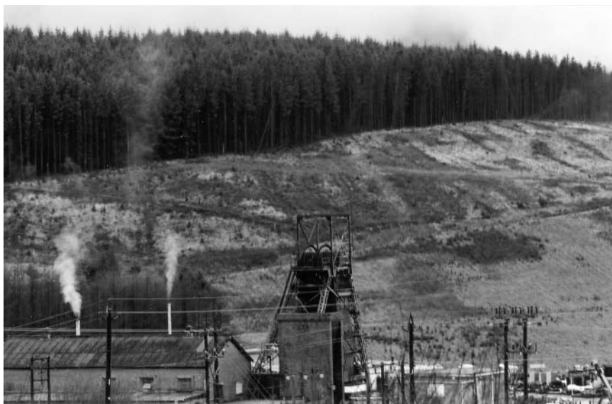
Photo 7.1: The winding gear at Tower Colliery, at the top of the Cynon Valley
