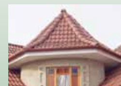
Plastic roof tiles made from recycled materials in Ukraine.
