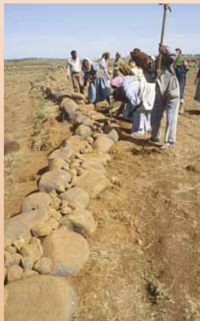
Villagers in Ethiopia using stones to create terraces, a technique to prevent soil erosion.
