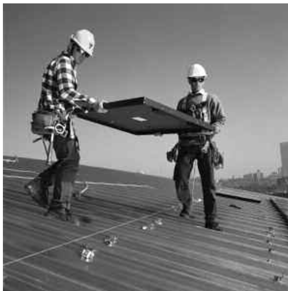
Installing solar panels on a roof in Atlanta, Georgia
