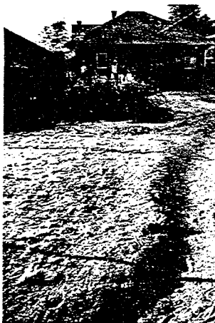
An earth water-harvesting swale, completed with the help of a bunyip.
