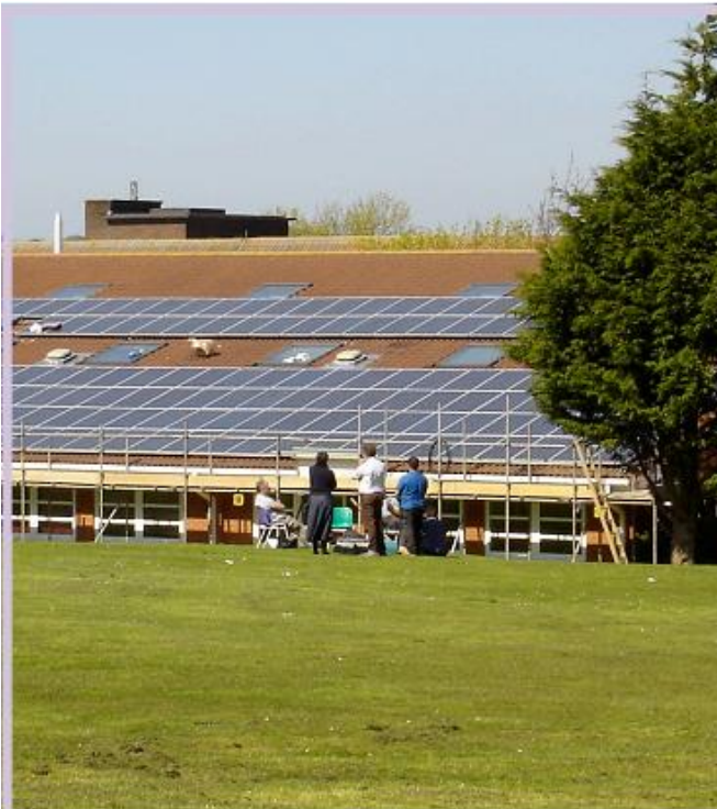
Installation of 100kWp of solar PV panels on the Matthew Arnold secondary school in West Oxford. Courtesy of David Hammond
