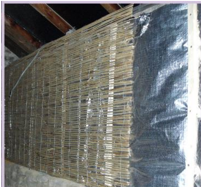
Multifoil insulation installed behind a reed mat to be lime plastered later as part of Hook Norton Low Carbon's energy efficiency improvements to Hare Cottage and Barn. Courtesy of Hook Norton Low Carbon
