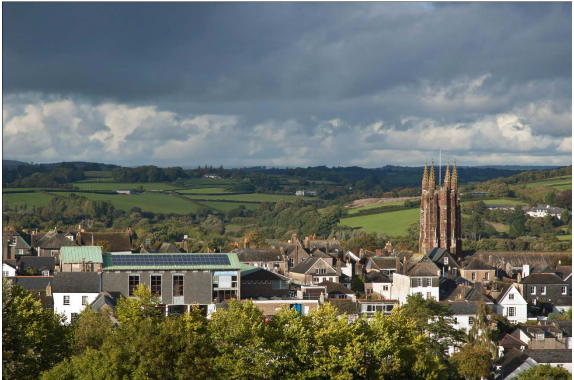
Figure 7.6. Panorama of Totnes town showing the Civic Hall with its new photovoltaic roof installed as part of the Transition Streets initiative (Source: Lou Brown/Transition Streets).
