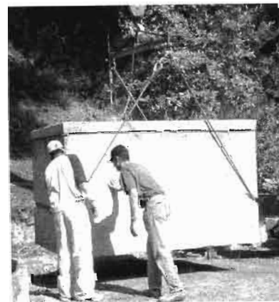
A 1,000 gal (3.8 m 3 ) pre-cast concrete septic tank.
