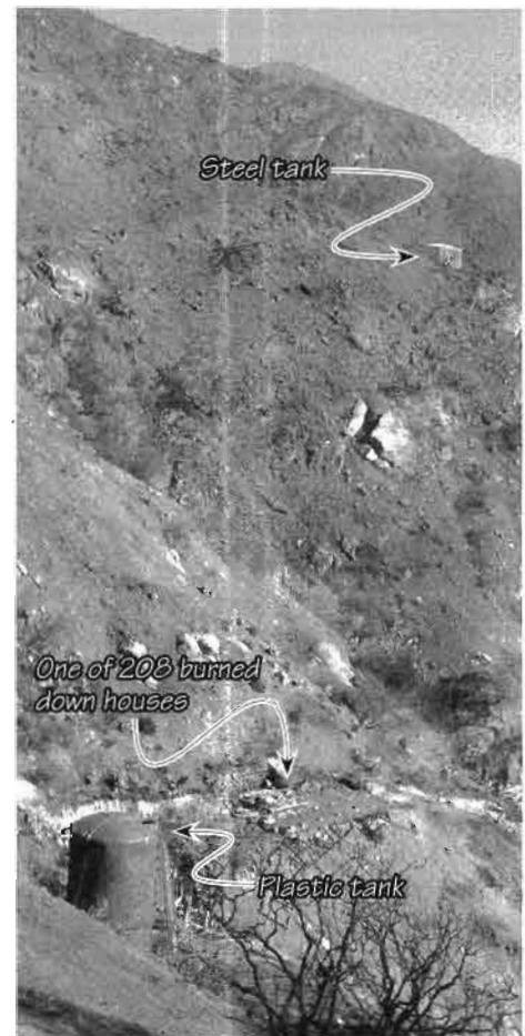
Almost all water tanks survived the 2008 Tea Fire in Santa Barbara, CA, somewhat worse for the wear, but still watertight. Several ferrocement tanks did well.
