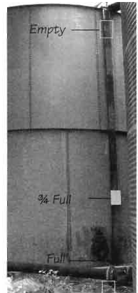
Bought float-type level indicator.
