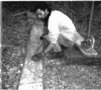
7. Bending the rebar verticals.
