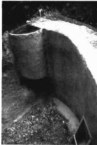
A 12,000 gal (44 m 3 ) mortar and rock diversion at the base of a waterfall in Mexico.
