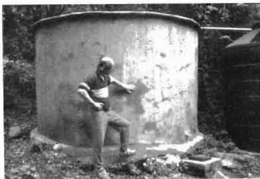
Here a 20 year old, ultra-light-duty ferrocement tank gets a re-plastering in an effort to slow its disintegration, with mixed results.
