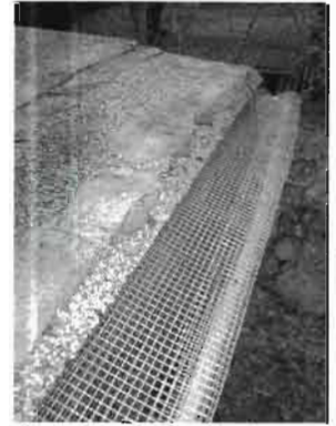
Quarter-inch welded wire mesh over gutters is first line of defense against rats crawling into this rainwater harvesting system. A water seal downstream stops mosquitoes.
