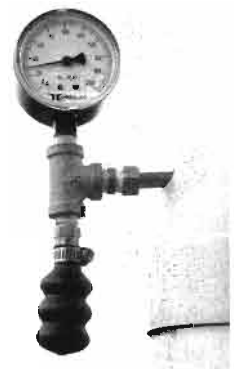
Air pressure gauge to show tank water level.
