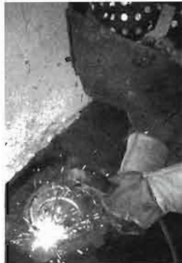
The whole assembly was then welded to the bottom of the old, assembled tank from the inside.
