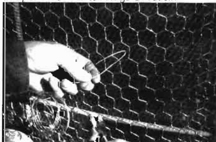
11. Tying off lath (inside) and chicken wire (outside); first make a hook on the end of the wire, push it through...
