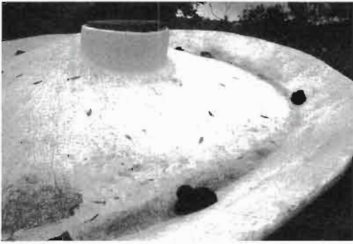
Placing the service access at the conical peak of this 13,000 gal (50 m 3 ) ferro-cement tank allows several thousand gallons more water to fit before it overflows out the access.
