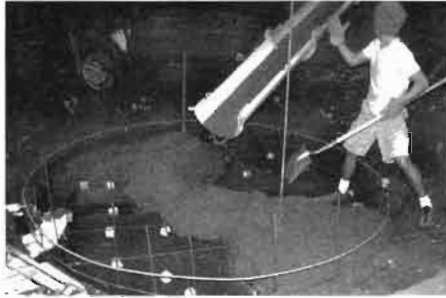
5. Pouring the floor.
