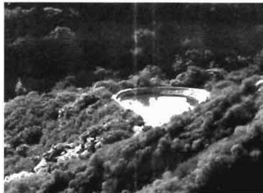
A concrete-lined storage pond excavated into the spine of a ridge above an avocado orchard. It is filled by water pumped up from a creek diversion through a few hundred feet of 4” pipe.
