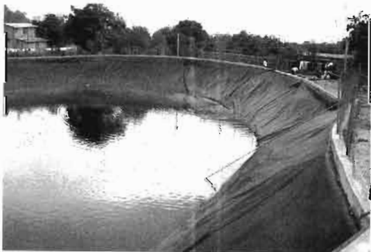
Runoff-harvesting storage pond for a village in Mexico. This EPDM-lined pond is filled through a mile (1.5 km) of 2.5” HDPE line from a seasonal creek. It fills for about four months and is used primarily for laundry during the long dry season.
