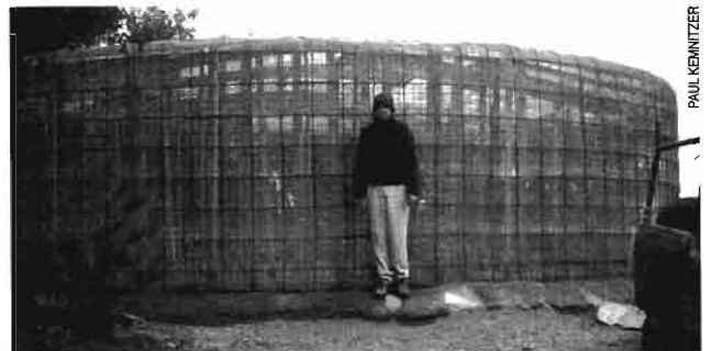
40,000 gal (150 m 3 ) ferrocement tank, ready for plaster.
