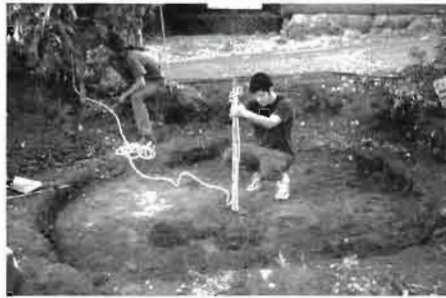
2. Grading the excavation with slope to the drain, using a water level.
