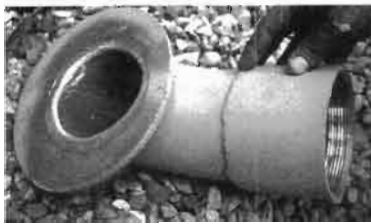
The whole assembly was then welded to the bottom of the old, assembled tank from the inside.
