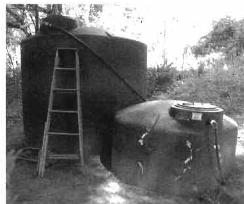
Different height HDPE water tanks. Shorter tank is for drinking water; taller tank is for all other uses. The systems aren't connected at all.
