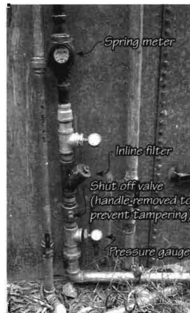
Inlet hardware. Pressure gauge before shutoff shows static pressure. Pressure gauge after shutoff shows dynamic pressure across filter, which shows when it needs service.
