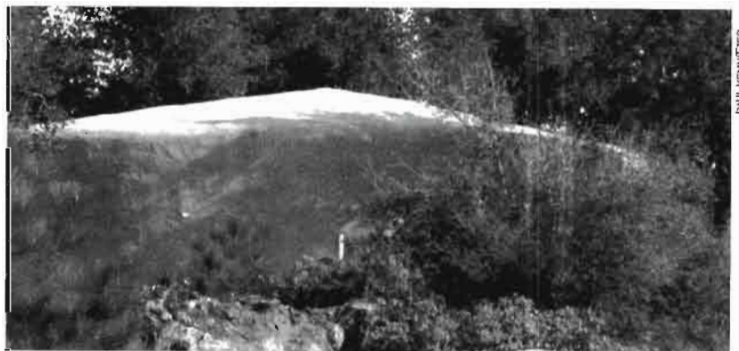
A completed 40,000 gal (150 m 3 ) tank.
