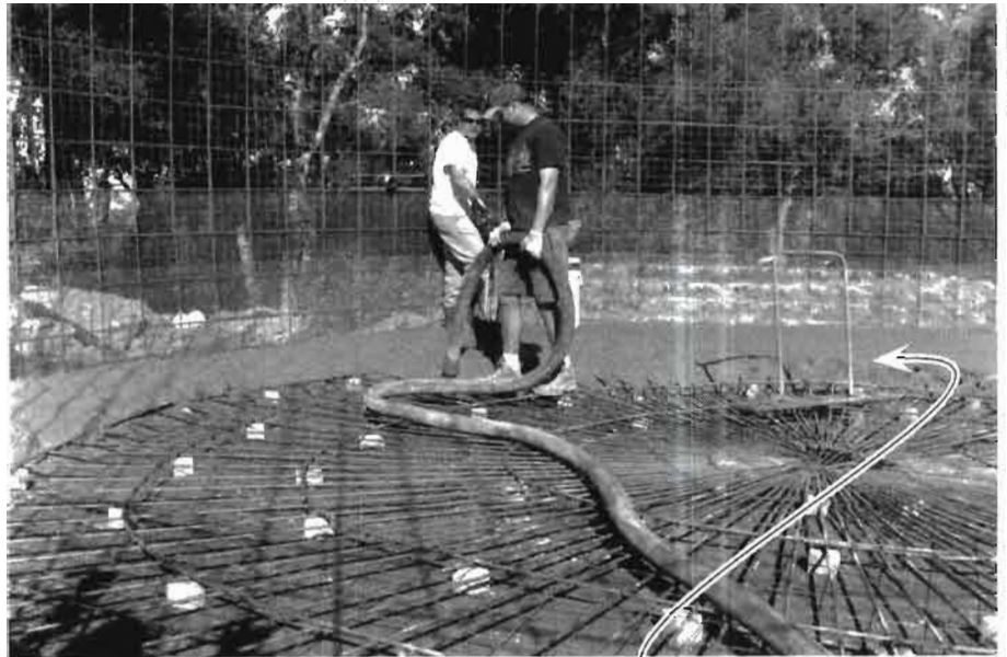
Pumping and spreading concrete for the floor.
