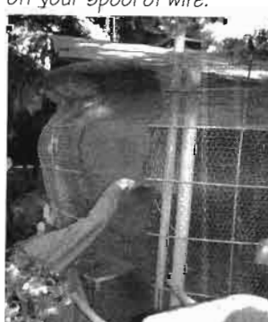
12. Then pull the hooked end back through, grab it with linesman's pliers, twist, then cut the tie off your spool of wire.
