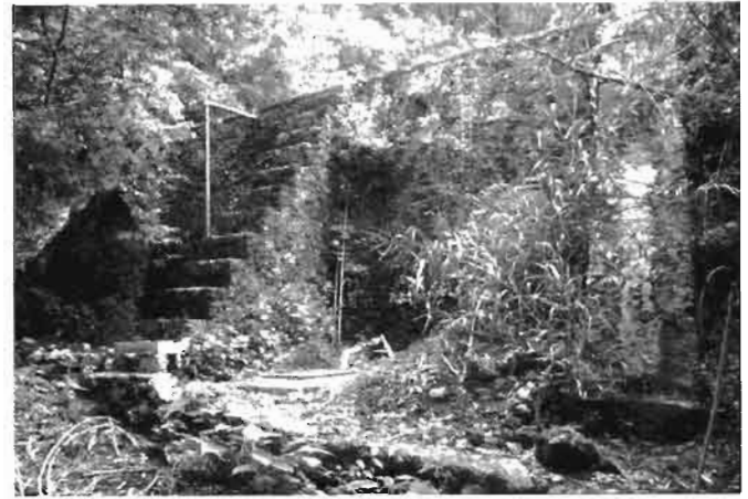
The "presa piramida" (pyramid dam)—a 100,000 gal (380 m 3 ) cistern made by sealing off the space between two walls of bedrock with stone and cement. This construction is difficult to seal perfectly leak-tight, which is important if you don't have water to add to the cistern for eight months.
