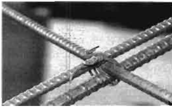
Double rebar tied.
