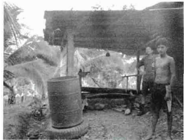
55 gal drum as roof-water catchment and storage in Panama. Much of the world lives permanently with what would be considered a state of water emergency by most readers of this book.
