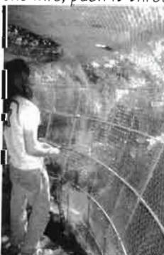
11. Tying off lath (inside) and chicken wire (outside); first make a hook on the end of the wire, push it through...
