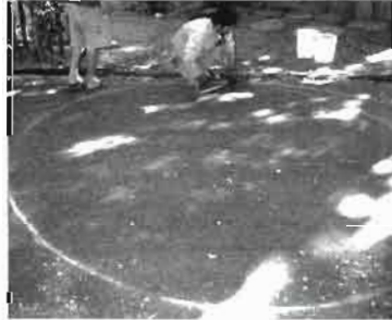
8. Circle drawn on driveway as guide for shape of horizontal rings of rebar.
