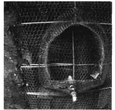
18. Altar detail over tap, formed from lath.
