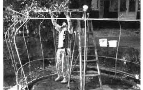
9. Placing the first rings and then verticals.
