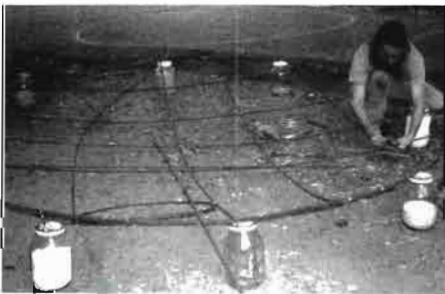
10. Bending and tying off the roof rebar.
