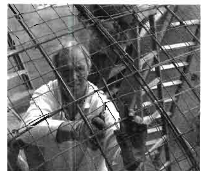
Tying off welded wire mesh with hog ring pliers.
