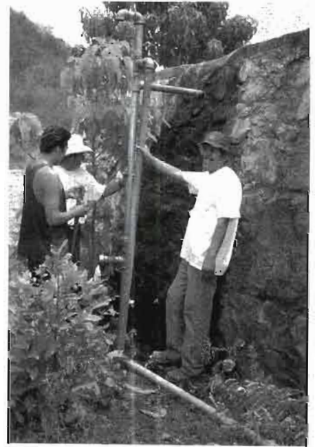
5,000 gal (20 m 3 ) leak-plagued mortared stone tank for a community water supply in Mexico.
