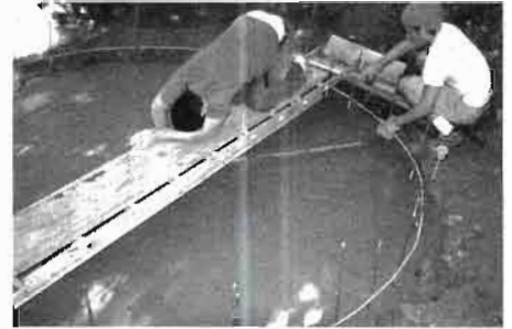
6. Leveling the floor to 2% slope and finishing.
