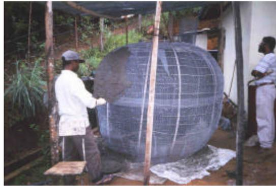
Figure 14: a) One of the 10 legs used to form the skeleton frame. b) The skeleton frame being rendered.
