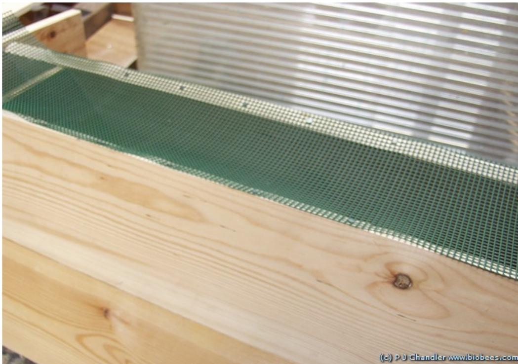
*Plastic, galvanized or stainless steel mesh may be used to cover the base of the hive. This is heavy duty plastic garden mesh, which has the advantage of forming a flexible, convex curve inside the hive, enabling the follower boards to form a bee-proof and moth-proof seal. It must be cut carefully to fit the ends and held in place with flat-headed pins or tacks.*
