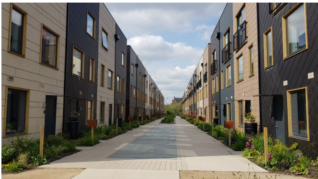
Climate Innovation District, Leeds. © Leeds Community Homes
