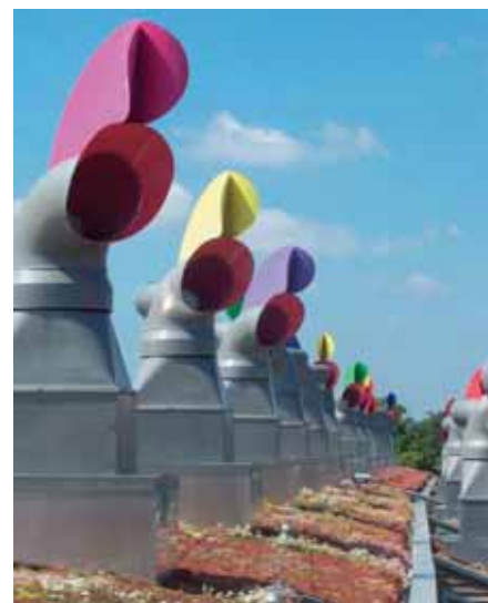
Wind cowls provide passive ventilation with heat recovery
