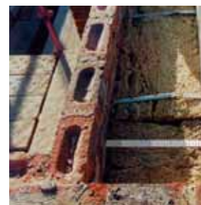
Super-insulation with wall tie
