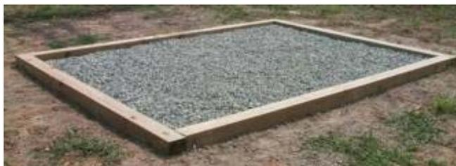
We used gravel to complete our greenhouse floor. There are many options to choose from for your greenhouse floor, but we recommend sand or small gravel because they have good drainage. In the picture to the left, there is about 2 to 3 inches of gravel in
