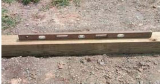
Once you have cut the wood to fit the greenhouse, lay the boards together on the ground like you are going to set the greenhouse on them (make sure you remove any rocks, sticks or dirt clogs that keep the board from laying flush on the ground). Set a level on top of one of the boards (shown in picture at left). The horizontal bubble should be in-between the 2 lines marked on the level. This should be
