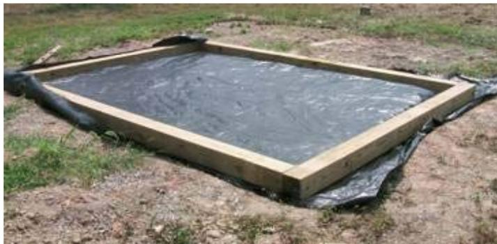
Now that the greenhouse foundation has been built, it is important to make sure your base is square. To do this, use your tape measure, and take two diagonal measurements of the base (One from the front left corner to the back right corner and the other from the front right corner to the back left corner). The base needs to
