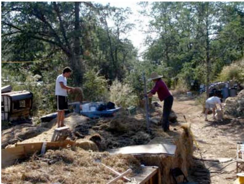
This is what the compost bins looked like. The near bin has salvaged wood sides. The far bin has straw bales sides. The deposits are covered with straw or hay each time to prevent odor and flies. They're adding the straw cover material above. The straw bale bin shown had another level of straw bales by the time it was all done. Toilet material was collected from 400-500 people over a ten day period, plus workers and staff who were there for set-up prior to the festival and after.
