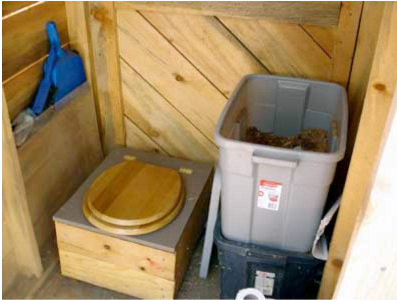
This is a closer look (above). The toilet receptacle is 5 gallons and lifts out (a white bucket). The rectangular tubs hold the sawdust cover material. It's the cover material that prevents the odor, prevents flies and prepares the human excrement for composting (urine and feces and toilet paper, even the rolls in the center of the paper).
