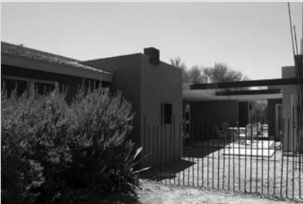
A newly formed external space provides a partially shaded seating area.
