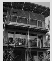
Balconies at each level provide shade to the floor below.
