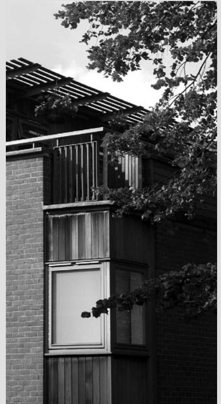
The second floor terraces of the flats provide private outdoor spaces for the tenants.
