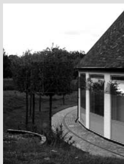
At the new BCZEB headquarters building near London (see p.248), a row of deciduous trees shades the office windows in summer and allows solar gains in winter.
