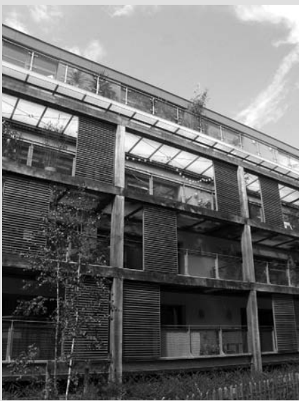
The timber balconies give character to the elevation and provide an outdoor area for the residents.
