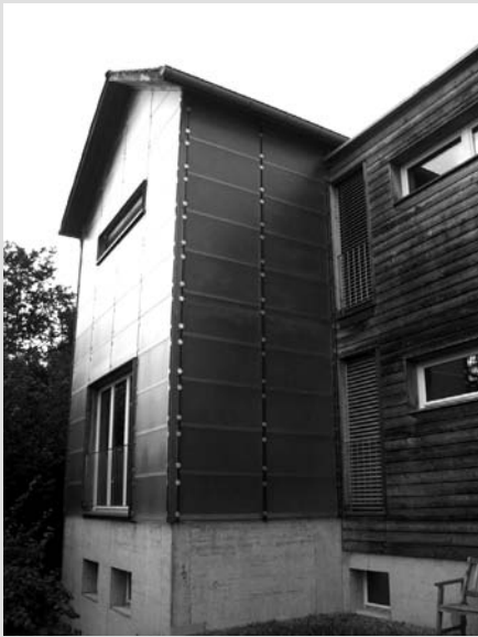
The south-facing block on the left is clad in glass, while the north-facing block is clad in larch horizontal boarding. All east-facing windows benefit from impressive views of the valley below.
