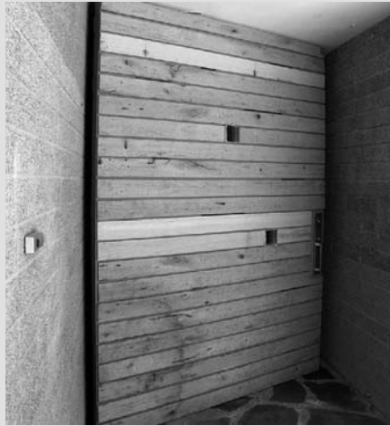
The main entrance door incorporates small glass elements and reclaimed timber.
