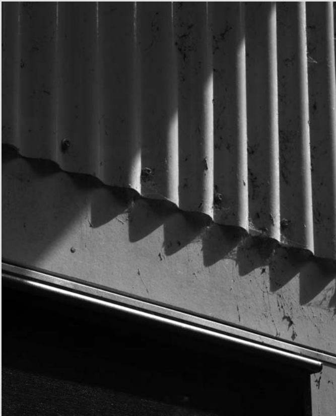
Corrugated metal cladding and timber are used to clad the pavilions
