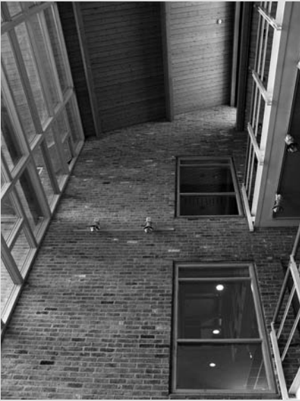
The Building Research Establishment Building 16 used 80,000 reclaimed bricks for the external walls and some internal walls.
