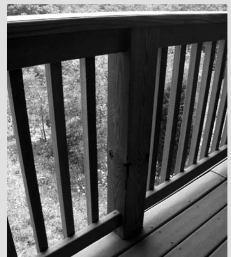
Trex post-consumer thermoplastic mixed 50/50% with recycled timber fibre used as an external decking material at the EcoVillage in Loudon County (see case study, p.140).
