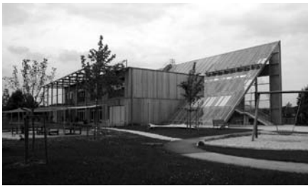
The kindergarten in the solarCity in Linz is designed to Passivhaus standards and only uses 8 kWh/m 2 yr for space heating (Architect Olivia Schimek).
