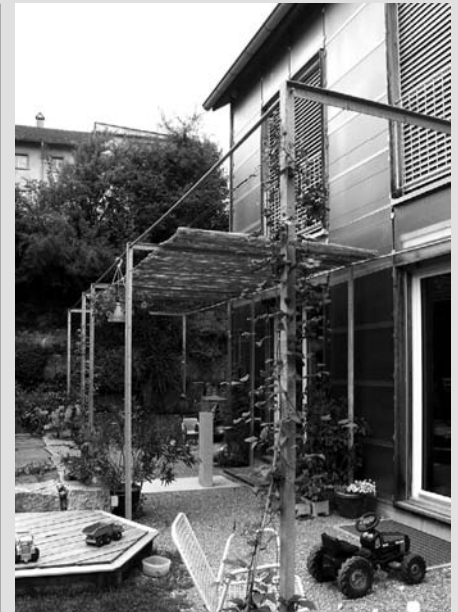
The Schreiber house is growing a planted trellis as a shading device. Until the plants are sufficiently grown a reed mat is used instead.
