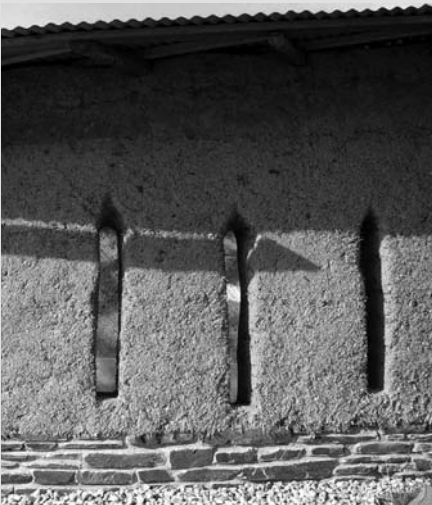
The cob sits on top of a stone base to prevent it becoming saturated with moisture.
