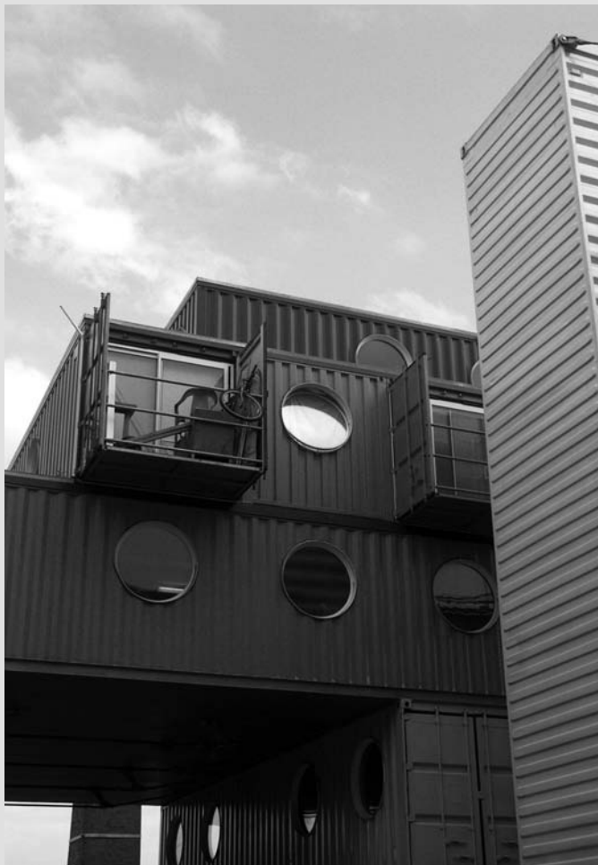
The containers overhang each other, creating a space below the units for vehicles to pass through.
