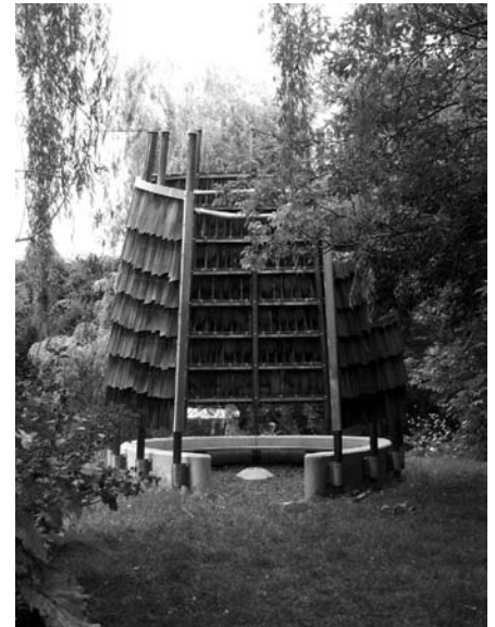
The concrete base supports timber seats around the perimeter of the pavilion (Architect Dan Hoffman).
