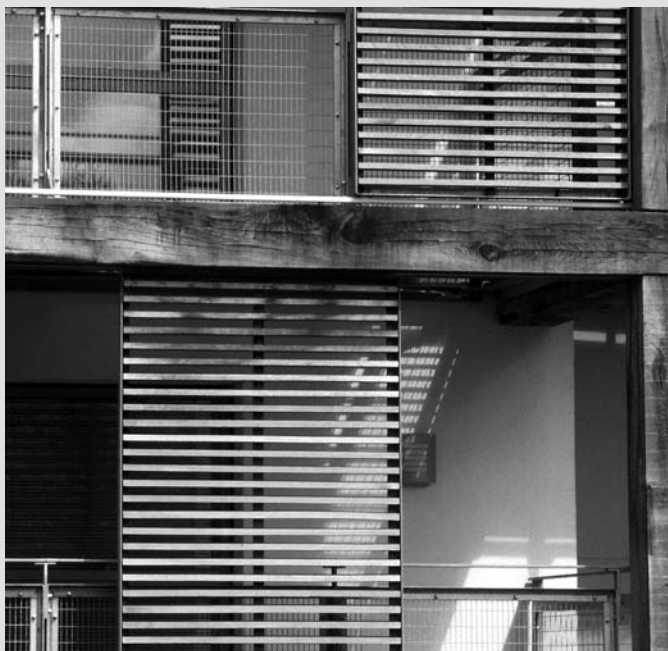
Sliding solar shading panel
