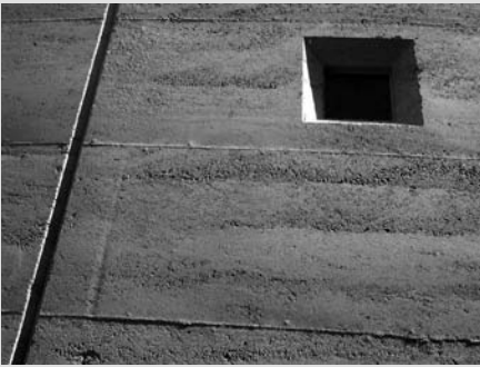
Small glazed opening in rammed earth wall.
