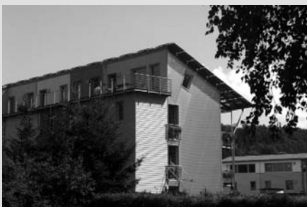
Some of the houses have monopitch roofs with PVs that face south, and a north-facing terrace.
