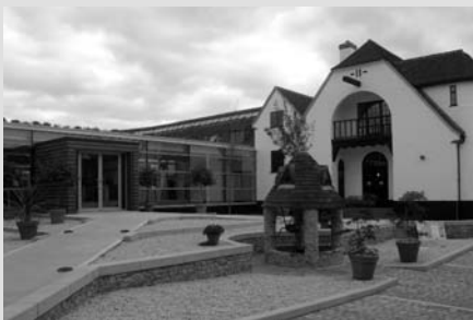
The main entrance to the offices and exhibition areas is through a single-storey glass block, linked to the existing Arts and Crafts building.
