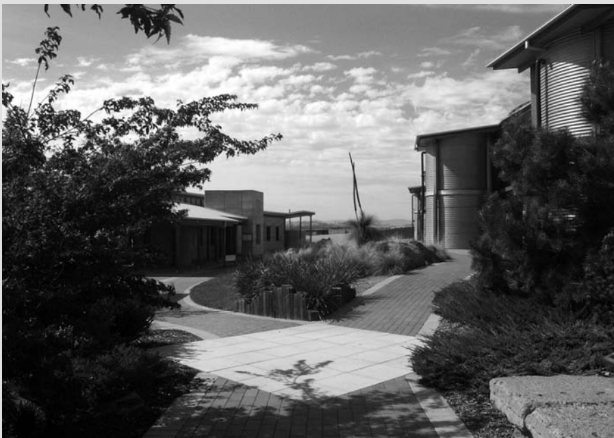
View through the planted corridor between teaching blocks. Planted areas help reduce the stormwater run-off and swales direct the water into purification wetlands.
