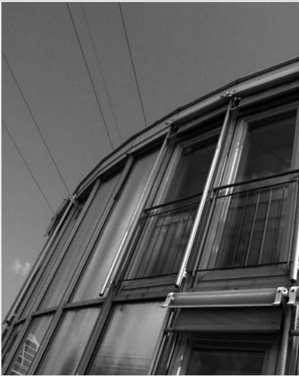
The windows have motorised, manually operated external shading.
