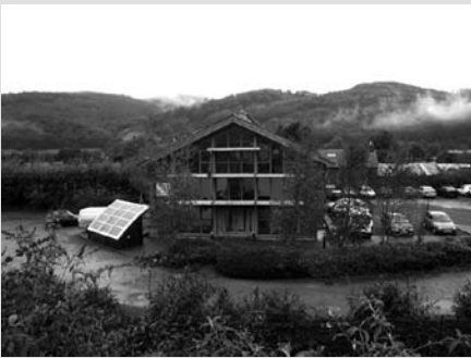
Unit One with a small PV array covering a bicycle stand.
