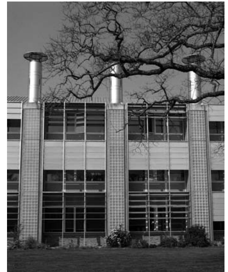
The Building Research Establishment Building 16 is a model of maximum reuse of demolition material. The building, located at the Building Research Establishment in Watford, near London, was designed by Feilden, Clegg, Bradley Architects. The existing building on the site was dismantled and 96 per cent of the materials by volume were reused or recycled: fixtures, fittings, and furniture were given to charities; roof sheeting, slate cladding and cast iron drainpipes were reclaimed; metals and timber were recycled; and masonry was downcycled. The new building (above) used reclaimed timber floors, bricks and aggregate in the structural concrete.
