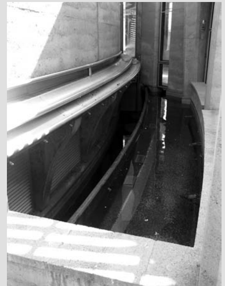
The ledge above the vents to the lecture theatre contains spray nozzles that form a screen of water, cooling the air taken into the theatre.
