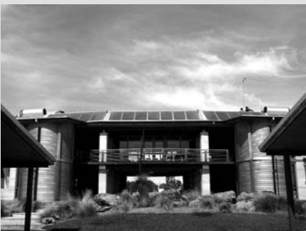
One of the teaching blocks. Two-storey rainwater tanks are located on both sides of the staff room on the first floor and an undercroft on the ground floor.
