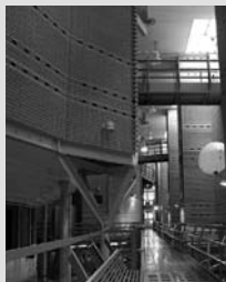
Exposed brick and concrete provide thermal mass.
