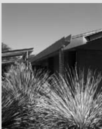
Rainwater is collected in the gutter and directed to an underground tank along the chains among the planting.
