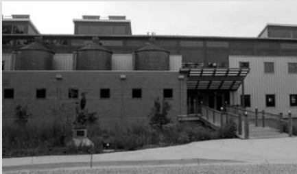
The three large rainwater tanks are located on the roof over the ground-floor offices to the left of the entrance.
