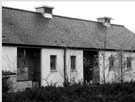
On the roof are the ventilation inlets for the houses with dynamic insulation.
