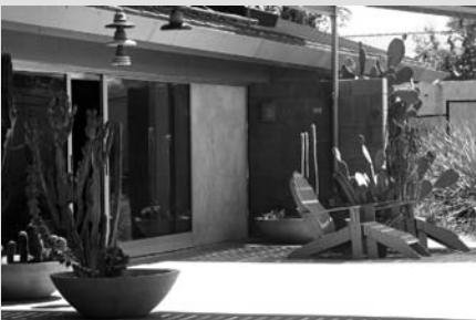
On the south elevation facing the private garden is a large glazed sliding door which links the living room with the patio.
