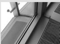
The metal ventilating elements between the external and the internal glass layer let air in and out through perforations in alternative bays. Floor level detail shows heating grill and ceiling detail shows edge of suspended ceiling.
