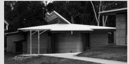
Student accommodation. Composting toilets and vent pipes are located on left side of building.
