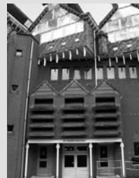
Above the doors are the air inlets for the second theatre, which has the seating facing the street.
