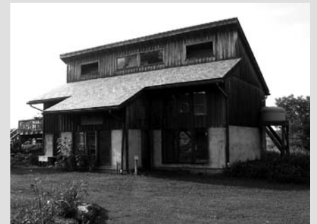
The barn collects and stores rainwater in an elevated rainwater tank.
