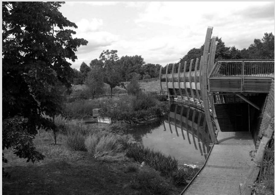
The Mile End Park art and exhibition buildings are partially located under ground and are linked thermally to the earth.
