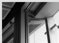
The metal ventilating elements between the external and the internal glass layer let air in and out through perforations in alternative bays. Floor level detail shows heating grill and ceiling detail shows edge of suspended ceiling.
