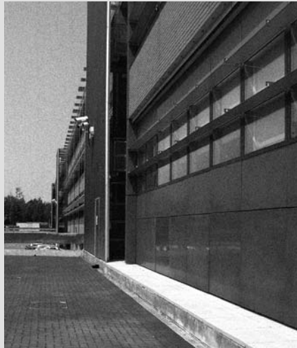
The escape stairs are clad in metal mesh and break up the over 100-metre long façade.
