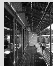
The top floor is shaded by the overhanging PV roof.
