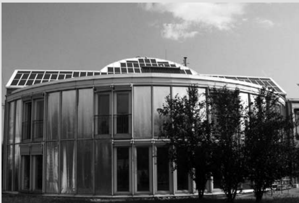
In summer the blinds shade the transparent insulated façade and roller blinds can be used to shade the windows.
