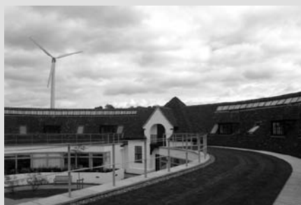
The extension to the inside of the courtyard has been covered with a green roof.
