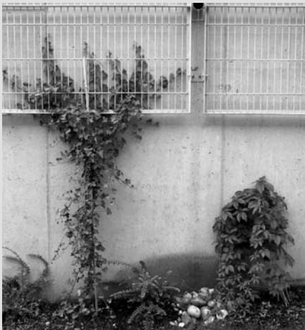
The concrete wall to the undercroft of a housing block is designed to be covered with climbers.
