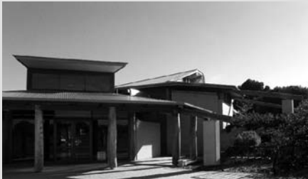
A veranda protects the entrance from the sun, while high-level windows let in light deep in the building. Rammed limestone walls and reclaimed light poles make up the structure.
