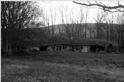
The craft workshop is nestled among the trees with the turf roof blending in with the surroundings.
