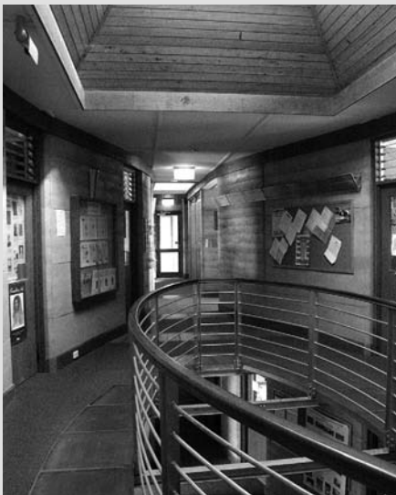
The naturally ventilated teaching block with a central vent. Note the glass louvres over the doors, which allow cross-ventilation from the office windows to the central vent.
