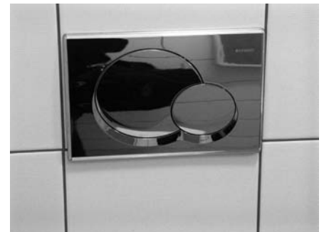
Dual flush WC flush mechanism.
