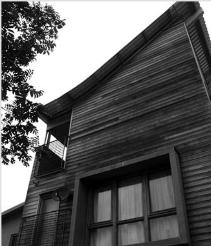
Eight flats for market rent were included in a block.
