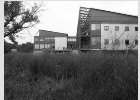
The block on the right houses the main office space and the smaller block houses the conference rooms. Each section of the building can be ventilated separately.
