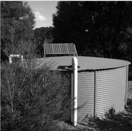
Rainwater is pumped from the main tank to header tanks by means of a solar-powered pump
