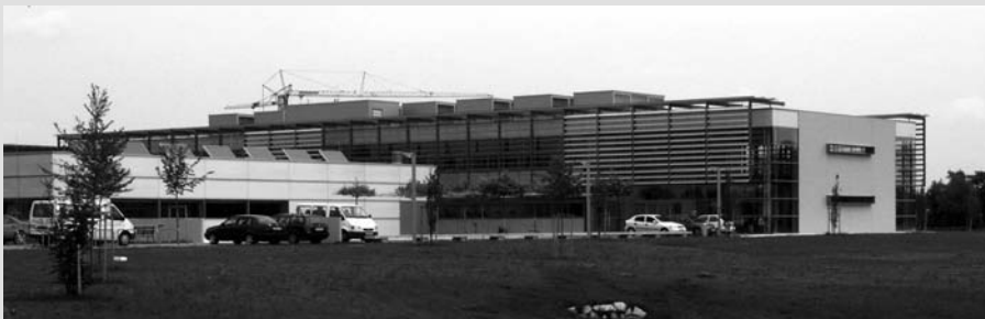
External view of school with its sun-shaded extensive glazed passive solar façade.
