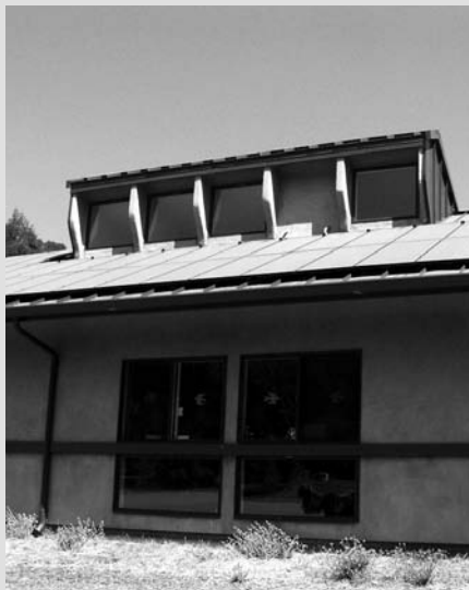
Below the windows and the horizontal strip are the water tanks providing thermal mass.
