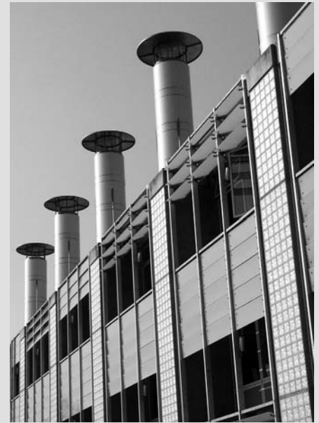
The exposed concrete soffits provide thermal mass at the Building Research Establishment Building 16, located at the Building Research Establishment in Watford, near London, designed by Feilden, Clegg, Bradley Architects.
