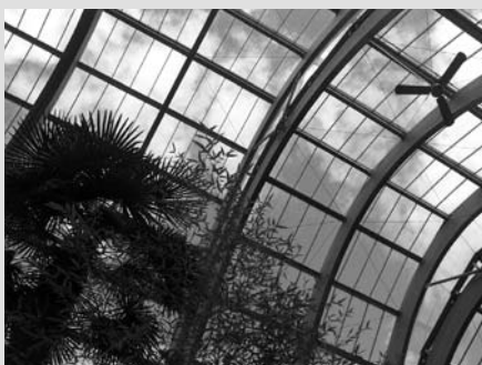
The fans induce air movement and avoid temperature stratification.
