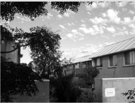
All houses have the main living accommodation and large windows on the north side to maximise solar heat gains.
