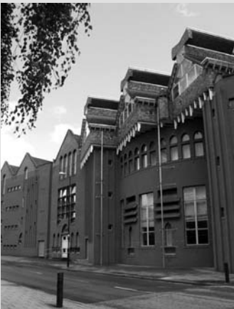
The curved external wall of the lecture theatre is visible from the street. Air inlets are located between the windows, which light the workshops below. The theatre seating has its back to the street.
