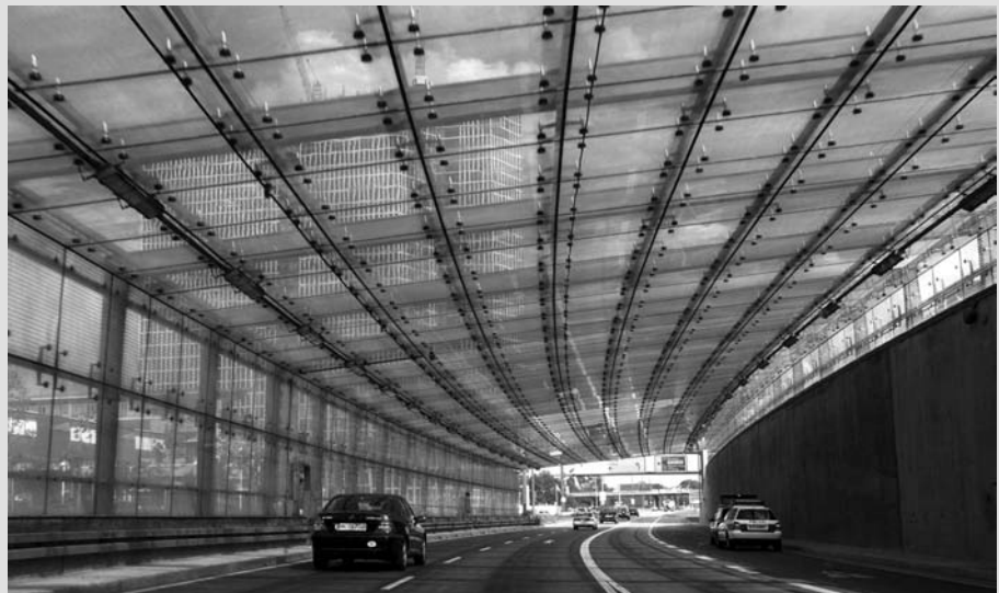
The car tunnel exit is covered with a glazed roof to protect the surrounding area from traffic noise.
