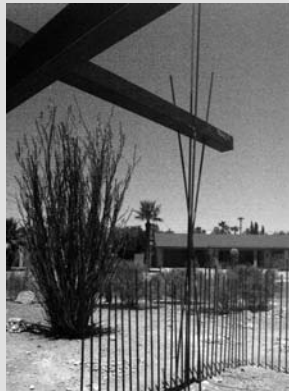
Rainwater is directed along the reclaimed rods to the ground.
