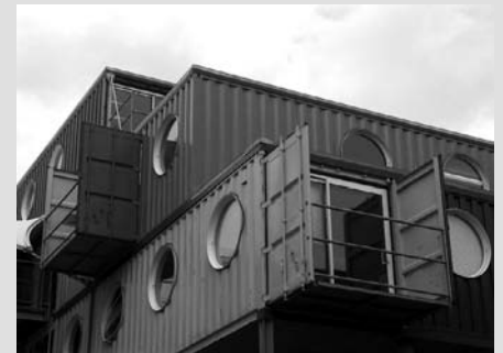
Circular windows and balconies are cut into the standard containers.
