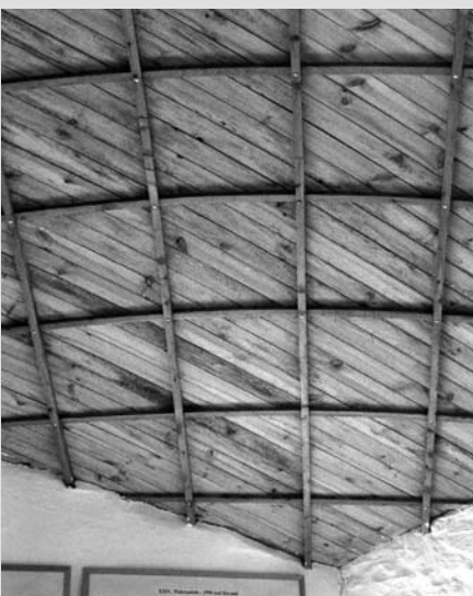
The gridshell roof structure comprises three layers of 12-millimetre thick timber planks fixed on top of a slender timber shell. The timber is left exposed internally.
