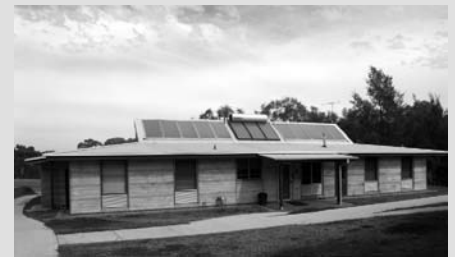
The typical student accommodation building has two types of roof-mounted solar panels. One thermosyphon flat plate collector in the centre of the array provides domestic hot water, which is stored in a tank above the panel. On both sides of it are flat plate collectors providing hot water for space heating.
