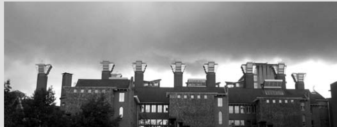
The tall chimneys provide ventilation to the teaching rooms.
