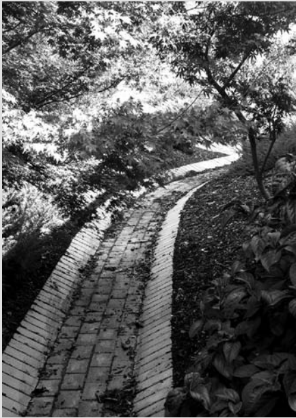
Swales and open waterways direct the rainwater to the wetlands.
