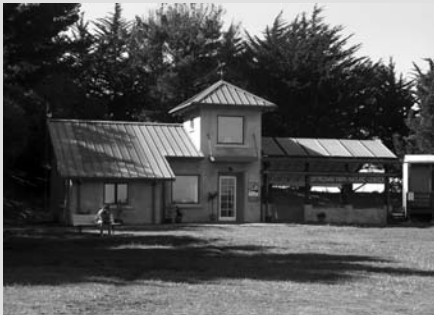
The Shorebird Nature Center in Berkeley is a passive solar building made of straw bales. It makes use of recycled materials and timber from managed forests. It also has a solar thermal and PV installation.
