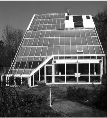
The conservatory is made with a standard prefabricated curtain walling system.
