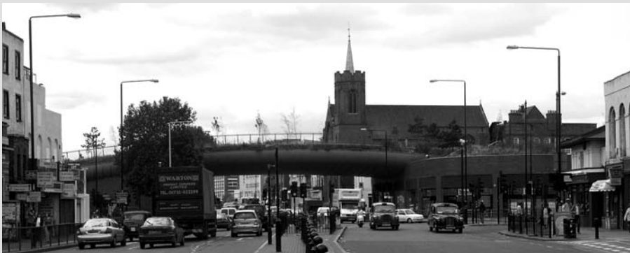
View of the bridge from Mile End Road.
