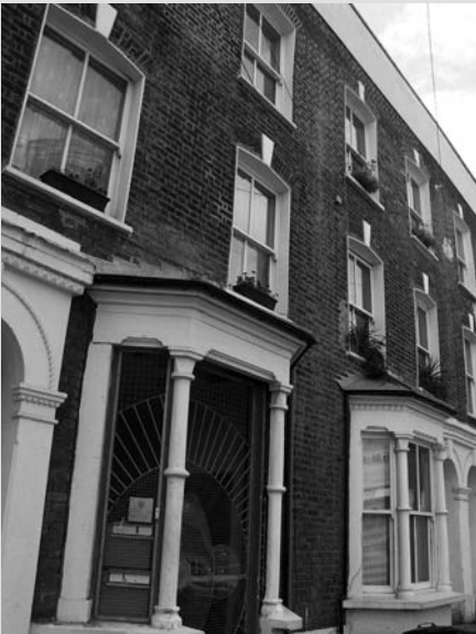
A converted bay window leads through a ground floor lobby to a rear courtyard and an external access stair, which provide access to the flats.
