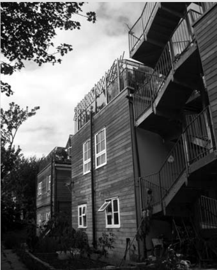
To the rear are the extensions clad in cedar, metal stairs to access the flats and communal gardens for growing foods and ornamental plants.
