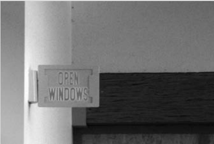
The sign tells occupants when conditions are appropriate for opening windows to cool the office.
