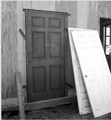
The Hidden Villa chicken house is designed to make use of reclaimed doors, windows and timber studs, rafters and joists.
