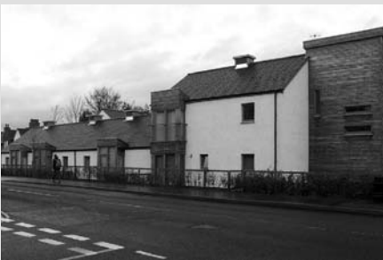
View of the Toll House Garden houses from the street. The chimney-like structures on the roof are the dynamic insulation ventilation inlets.
