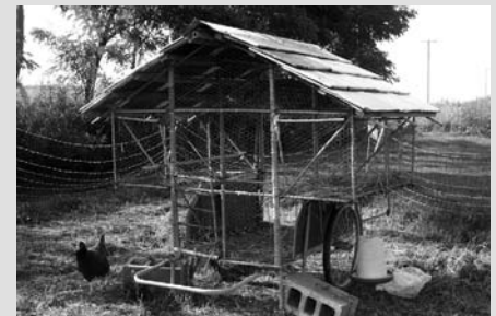
The Macoskey Center chicken house makes use of a reclaimed cart, timber sections, timber boards, and offset printing sheets.
