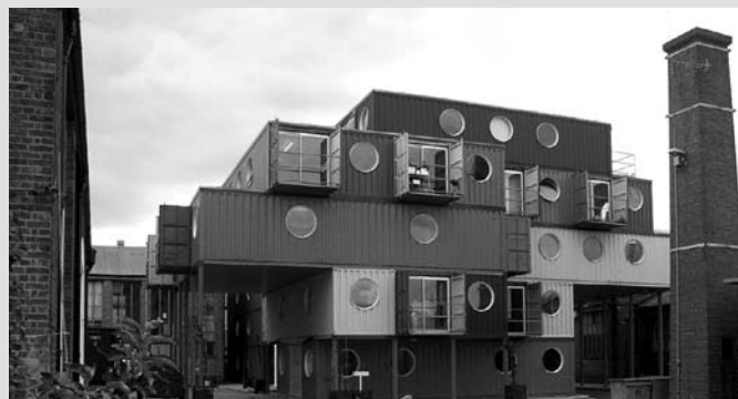
The brick contrasts with the brightly-coloured containers of the front block.
