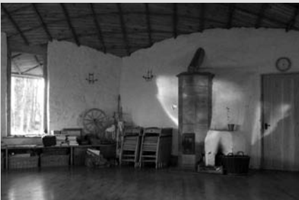
Internally, the gridshell has an exposed timber roof and a timber floor.
