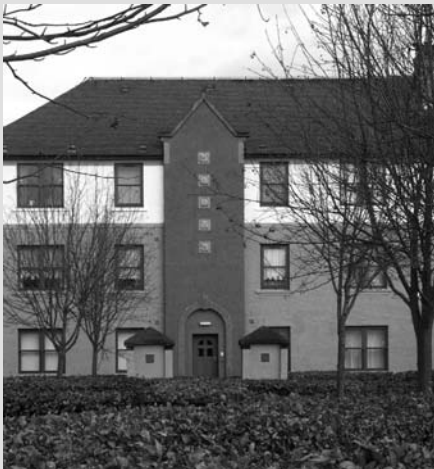
The existing blocks were refurbished.
