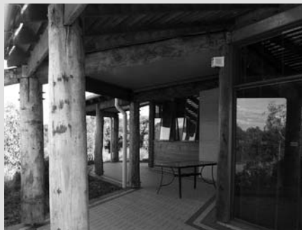
The building applies passive solar design principles, protecting the building from high level sun.
