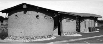
The cob walls are protected by an overhanging corrugated steel roof.
