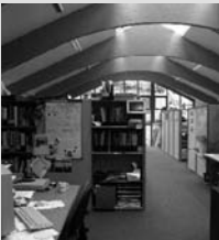
The rooflight is the main source of light in the first-floor offices. At the far end is the south-facing glazed elevation which also contributes natural light.
