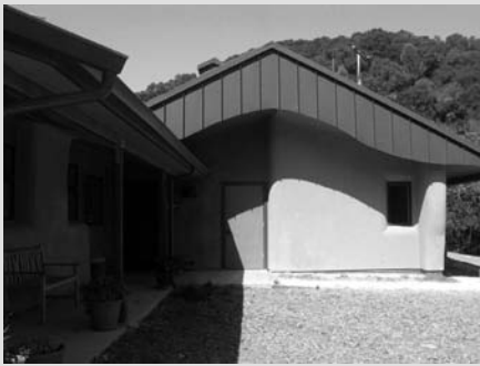
The overhanging roof provides protection for the bale structure and solar shading for the building. It also creates a seating area in the shade.
