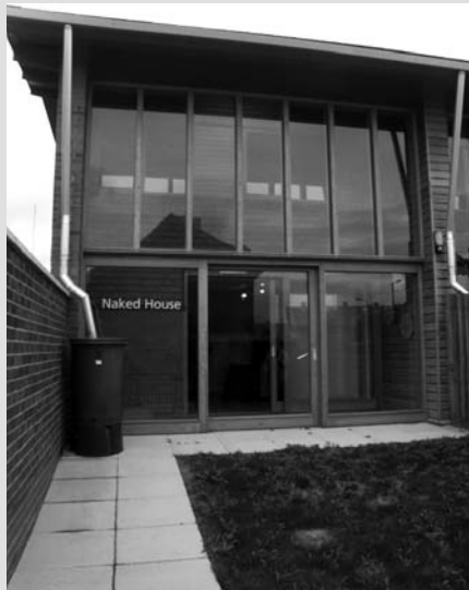
The south-facing houses have a fully glazed elevation to take advantage of the solar gains.
