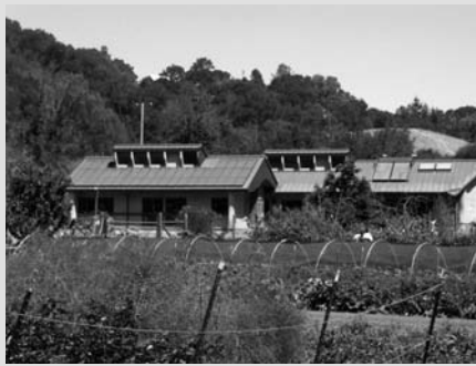
View of the Wolken Center from the south. In front is the vegetable growing area. The solar hot water panels, the PV and the clerestory windows are on the south-facing roof.
