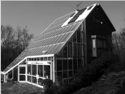
The house is designed to be passive solar and also includes active solar technologies.
