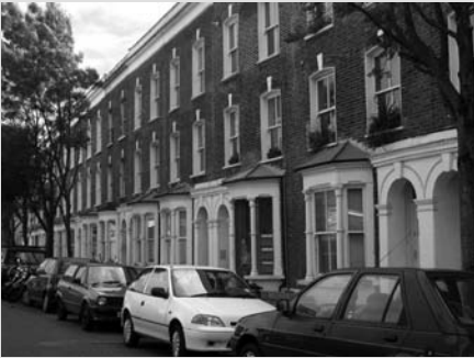
The Victorian houses were renovated, extended and reconfigured to provide maisonettes and flats with integrated work facilities.
