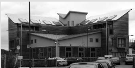
The flats for sale are situated on the north-west corner of the site together with the visitors' centre.
