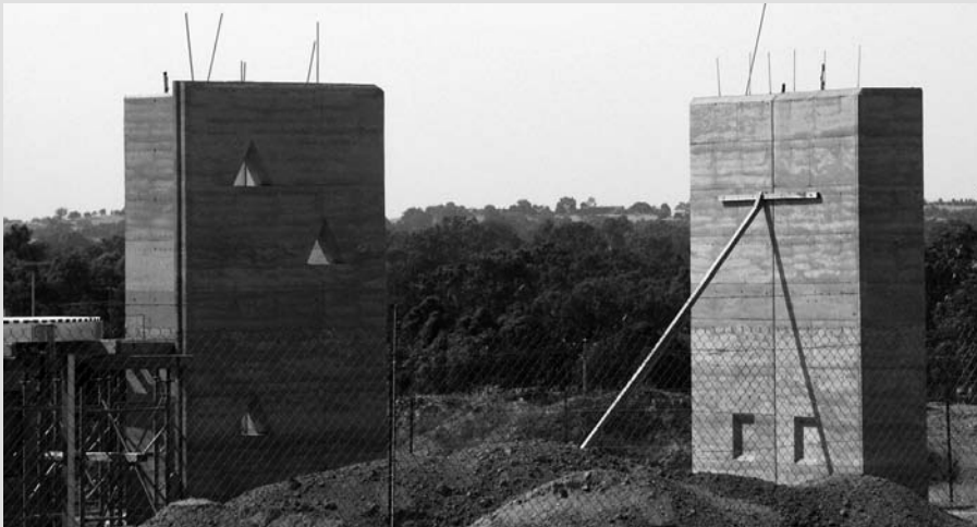
Rammed earth walls being erected for the new teaching block.
