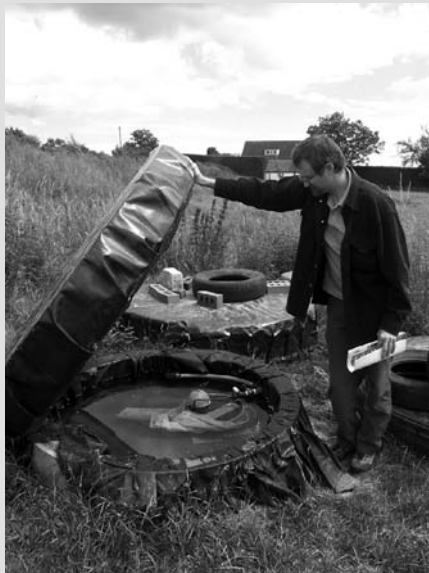
The water from the reservoir is passed through sand filters before being fed into the houses
