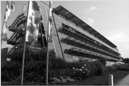
The Solar-Fabrik viewed from the road.
