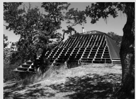
Timber louvres are designed so as to allow maximum natural light through the glazed structure, but prevent direct solar penetration, heat gain and glare.
