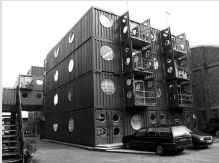
The rear block is made by stacking the containers one on top of the other in a regular manner.
