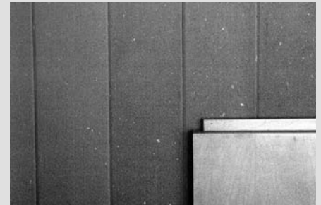
Trex used as decorative panel on the kitchen counter of the Environmental Showcase Home in Phoenix, Arizona, US (see case study, p.262).
