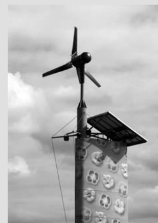
A small wind turbine and PV panel, which power the sign lighting, are symbolic of the sustainable building approach.
