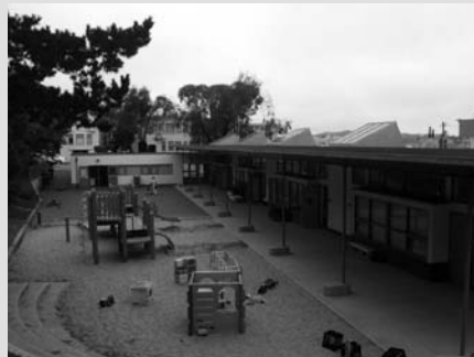
The classrooms face onto the play area as well as the gardens. PV panels are integrated within the rooflight over the toilets.
