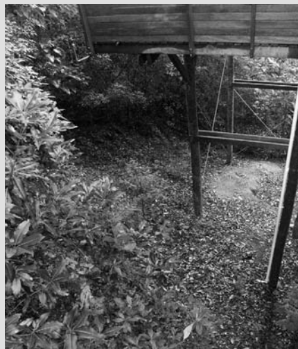
The pavilions are supported on slender timber posts placed on small foundations.
