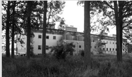
The entrance elevation on the north side of the building. The natural landscape around the demolished club house was left practically untouched.
