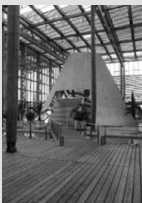
The roof above the library and the wall beyond are a combination of PV panels and clear glass double-glazed units.
