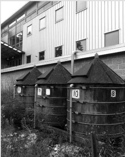
Smaller tanks collect rainwater from secondary roofs and release it slowly into the ground.
