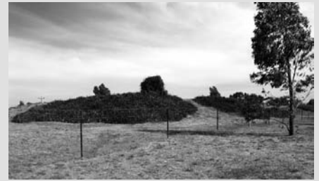
The reservoir is hidden behind the mound. The fencing is to prevent unauthorised access the site.
