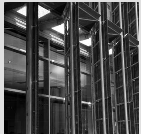
The shading on the north side, made of perforated metal, is both horizontal and vertical.
