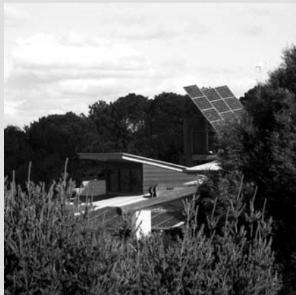
The solar hot water panels are located on the roof and the PV on the 'power tower'.
