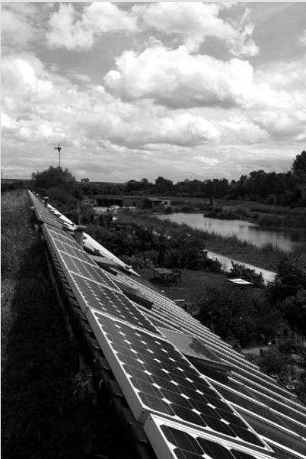
View from standing on the bermed side of the roof of the houses. A PV array and the conservatory both harness the sun's energy for use in the houses.
