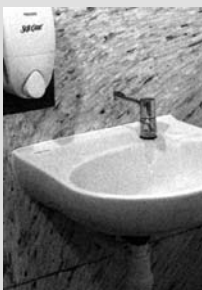
Wall cladding made of recycled plastic bottle in the Sainsbury's store in Greenwich (see case study, p.232).
