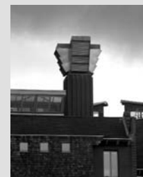
The chimneys for the lecture theatres are on the right of the tall stack and have glazed vertical openings.
