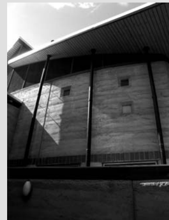
Composting toilets vent pipes on teaching block venting above roof level.
