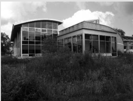
The Living Machine is situated in the small block on the right, which also includes the lecture hall, and is linked to the main teaching building.
