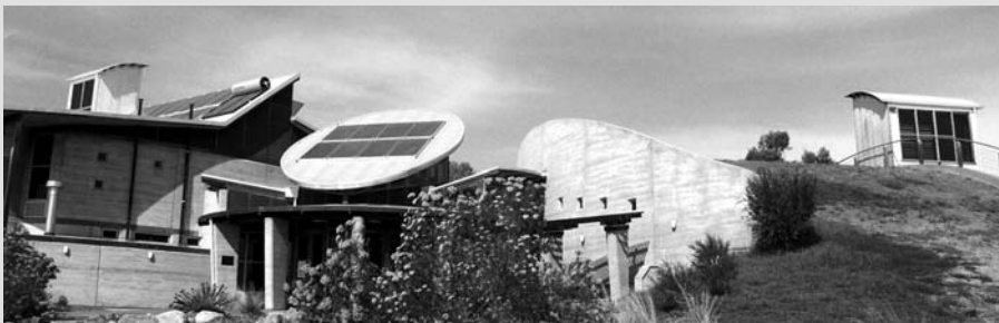
On the right the earth-bermed lecture theatre with the central vent. The theatre is accessed through the circular link which connects the theatre to other teaching facilities.
