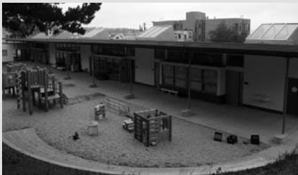
The south-facing classroom windows look out on the play area. The rooflights with PVs are visible from the communal garden around the school.
