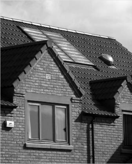
All houses have solar panels. Also visible on the roof is a light pipe that transfers light several metres into windowless parts of the building.
