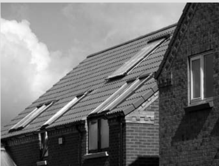
On the roof above the three rooflights is an evacuated tube solar panel.
