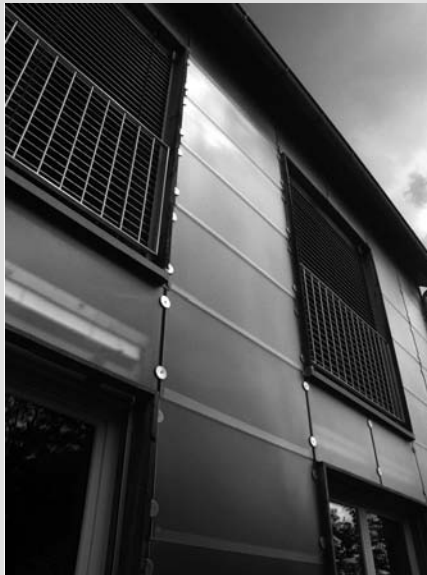
The external glass cladding is fixed over the cardboard honeycomb insulation.
