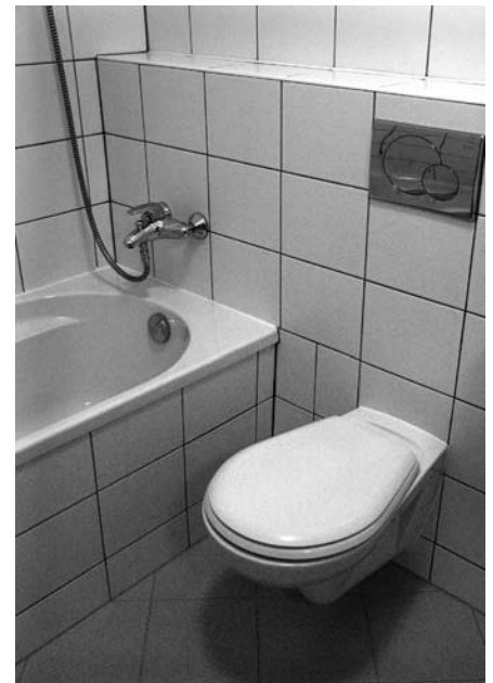
Dual flush WC in Barling Court housing (see Chapter 2.2).
