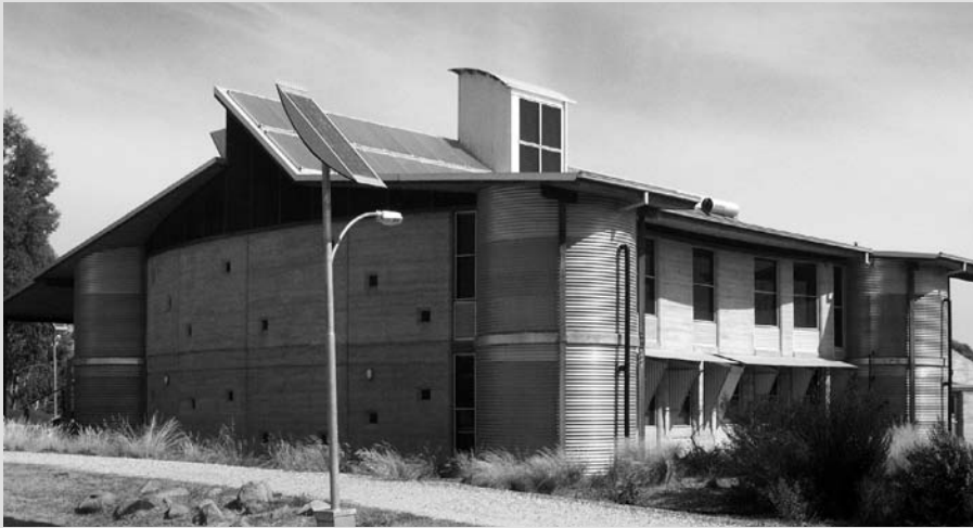
Teaching block with rammed earth end walls, roof vent and window shading.
