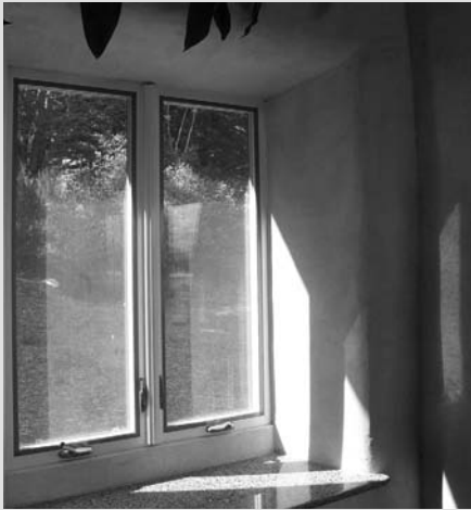
A window sill made with recycled post-consumer glass set in a resin mix at the Shorebird center in Berkeley, California, US (see case study, p.242).
