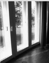
The double windows on the south elevation.
