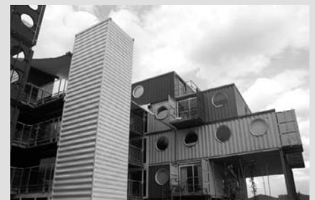
The upturned container is used as a stair core. Planting is being introduced at ground level to soften the environment.
