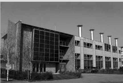
The Building Research Establishment Building 16, designed by Feilden Clegg Bradley, is a ground-breaking building in terms of environmental performance in general. In addition to using recycled and reclaimed materials, it is designed to be energy efficient through the use of natural ventilation in the offices and ground water cooling in the lecture room. It also has a PV array.
