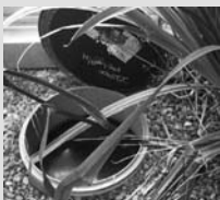
An inspection chamber is set in the 1-metre thick layer of planted gravel.
