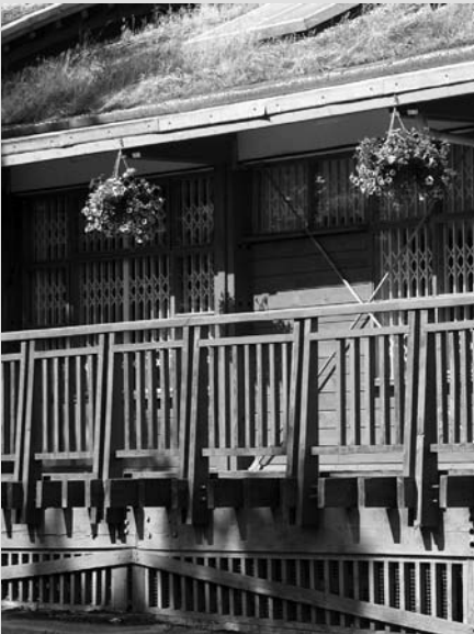
The timber structure was screwed and bolted together by trainees, while the grass roof was installed by specialist contractors.
