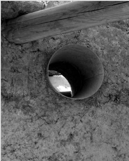
Reclaimed buckets are used to make openings.
