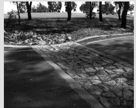
Waterways crossing the roads direct the collected rainwater and create a traffic calming device.
