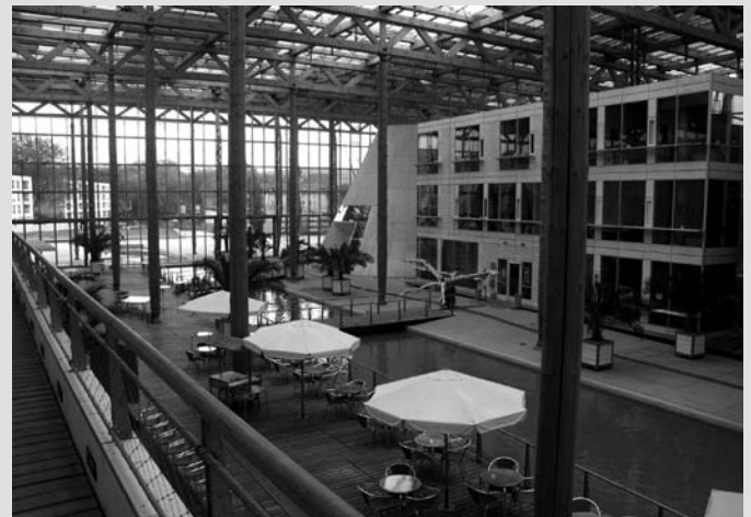
A glazed canopy with PVs covers individual buildings. Guidance strips on the ground, made of different colours and textures, lead the visually impaired around the complex.
