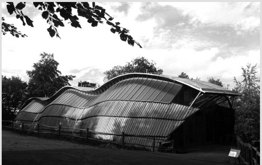
View of the east entrance and the south elevation with its cedar cladding, polycarbonate clerestory and central roof ribbon made of Roofkrete.
