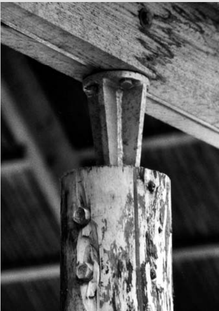
The timber sections of the covered entrance area are bolted or screwed to facilitate their dismantling.
