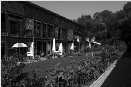
The south façades are fully glazed to maximise solar gains.
