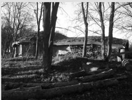
The gridshell roof forms a rounded and soft structure resembling a natural feature. On one side of the main space are storage facilities and on the other are offices.
