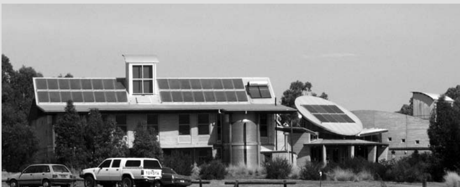
Teaching block (left) and adjacent lecture theatre (right). The teaching block has an extensive array of solar panels for space heating and cooling and one solar panel to provide water for washing. A natural ventilation chimney is centrally positioned.
