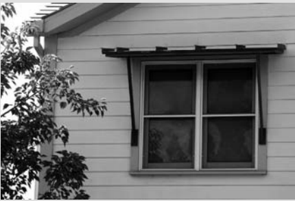
The window is shaded from the high summer sun. The cement-fibre cladding reduced the use of solid timber.
