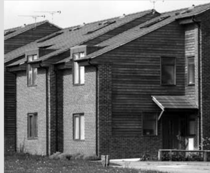
The brick and timber cladding give the houses a familiar yet contemporary appearance.
