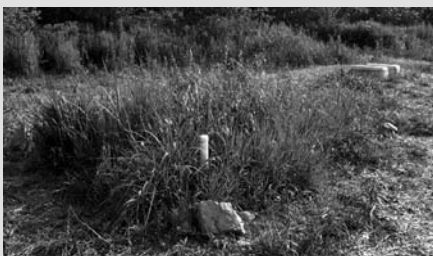
The greywater treatment system is underground, with only the testing tubes and the septic tank hatches visible.
