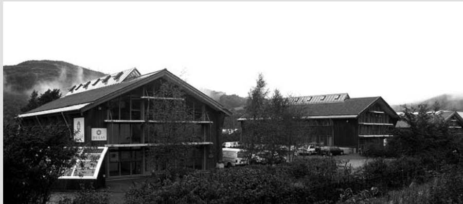
The two-storey units have a long rooflight and glazed south-facing elevations.
