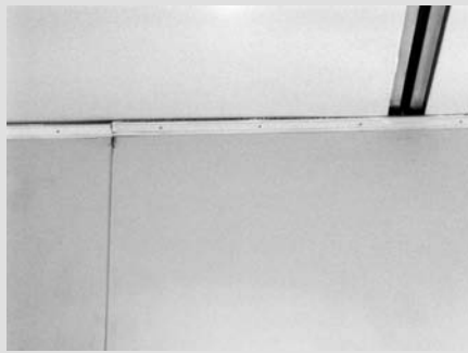
The top section of the wall includes a trim and the track used to move the partitions is recessed in the ceiling
