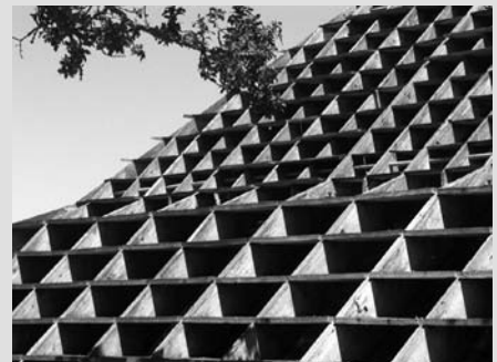
Timber louvres are designed so as to allow maximum natural light through the glazed structure, but prevent direct solar penetration, heat gain and glare.
