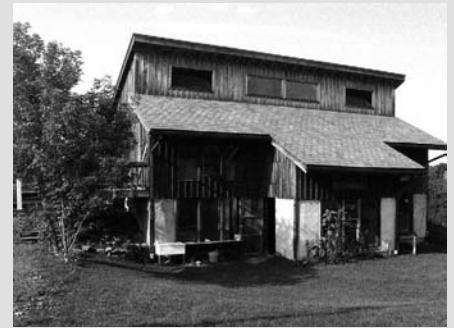
The Macoskey Center (see Chapter 4.6) comprises a couple of small buildings refurbished with much care. The barn roof is covered with reclaimed tiles and the barn structure is a reclaimed timber frame.
