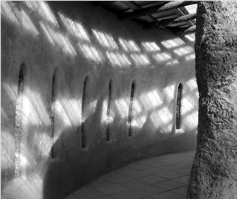
The larch thinnings support the roof, their natural texture matching that of the cob.
