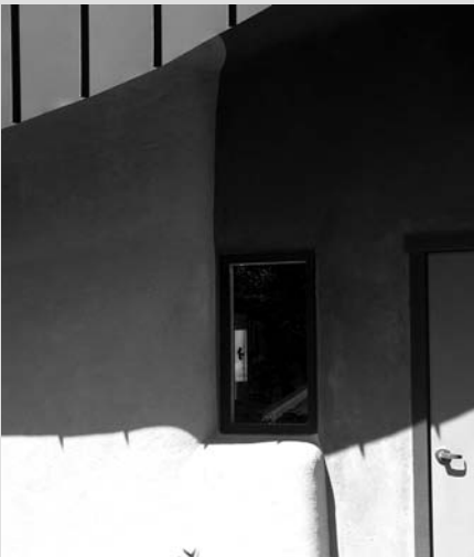
The straw bale walls have been covered with a layer of mesh and render and lime washed.
