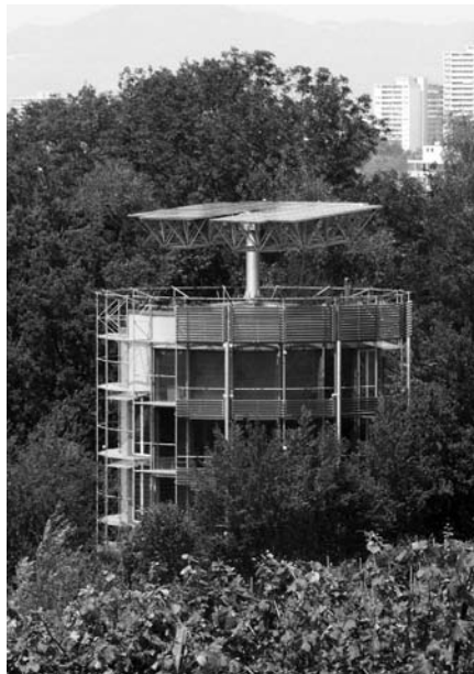
The Heliotrop, in Freiburg, is a low energy dwelling and work place designed to track the sun to optimise its solar orientation. Its 54 m 2 PV installation with a peak output of 6.6 kW exports 5 to 6 times the energy the building uses (Architect Rolf Disch).
