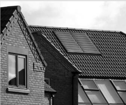
A flat plate collector.
