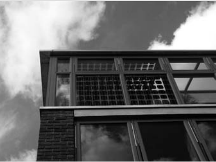
The development makes use of energy from a CHP system and building-integrated PVs.
