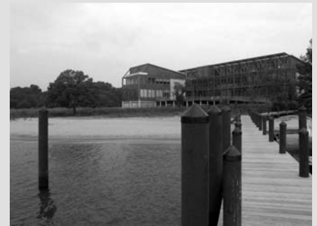
The long block houses the main office space, and the smaller block houses the conference rooms.
