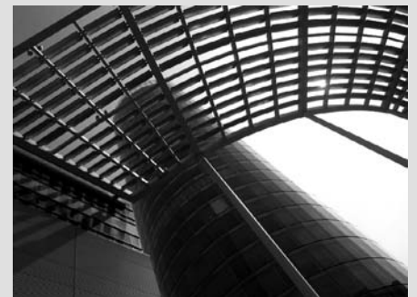
The entrance canopy is covered with 192 metal louvers with PV cells. The total installation has a peak rating of 19KWp.
