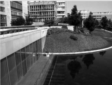
View of the glazed front to the restaurant.
