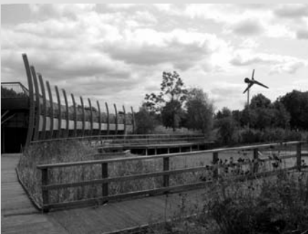
An ecology centre and an art centre have been built within Mile End Park. The bermed buildings are energy efficient – they have a seasonal heat storage and make use of wind power.
