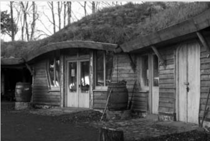
The Pishwanton gridshell (see case study, p.138) included the use of clay-based materials for the construction of some of the walls.
