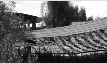
Timber and copper shingles on the roof.
