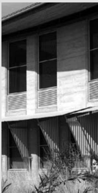
The naturally ventilated teaching block with a central vent. Note the glass louvres over the doors, which allow cross-ventilation from the office windows to the central vent.
