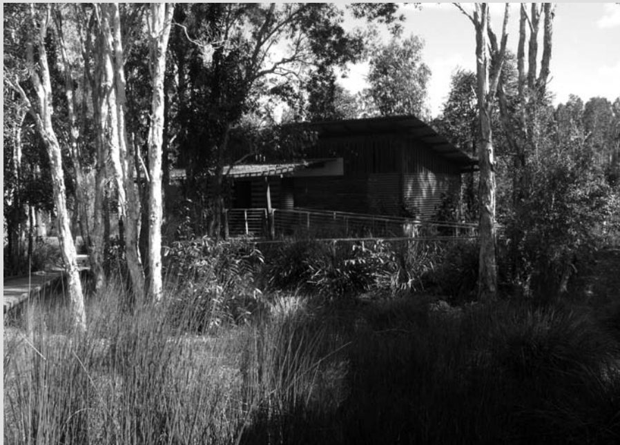
The toilet block is situated between the car park and the visitors' centre.
