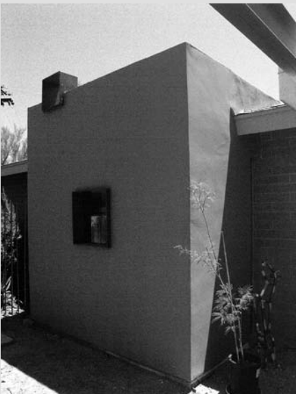
One of the extension elements made of SIP, rendered and painted in purple. Other extension elements are painted in muted green and yellow.
