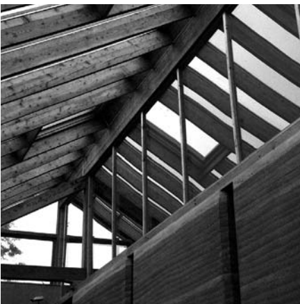
The rammed earth wall supports the roof.
