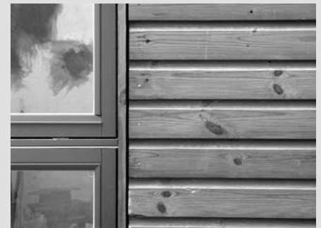
The ThermoWood creates an interesting contrast to the painted timber windows.
