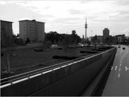
The entrance to the tunnel. The road drops underground and the park is elevated over the road.
