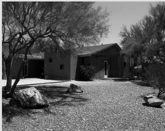
View of entrance. The addition of extension elements alters the aesthetics of the building, giving it a contemporary feel.
