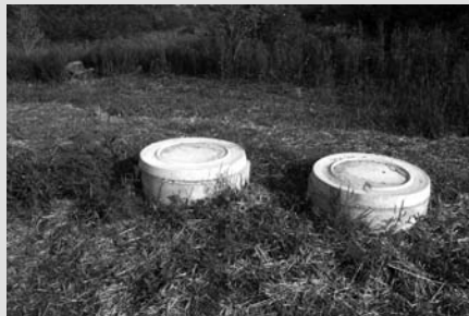
The septic tank access hatches.
