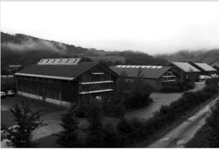
From the left: Units Two, Three, Four and Five. Units Four and Five have large south-facing, roof-mounted PV arrays.
