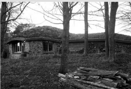
The Pishwanton gridshell in the woods west of Edinburgh has an extensive green roof. Its natural shape makes the building look almost like part of the landscape (see case study).
