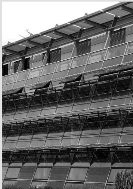
Some of the PV panels are integrated within the glazed elevation and some are mounted on steel supports and shade the glazing. Opening vents in the façade provide ventilation.
