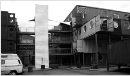
The front and rear blocks are connected to a stair tower made with an upturned container.
