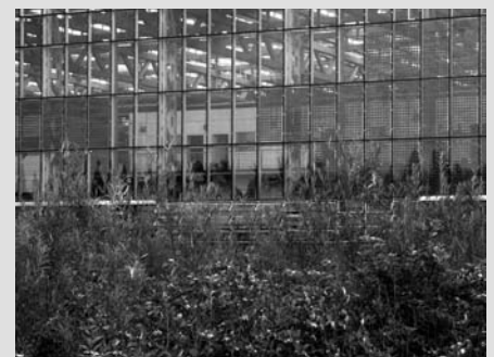
The PVs are integrated within the glass envelope.
