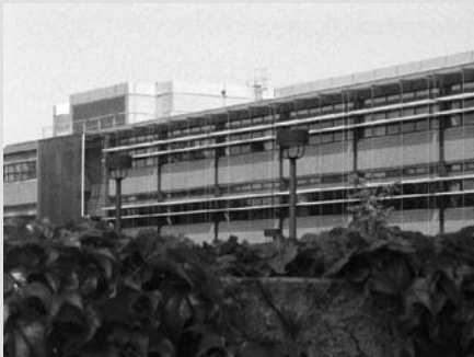
The south façade is protected from the sun by aluminium louvers. Pre-fabricated panels of stack bonded bricks form the wall cladding.
