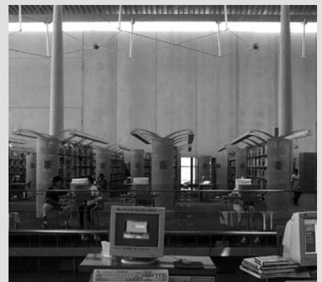
A lighting strip separates the wall and roof.
