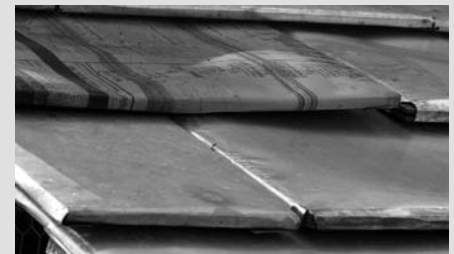
The roof tiles of the chicken house are made of reclaimed metal offset printing sheets.
