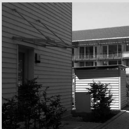
The Solarsiedlung houses (see case study, p.244) are timber-framed structures, with timber cladding externally. Internally, the ceiling timber structure is left exposed providing a large surface of a hygroscopic material.
