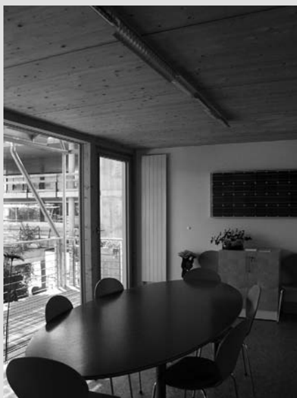
The Solarsiedlung houses (see case study, p.244) are timber-framed structures, with timber cladding externally. Internally, the ceiling timber structure is left exposed providing a large surface of a hygroscopic material.
