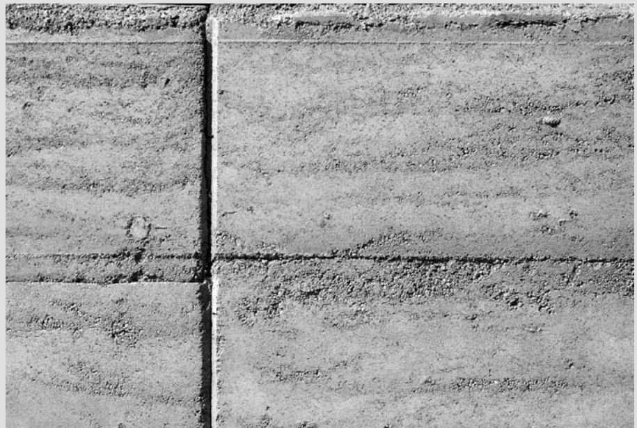
The rammed earth walls panel junction detail.
