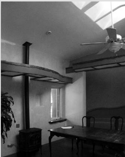
The soft curves of the straw walls give the interior a cosy feeling. The propane heater provides heat for extremely cold weather. The clerestory brings light into the rooms.
