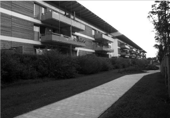
The concrete on the Neue Heimat blocks was made with revitalised water.
