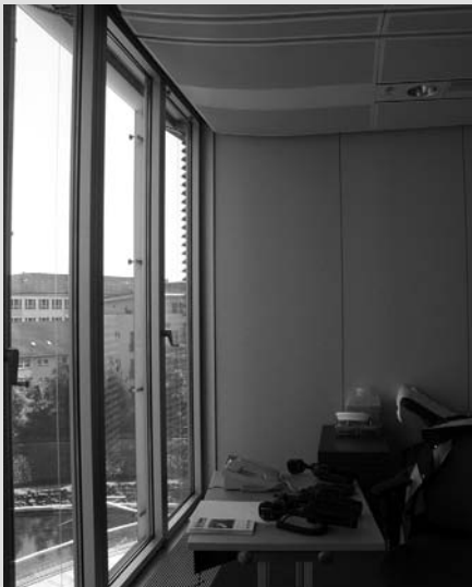
A 1.35m wide internal glazed element can be slid open to provide natural ventilation.
