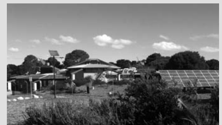
Solar hot water panels can be seen on the left-hand side of the roof, while on the right of the roof is a hot air panel and in front of the building a free-standing PV installation.
