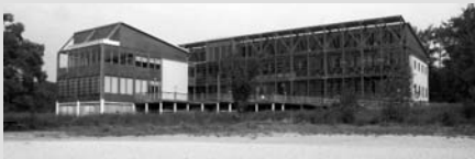
The Merrill Center is designed to be passive solar, uses energy-efficient appliances and renewable energy systems as well as being virtually water self-sufficient.
