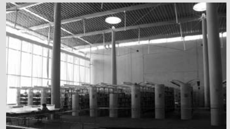
The rooflights are positioned above the concrete columns that support the 'tensegrity' roof.
