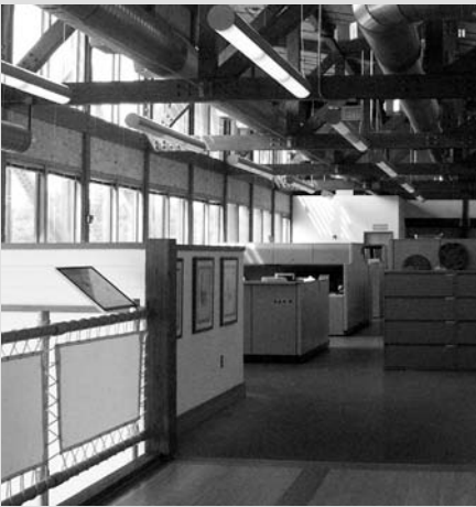
The workspace lights are controlled by movement and light sensors to avoid being left switched on unnecessarily. The overhead lights are controlled by light sensors measuring the level of natural light and dimming the lights when needed.
