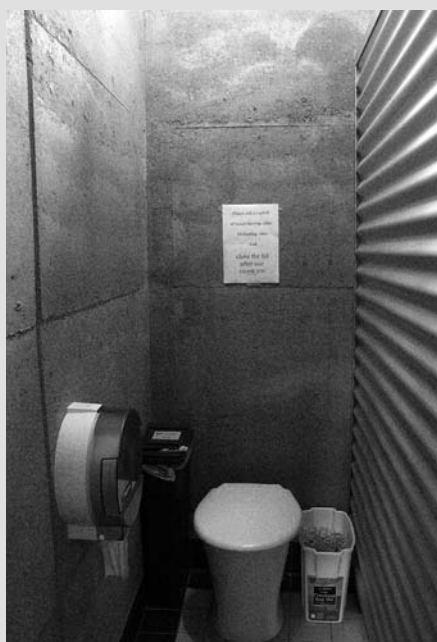
A composting toilet in the student building. Note the plastic container with wood shavings beside the pedestal. The toilet cubicle is enclosed by the rammed earth external walls and an internal metal partition.
