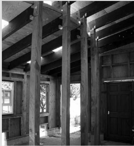
The Hidden Villa chicken house is designed to make use of reclaimed doors, windows and timber studs, rafters and joists.
