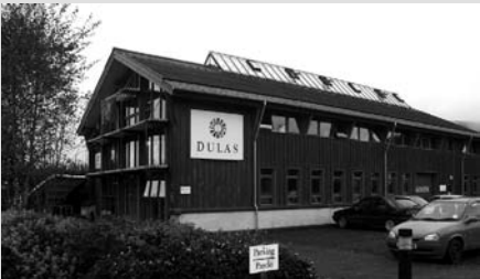
Unit Two. Horizontal glazed openings, as in rooflights, allow more light to penetrate a building than similar areas of vertical glass.
