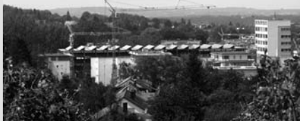
The roof-mounted PV panels are clearly visible from the neighbouring hills.
