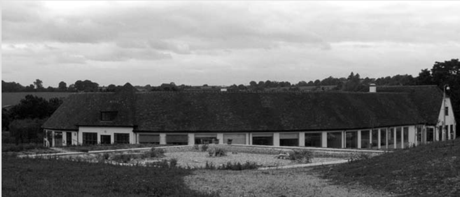
The BCZEB seasonal store has a polystyrene cover, which is weighted down with stones and some plants.
