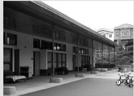
The south-facing classroom windows are protected by an ample overhang.
