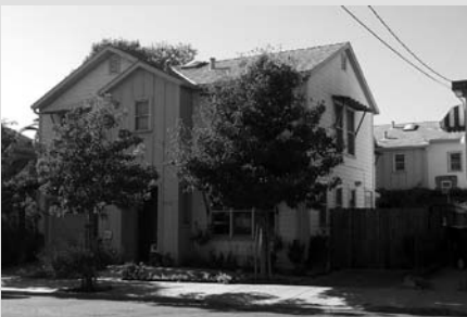
One unit is on the street edge and the other two are set back and accessed through a courtyard.
