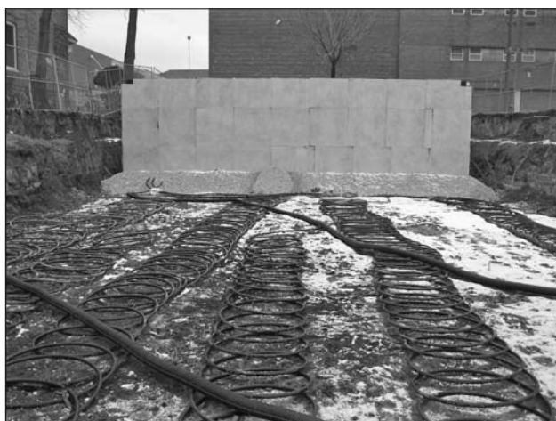
The installation of a home geothermal heating system.
