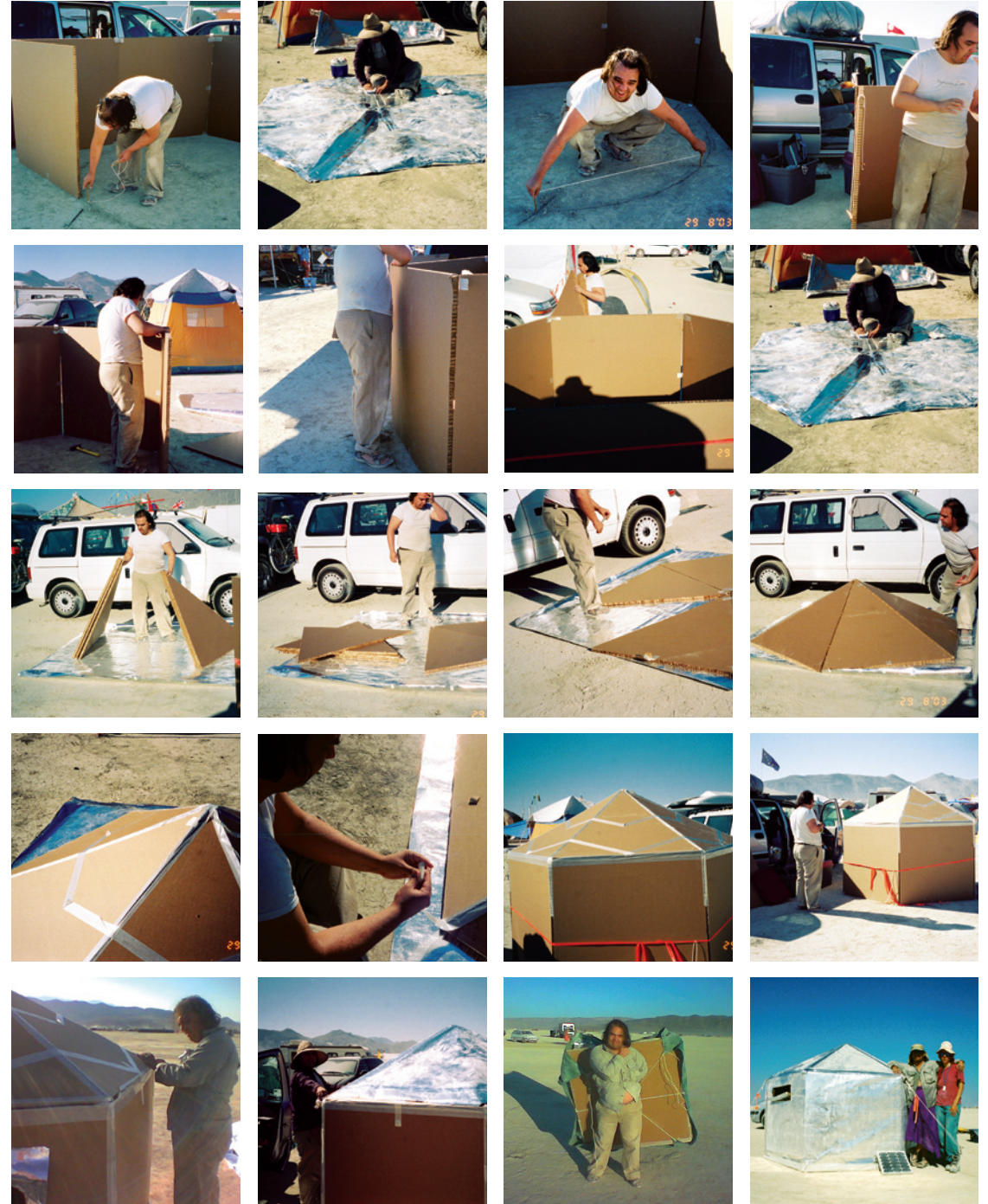
left to right, top to bottom The cardboard shell under construction; application of the reflective heat shield; transporting the shelter; the designer, left, with friend Beatrice Aranow in front of the completed structure
