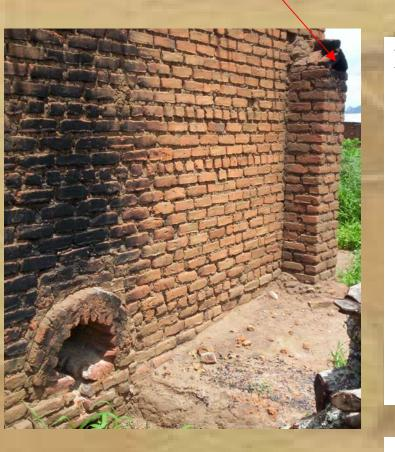
External (60cm) chimney draws air through tobacco. The entire barn is sealed with the exception of a single air inlet shown on next page
