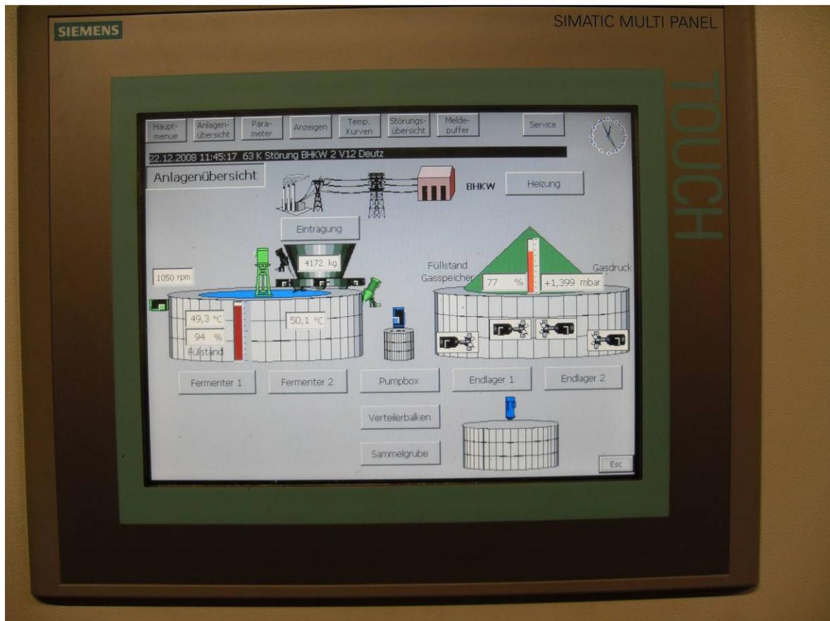
**1 Part of the AD plant control system that can provide a graphical display of many of the functions of the plant and its operation.**
