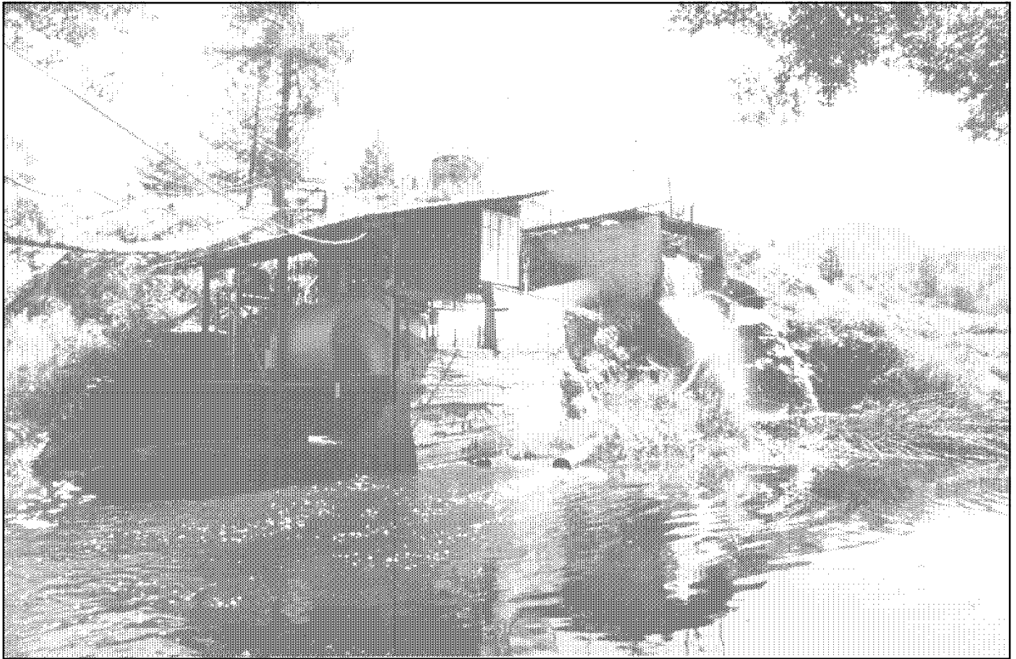
Above: Stuart Higgs' hydroelectric turbine generates power for two all-electric homes. On the left is the powerhouse holding the 30,000 watt alternator. To the right, overflow water spills from the fish guard. The day this photo was taken the turbine was producing 12 kw. (288 kwh/day) while cycling 770 pounds of water per second. Photo by Richard Perez
