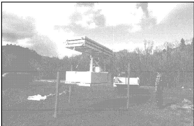
② Above: Voltar is jacked up and the pickup drives away. We used three jacks and a special jacking kit provided with Voltar. Photo by Therese Pepper
