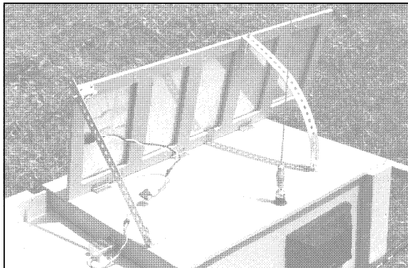
Above: PV module swings on hinges. Perforated metal strips hold module at proper angle to sun. Output from module passes through in-line fuse to controller.
