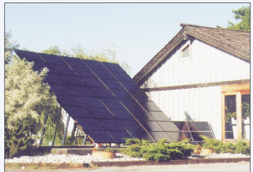
Our shop utilizes its own 2.5 kw array and 35 kw battery bank for daily power needs and testing of new products.
