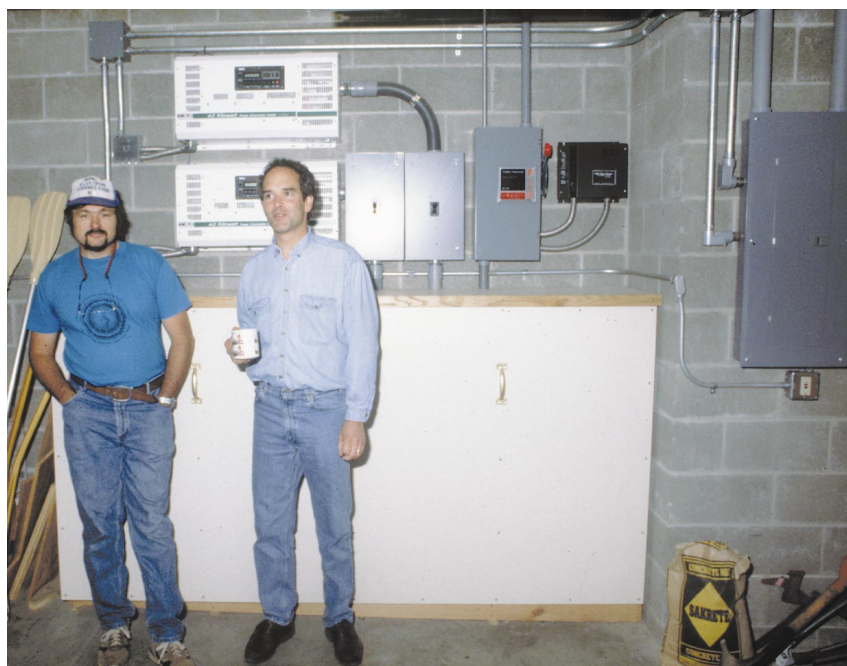
Top: The power center located in the garage. Note the ultrafine cabinets (with covers removed) that house the batteries.
