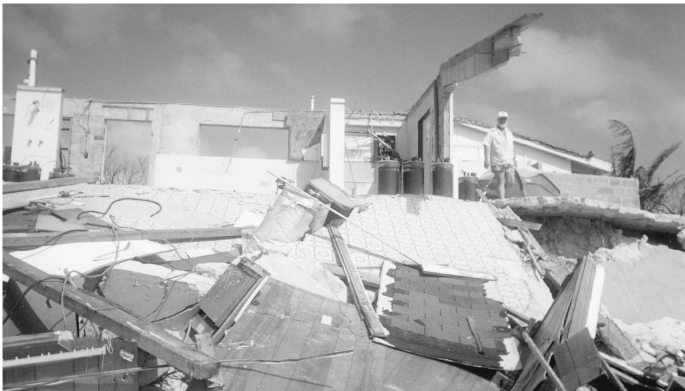
Above: The aftermath of Hurricane Luis at Frank Delisle's place in Antigua. Note some of the batteries still standing. The modules are somewhere under the mess fallen onto the beach. They survived intact.
