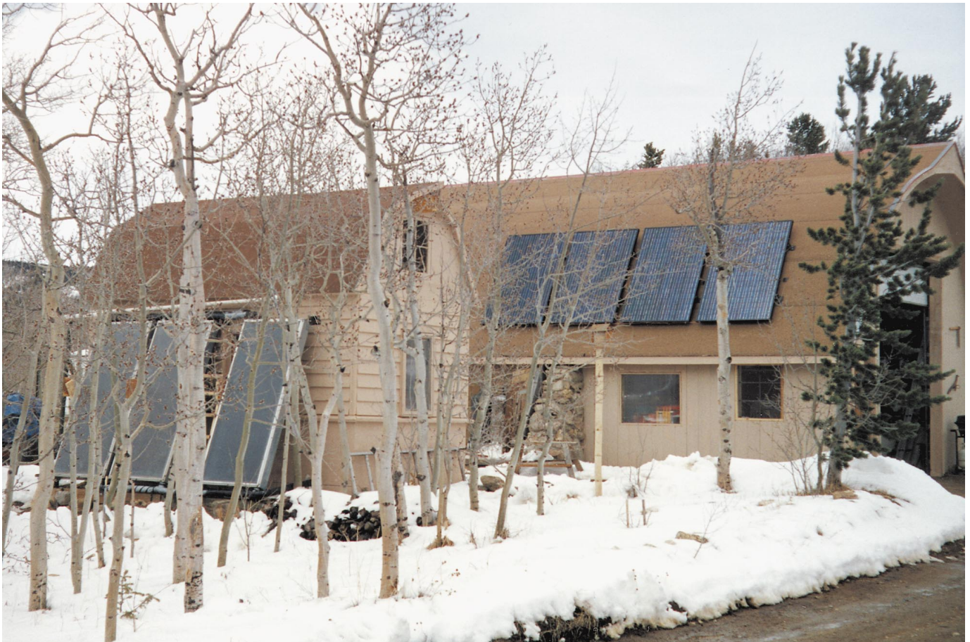
Above: Rob's shop with four 245 Watt ASE panels. The battery shed with solar thermal panels is in the foreground.
