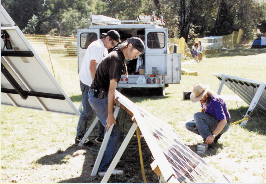
Above: The Alternative Energy Engineering crew setting up the PV system.
