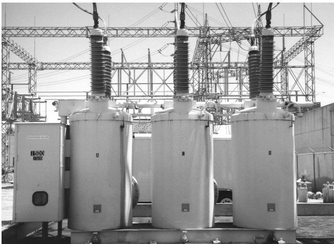
Picture 6, Above: Same as picture #5, however filled with insulating oil. The data in the text is from this oil breaker. Each tank has an insulating bushing on top that carries power through the breaker. Each tank has a moveable contact.
