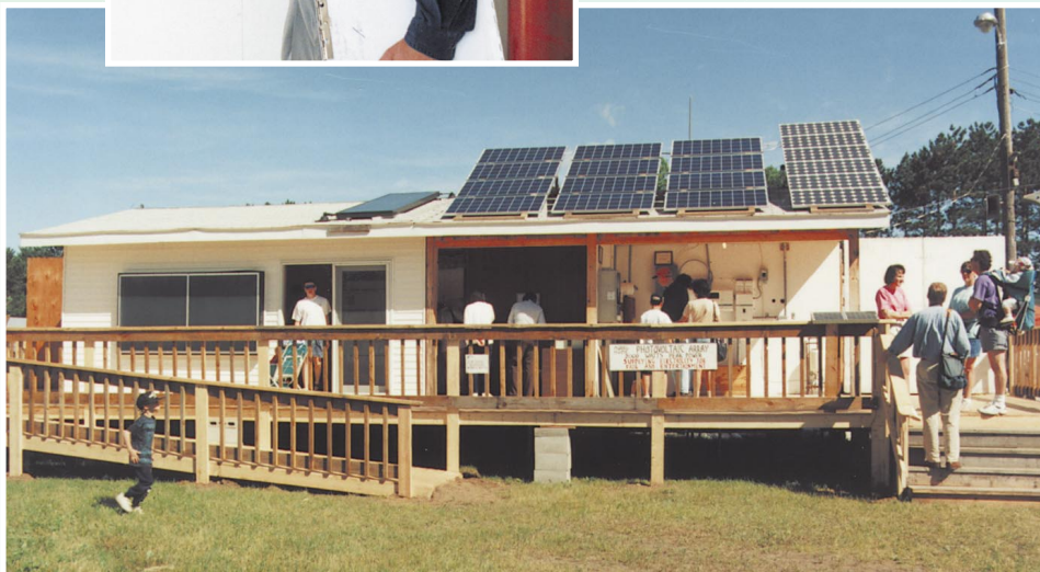
Model home: A whole house was built on site to show the integration of multiple systems in an energy efficient dream home.
