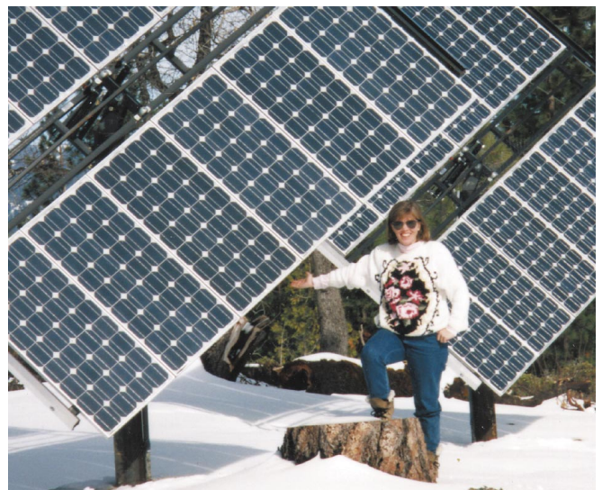
Below: Sylvia Leutz in front of the three tracked arrays of twelve Solavolt modules each.
