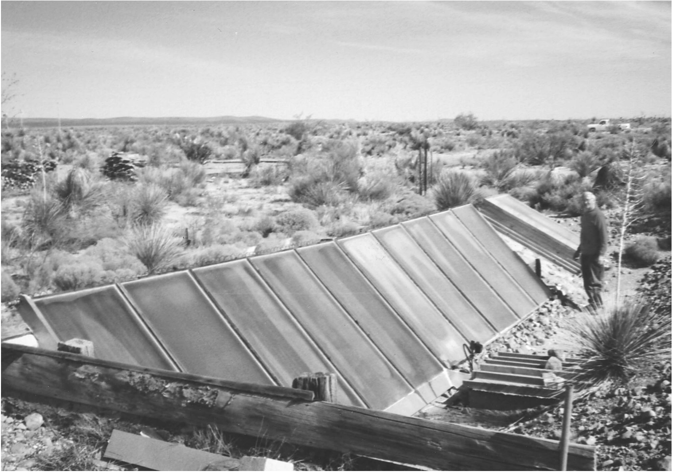
Above: Ten home-made solar heat collectors. Water sump is at bottom left. Rain gutter runs along bottom of panels, and is covered by sheet metal and rocks to keep out critters and rain water.
