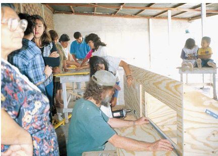
Above: Attaching the doors for the oven.
