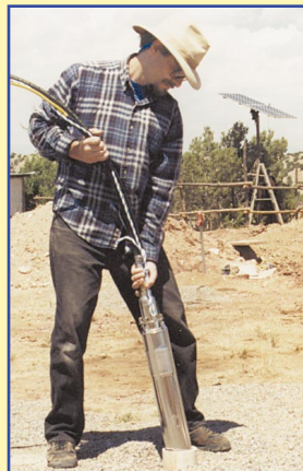
HP author Windy Dankoff installing a SunRise™ Pump
