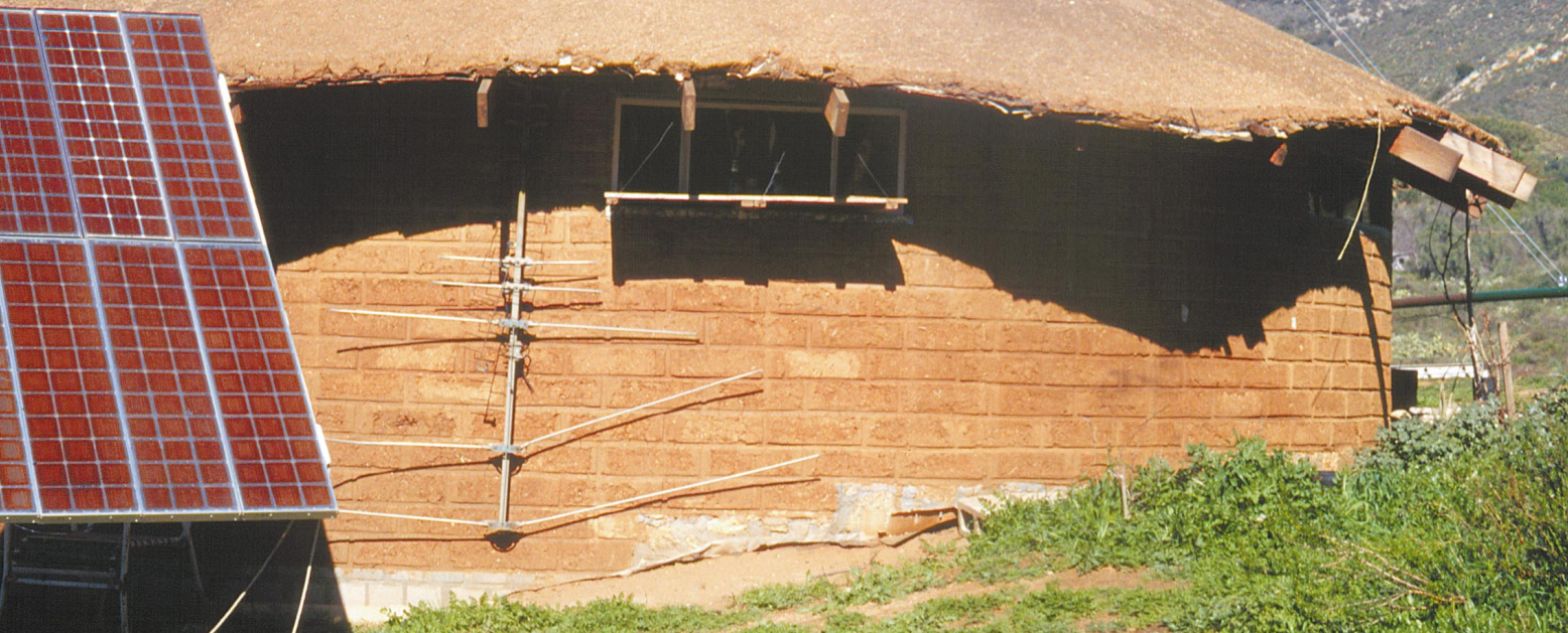
Above: Richard Dutton's round adobe brick studio with mud roof, and the QuadLams that power it.
