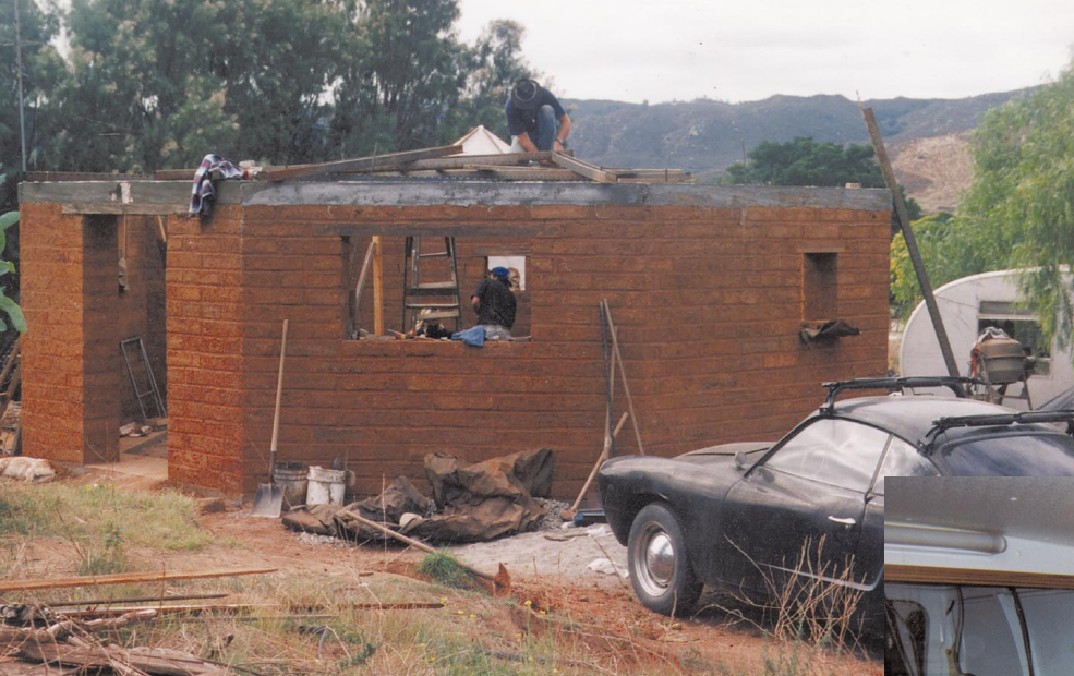
Left: Ready for the roof: The kitchen under construction.
