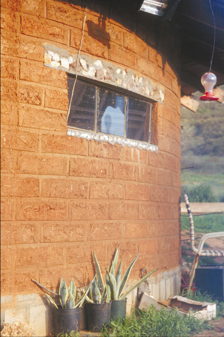
Above: Home-made concrete lintels save wood.
