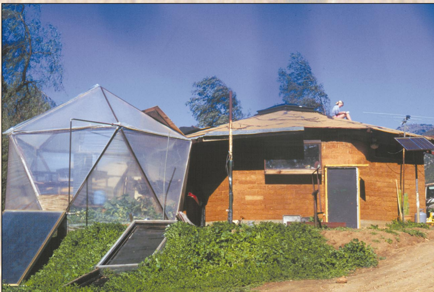
Above: The octagonal adobe kitchen, greenhouse, solar hot water panels, and solar hot air food dryer.
