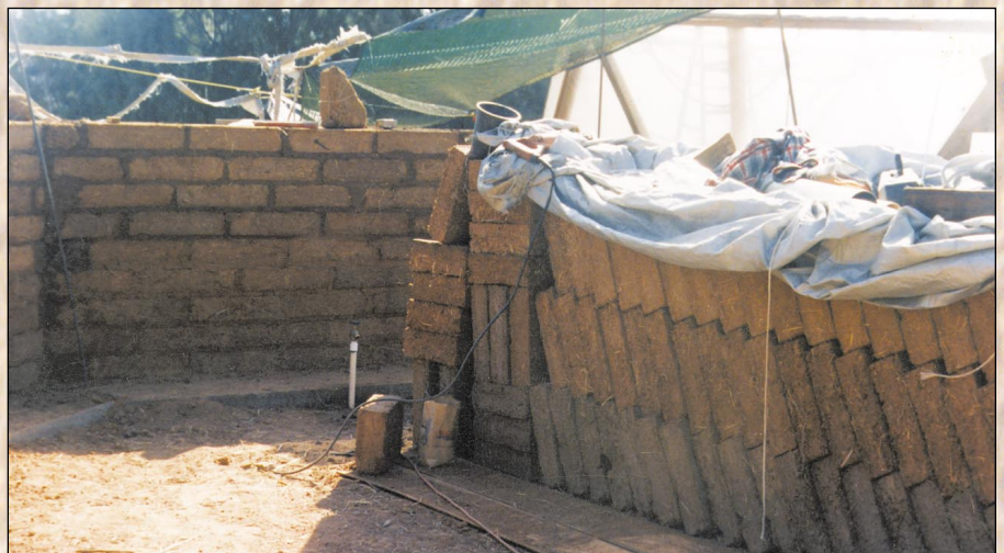
Below: Wall building in progress and bricks stacked for drying.
