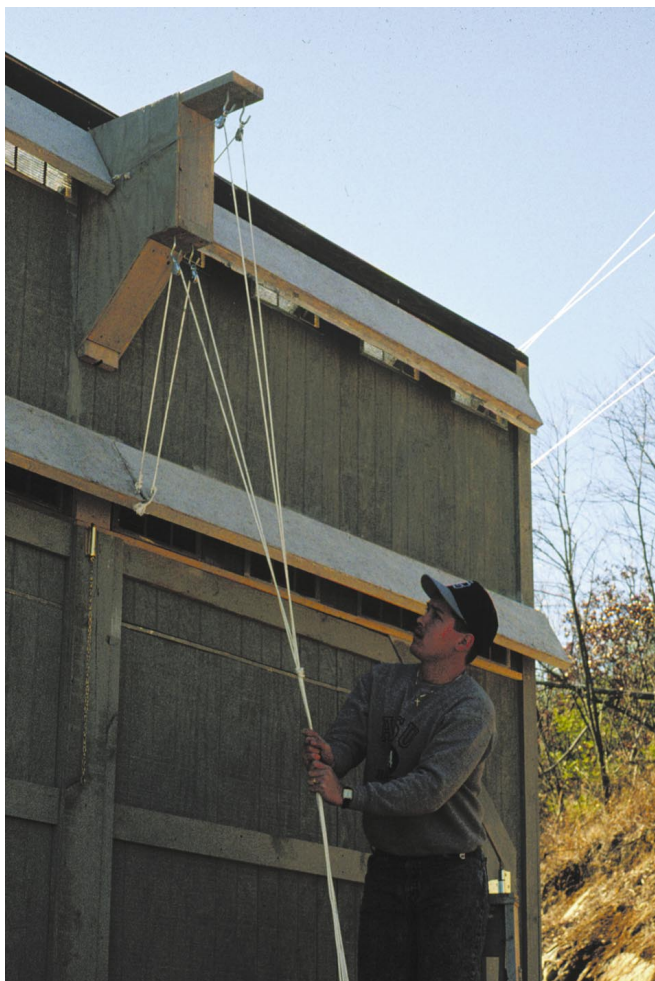
Above: Setting up vent control lines.
