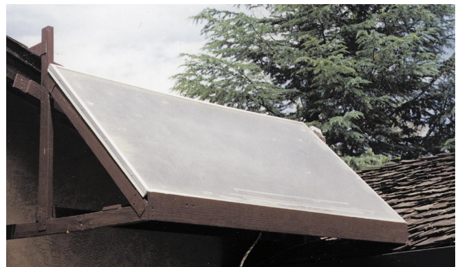
Figure 3: The solar thermal water panel.
