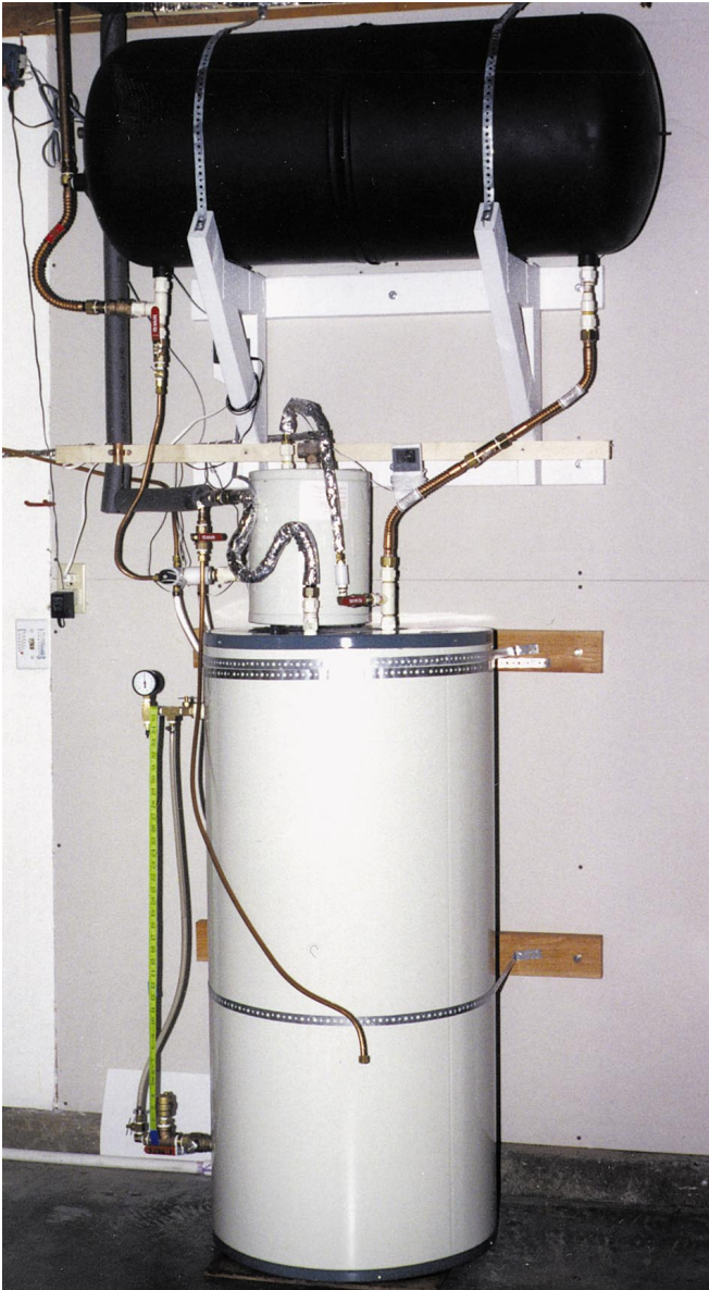
Figure 2: The gravity siphon system.
