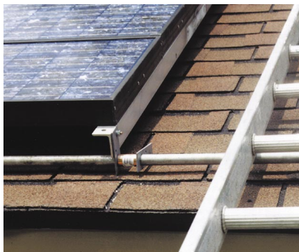
Left: Don Laughlin designed sub-array mountings to pivot for wiring access.
