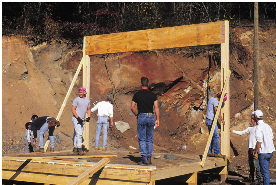
Above: Bracing the north wall.
