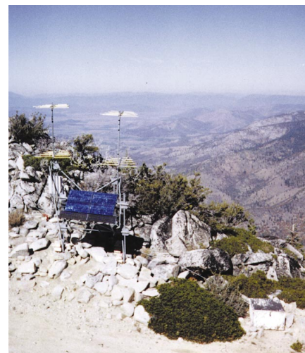
Above: Ariel view of Boulevar Mtn. shows the PV / Antenna arrays (left) and battery vault (lower right).
