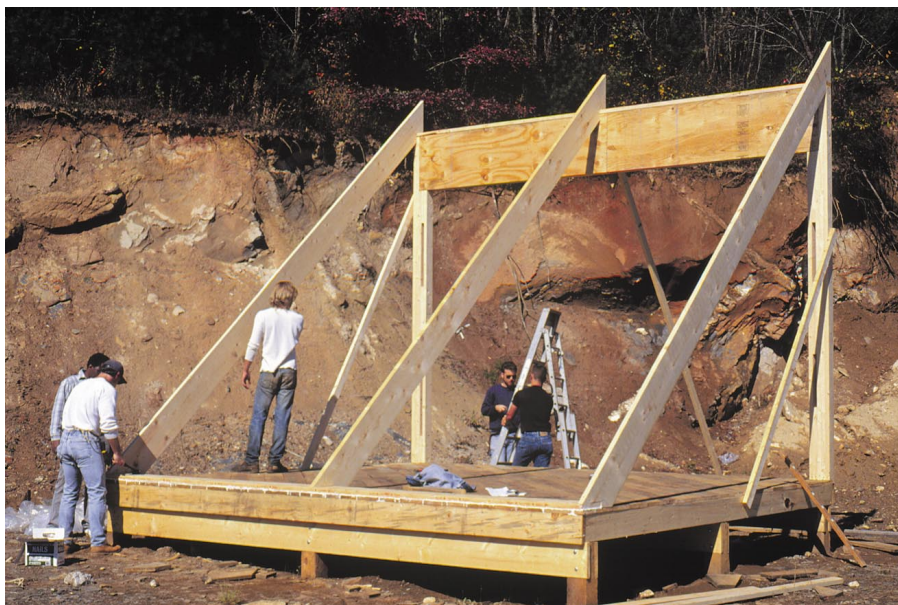
Above: Setting up 2 by 12 south wall rafters.
