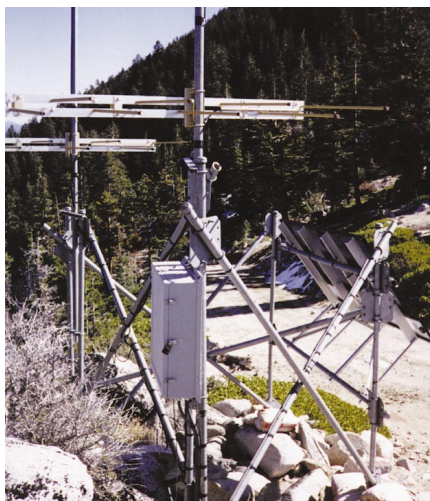
Above: The complex structure supports translator, PV panels, and four Log Periodic antennas.
