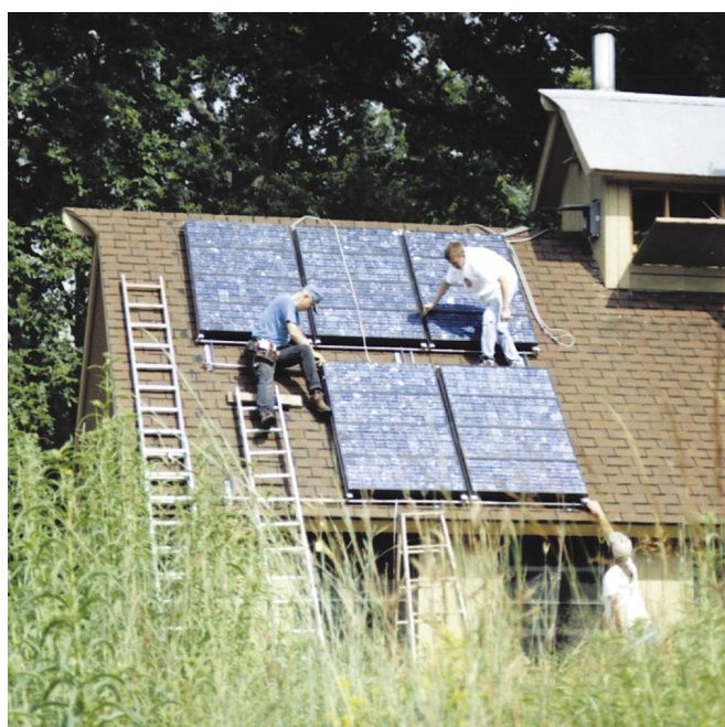
Below: Mounting the 24 Volt sub-arrays.
