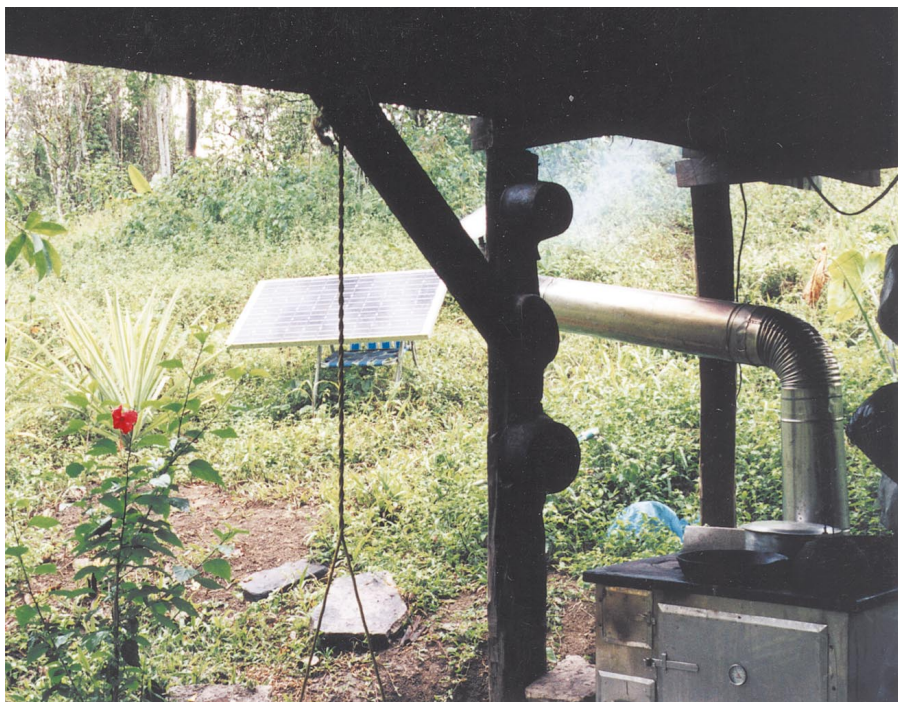
Above: A view from inside the open-air kitchen showing the wood-burning cookstove. Outside, the temporary "lawn chair" mount supports a 90 Watt Solec PV panel.
