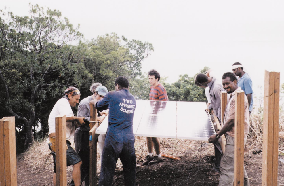
Above: Installing the almost horizontal PV array of twelve Siemens SP75s.
