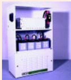
MPS shown with cover removed.
