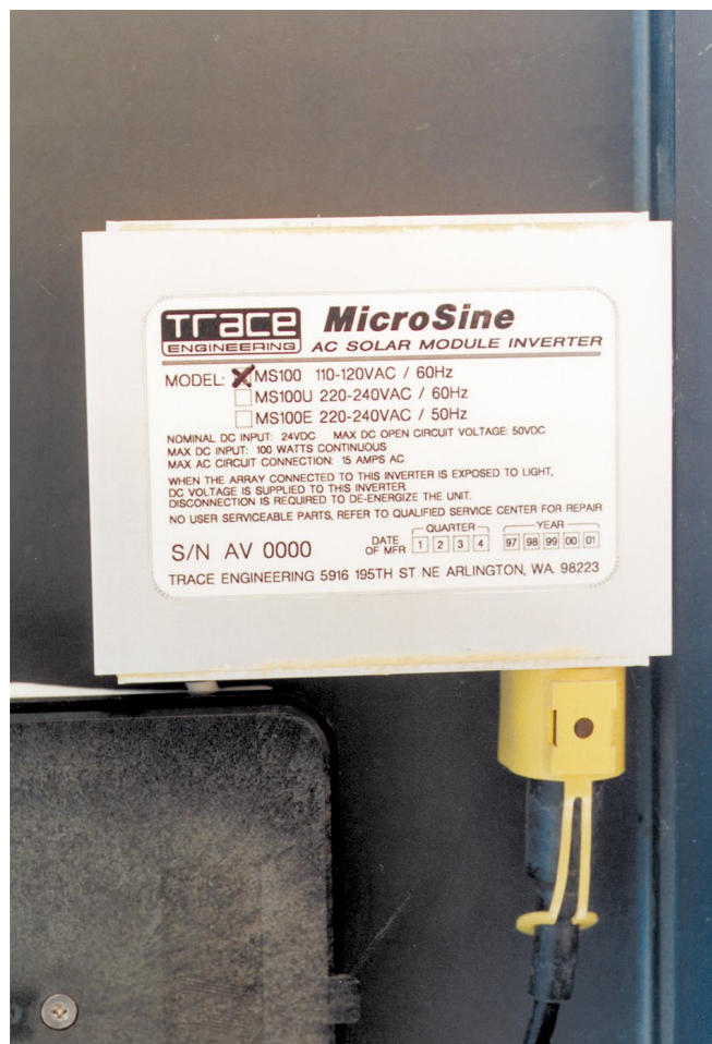
Above: The Micro Sine on the back of the 24 Volt PV.
