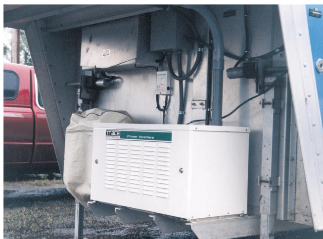
Above: The Trace battery box in place.
