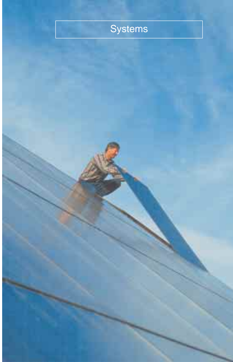
Above: Installing the high voltage ASE modules.
