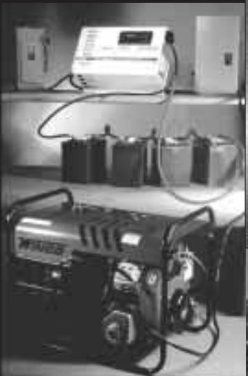
13 KW Inverter Generator System
