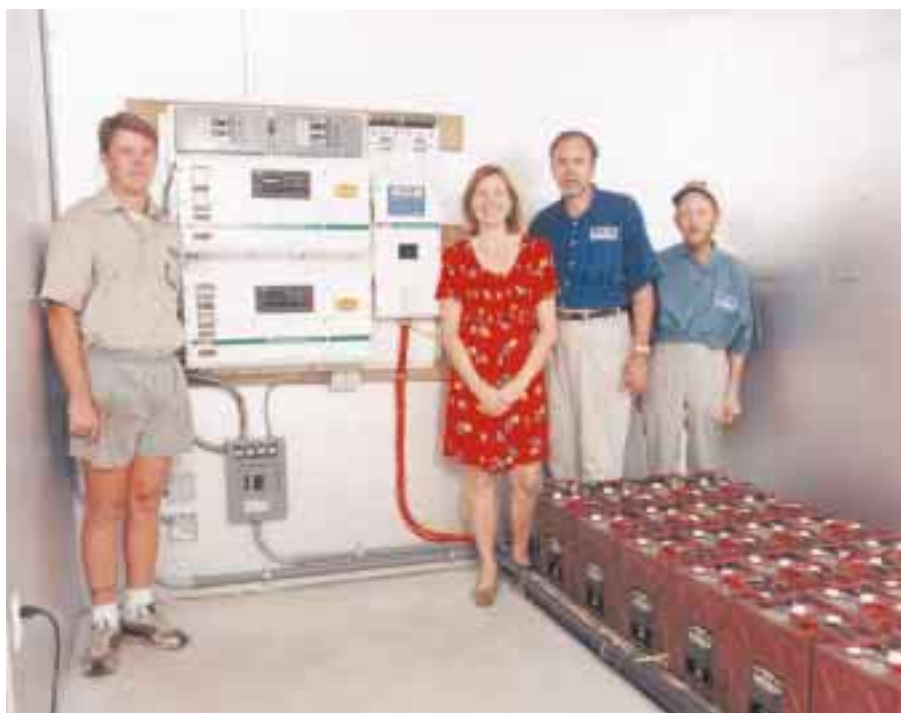
Below: ECS crew members (from left) Jamie Dempsey, Shirley Lane, Tom Lane, and John Ault in the custom built power shed which houses the Trace Power Panel and thirty-two Trojan L-16 HCs.
