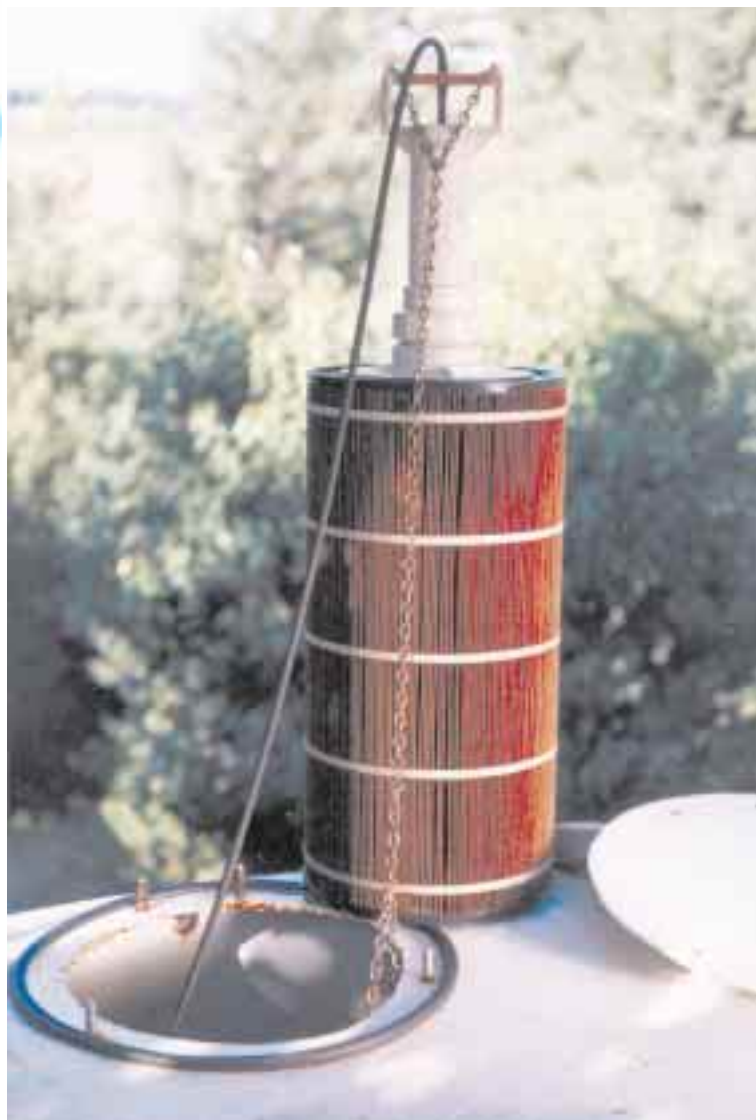
Above: The author's ozone filter just pulled from the tank for cleaning. The filter is white when clean.
