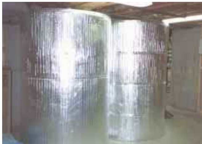
Below: Two 500 gallon insulated storage tanks.
