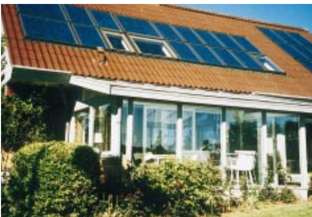
Even skylights aren't an obstacle as demonstrated in this roof-integrated system using Solarex laminates.
