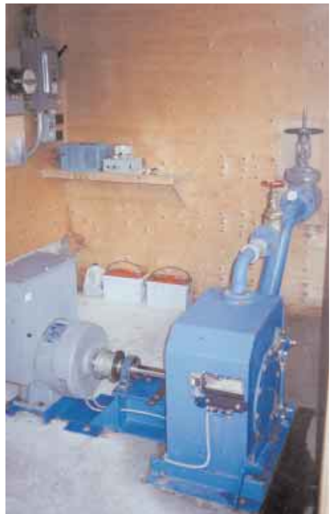
The 14 KW Lima generator is direct coupled to the Dependable Turbines Pelton runner.
