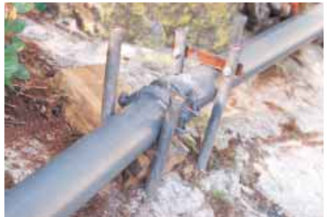
Pipe anchors were drilled into solid rock.
