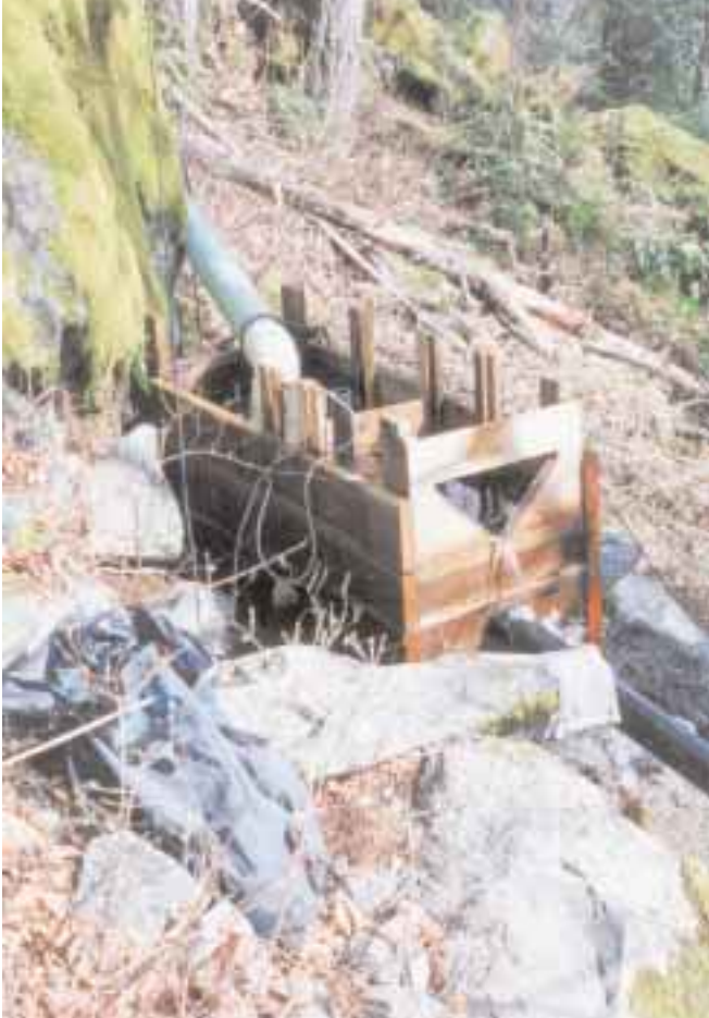
The intake box is used for filtering and settling of debris. The V-notch was used for determining flow during system planning.
