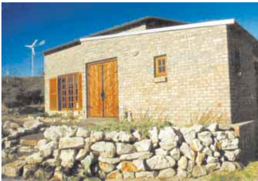
The passive solar home and offices at Redhill Mountain Reserve.
