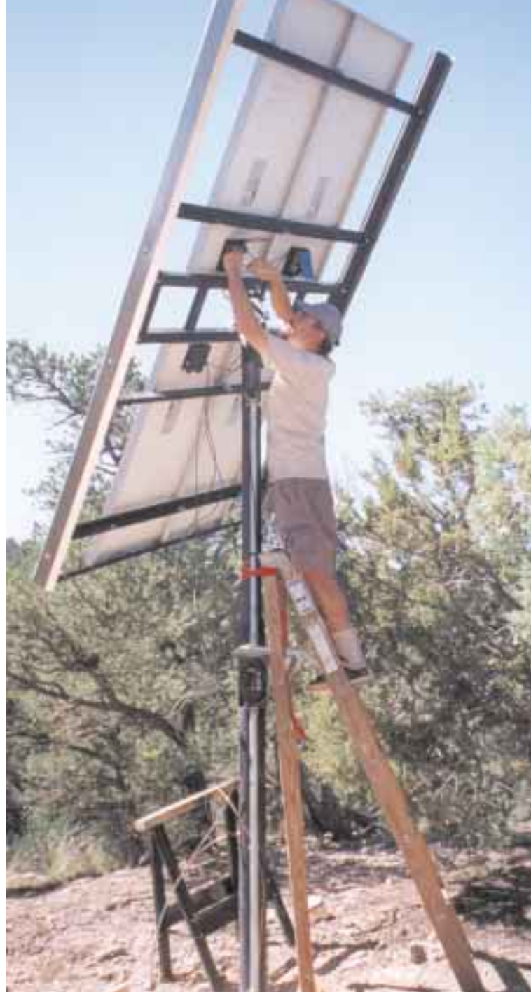
Windy does the final wiring of the PV array.
