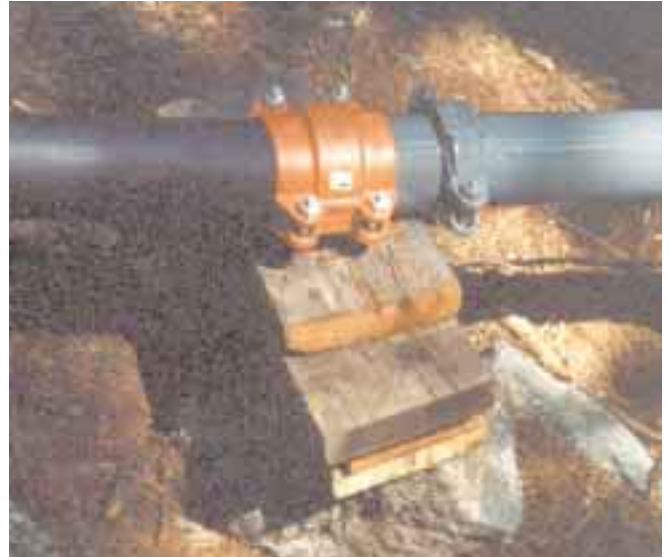
A hugger clamp joins poly pipe to steel pipe.
