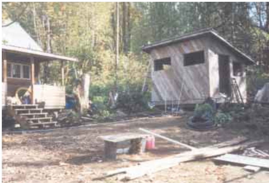
Floyd and Frasia's cabin (left) and power shed (right).
