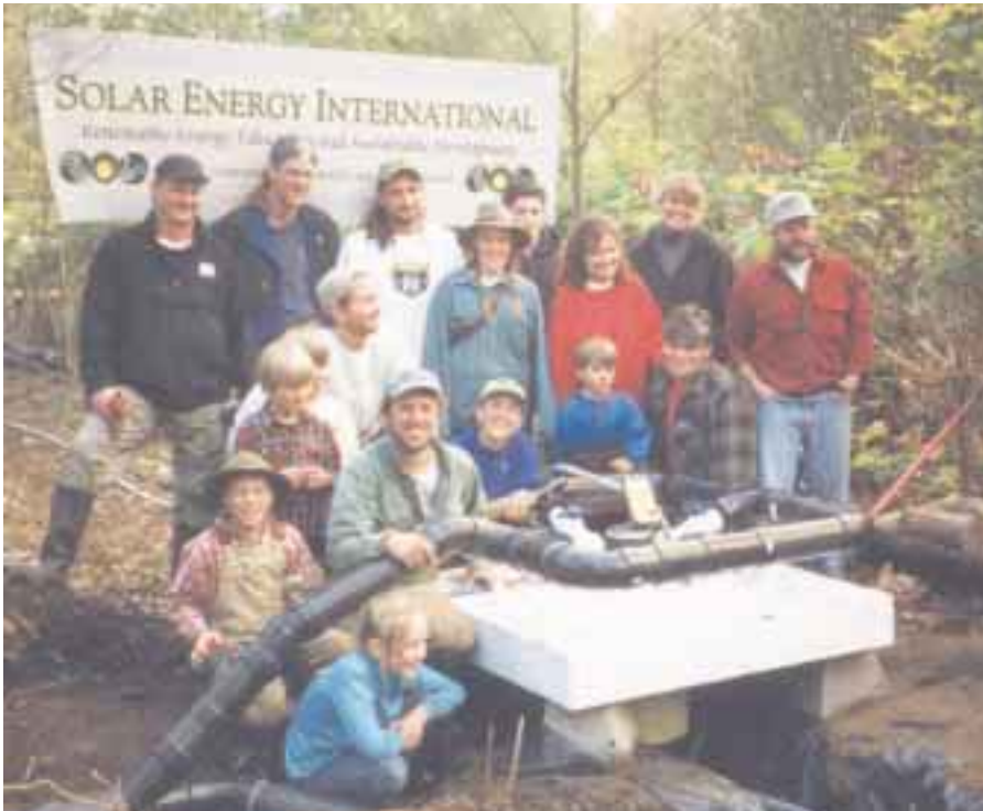
After two long days of work, remaining SEI students, staff, family, and friends gather for a group photo with the running turbine.
