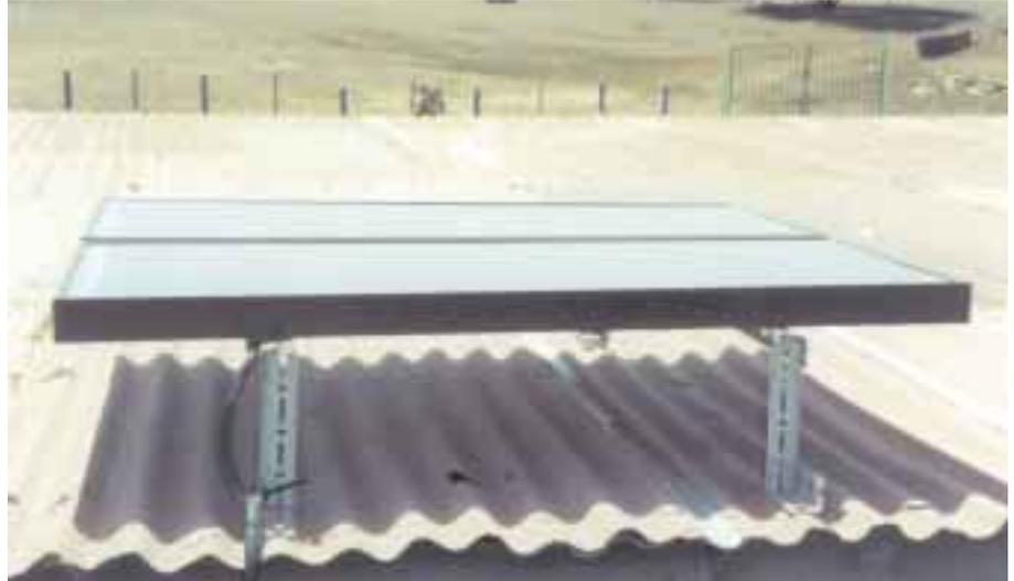
**Because of Bonaire's tropical latitude, the Solarex MSX-60 PVs are mounted at a 15° angle from horizontal.**
