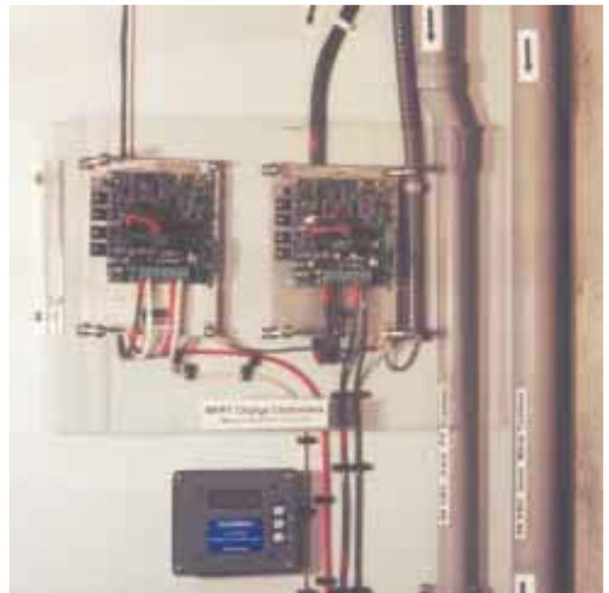
A pair of C-40s (acting as diversion controllers) regulates the battery bank voltage. They dump excess power into a pair of home-built, heavy-duty, resistive hot-air heaters. The C-40s are connected to the battery bank via a 110 amp class-T fuse with parallel #2 (33 mm<sup>2</sup>) cable from the fuse to the dump load.
