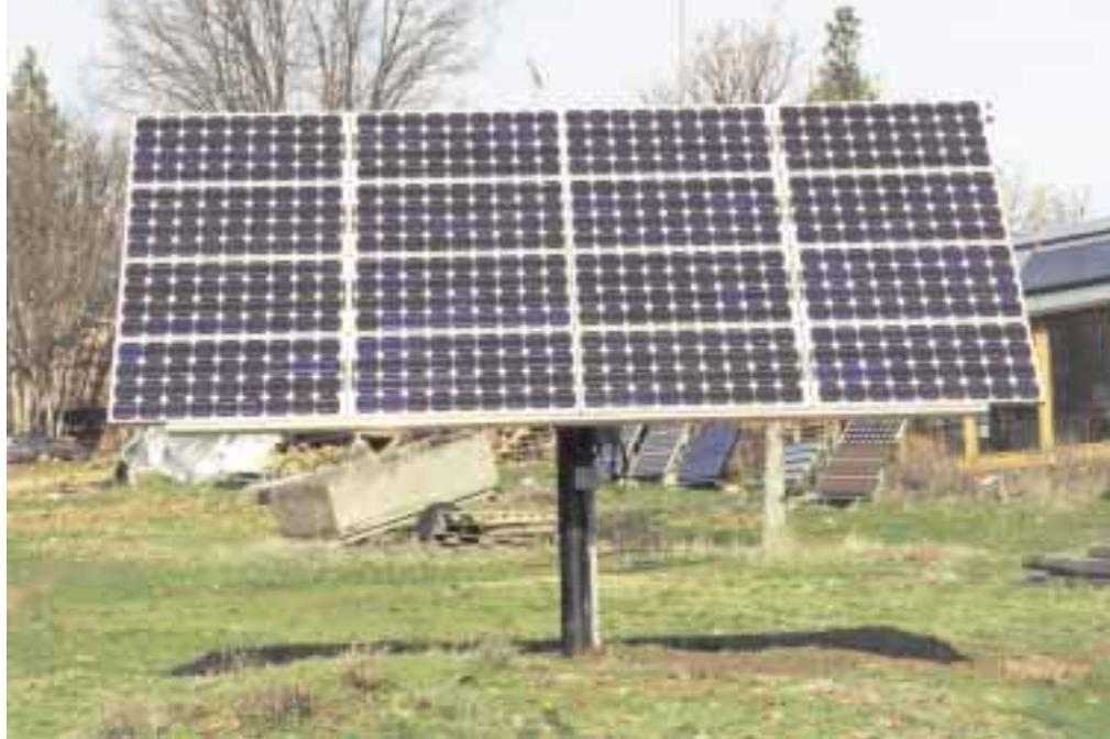
**Sub-array #1: Sixteen BP-590 PV panels on a dual-axis Wattsun tracker provide 1,140 rated watts at 24 VDC.**
