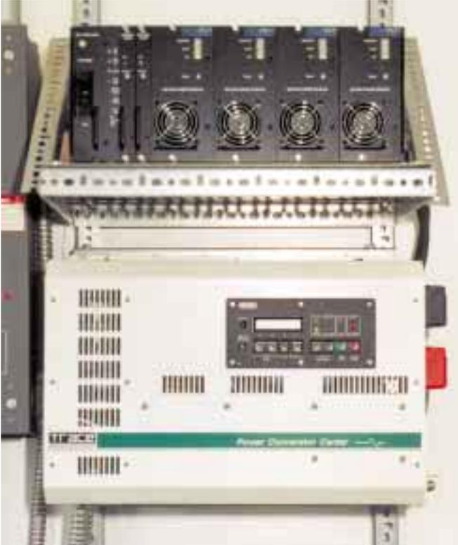
**Inverters: An Exeltech MX 4 KW (top) and a Trace SW4024 4 KW (bottom).**
