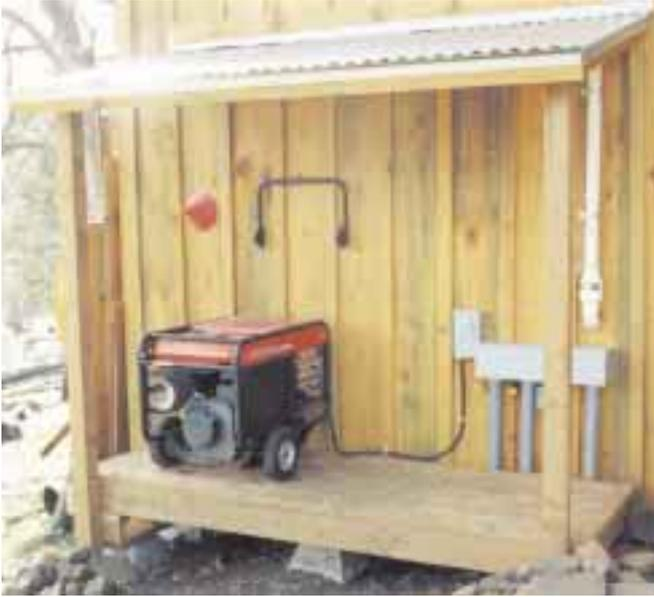
**On the north side of the power room, the Honda generator provides 6,500 watts of backup power.**
