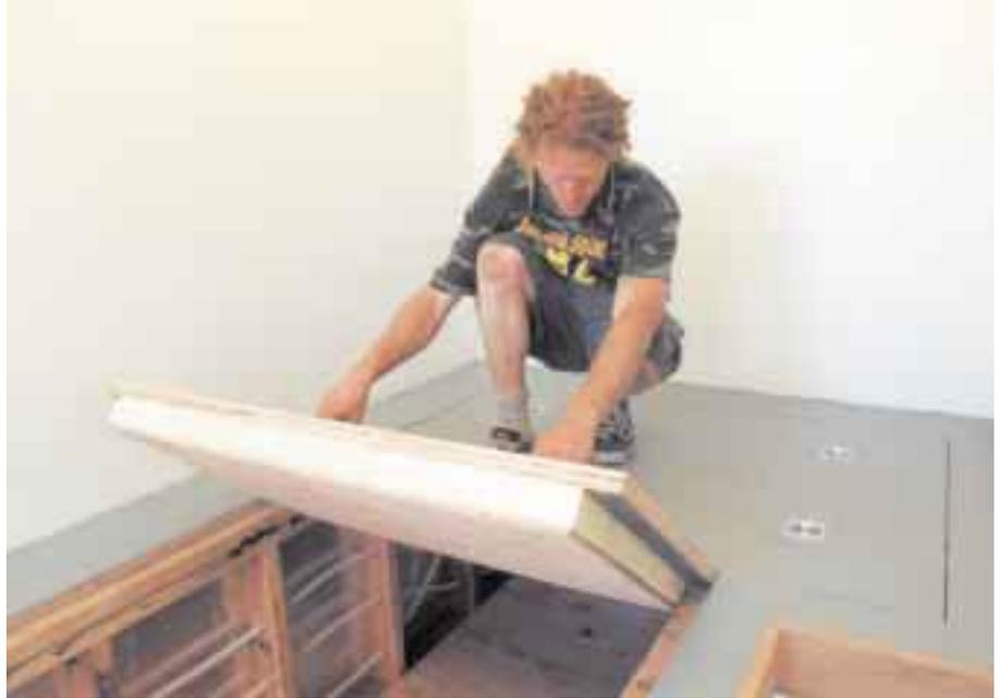
**Insulated battery box lids lift out for battery watering and maintenance access. Replaced, they act as a floor for access to power components on the walls.**
