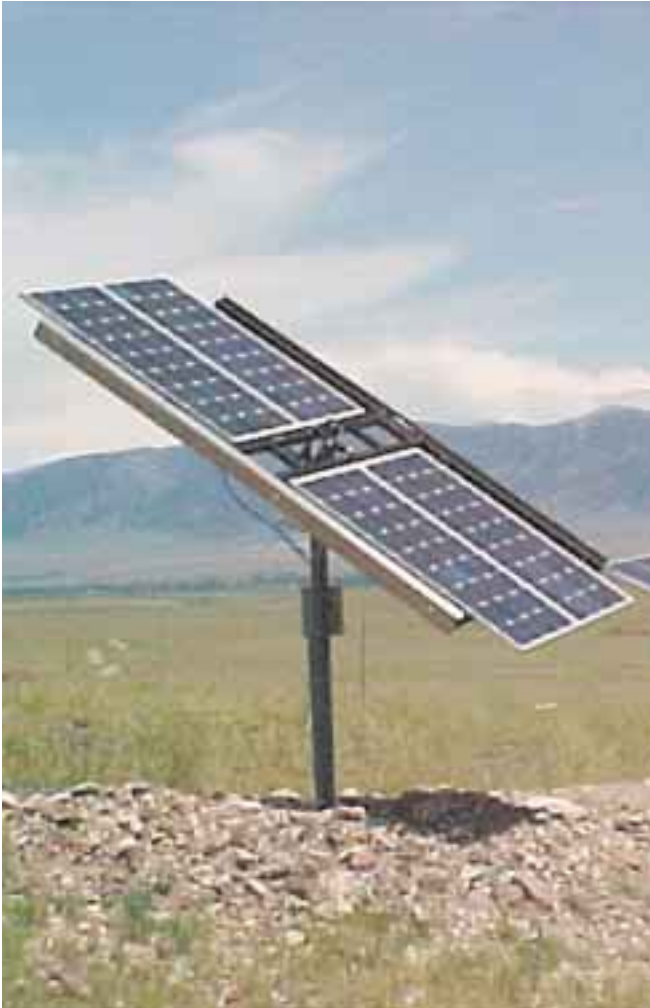
Four AstroPower 110 watt PV modules on a Zomeworks tracker contribute to the main 24 volt system.
