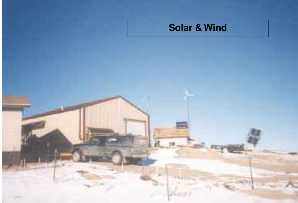
The shop and power shed with PV arrays and wind generators visible.
