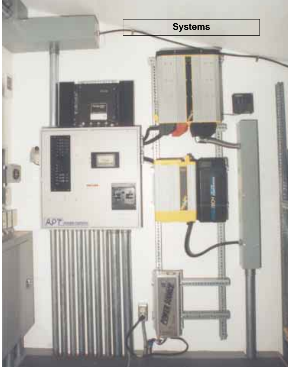
The 12 volt system including power center, inverters, controller, and charger.
