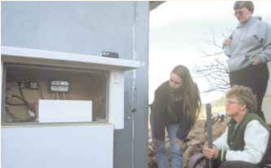
Darlene's exterior-mounted inverter enclosure keeps the hum outside.
