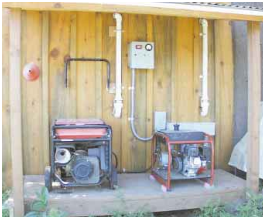
Fossil-fuel backup: A Honda ES6500, 6,500 watts at 230 VAC (left), and a Feather River Solar GennyDeeCee, 1,200 watts at 12 VDC (right).
