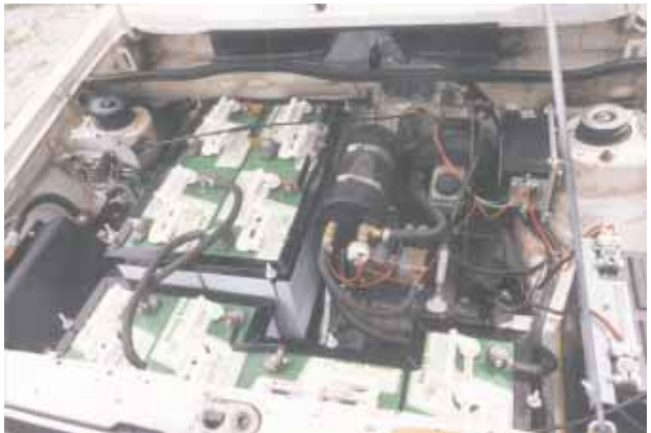
A split-level battery pack makes the most of the available space.
