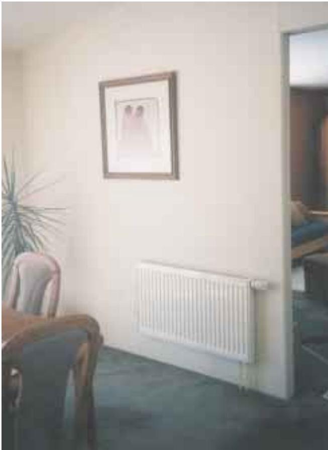
An individual thermostat controls each Buderus radiator.
